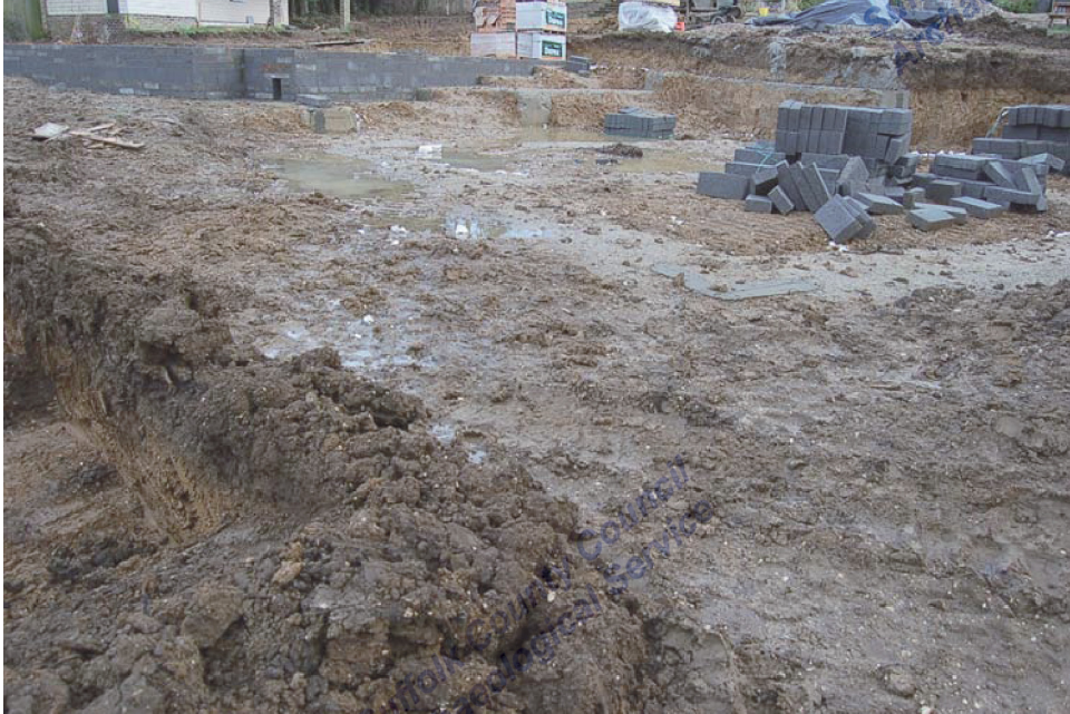
Figure 4. General site shot, facing north showing depth of truncation
