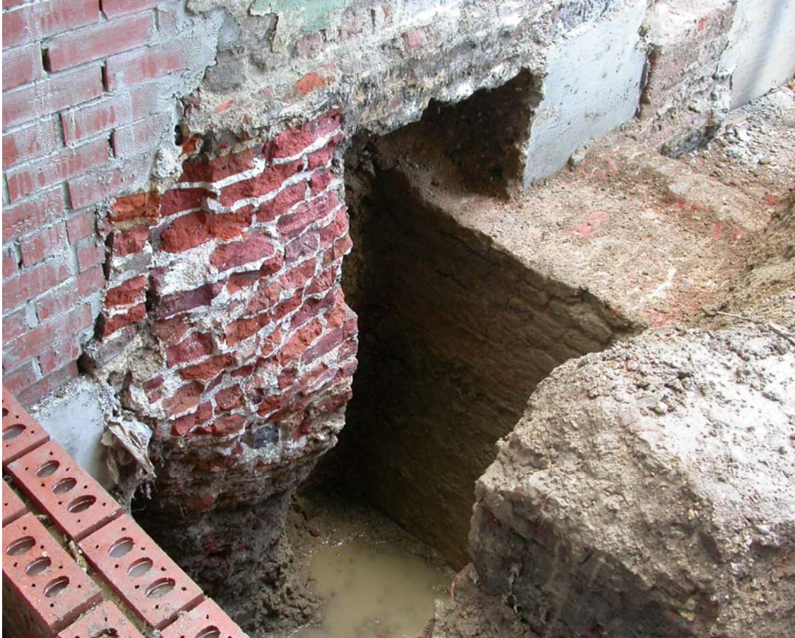
Figure 12. Underpinning 0031 (left) and foundation/cellar wall 0029 (right)
