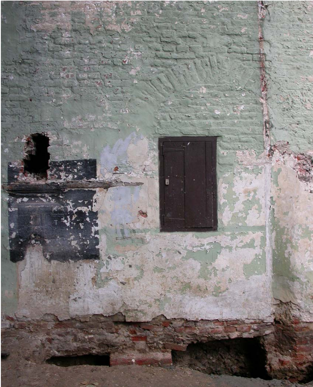
Figure 13. The top of brick plinth 0028 (lower centre) beneath a blocked arch
