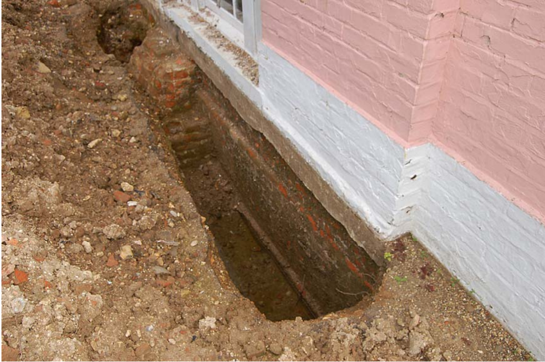
Figure 7. View of foundation 0039 and buttress 0019, looking east
