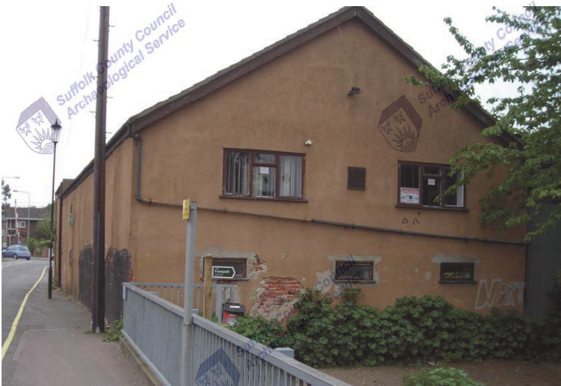
Plate 1. Trench 1 building prior to demolition; once owned by J. Prentice and Co?
