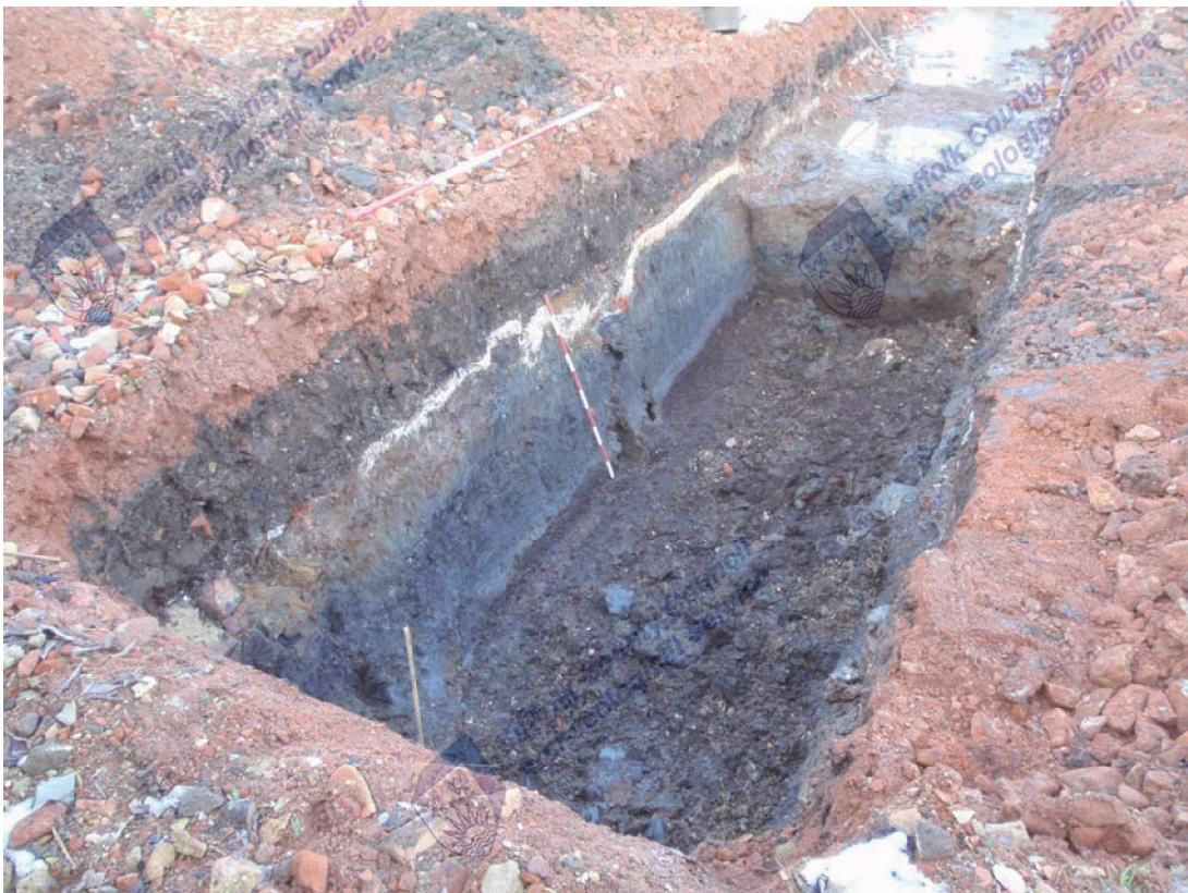
Plate 3. Trench 1 looking north-east
