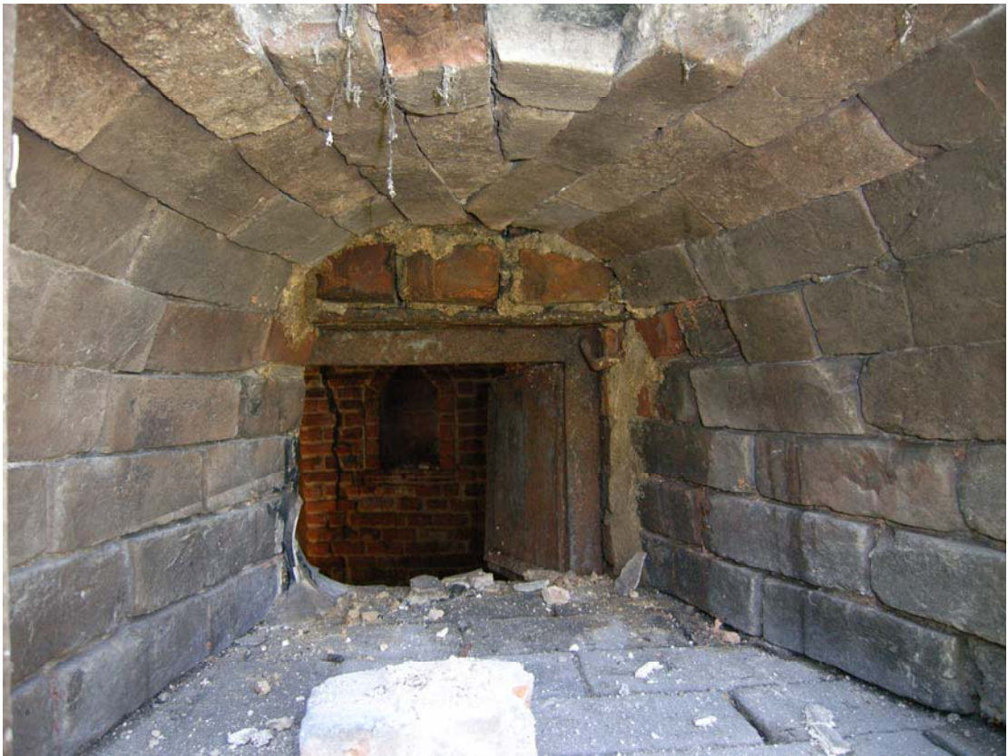
A2.8 Interior of brick oven between posts I and J
