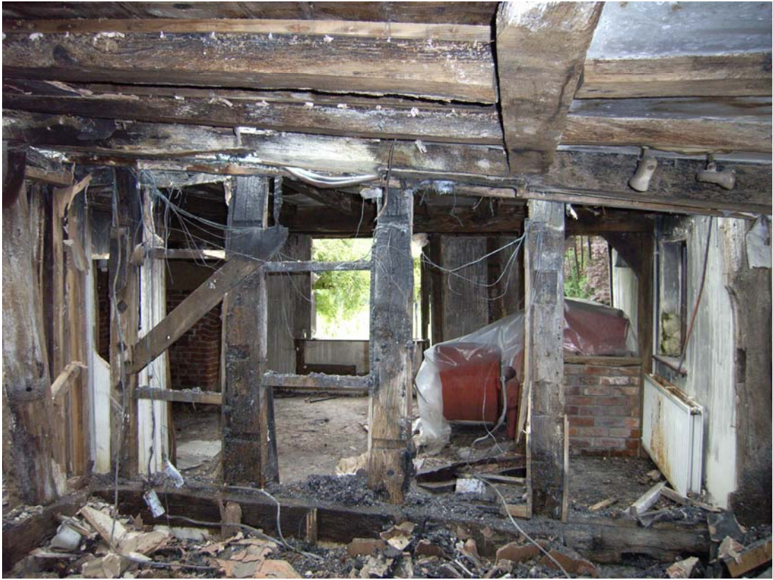
A2.9 Elevation J-G from west showing infill trenches and a window sill or lintel re-used as a stud to left (with original brace attached). Former door and stair trap to right.
