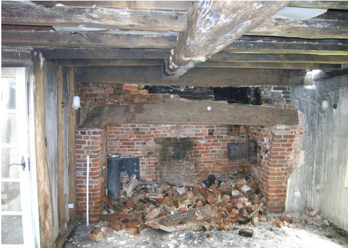
A2.3 Internal view of truss J-I from south, showing partly collapsed fireplace and largely original 17 th century ceiling in room G-J-H-I.
