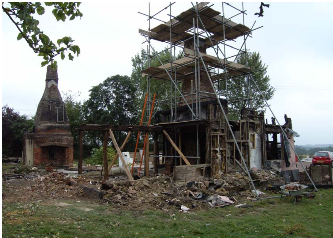
A2.12 General view of site from south-east showing demolition nearing completion (chimneys to remain in situ ).
