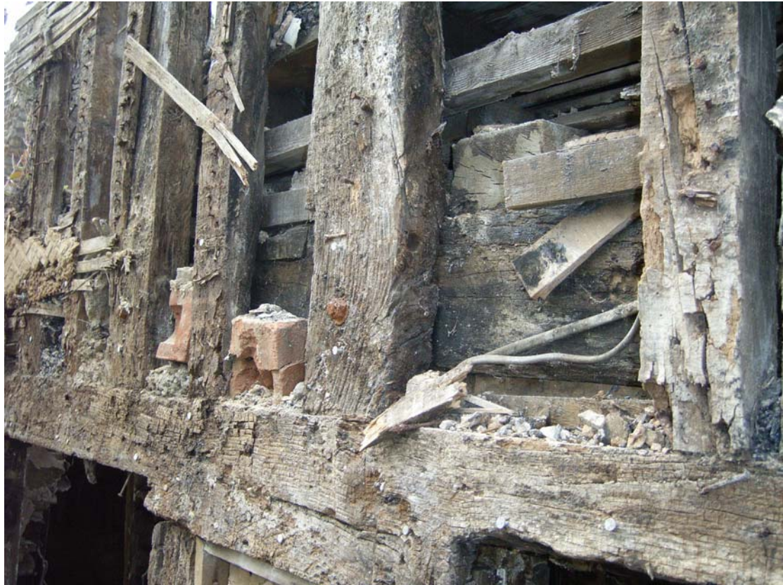
A2.11 Detail of external elevation A-E from south-east showing externally weathered studs with notches for infill staves (in contrast to infill of structure G-M-H-N).
