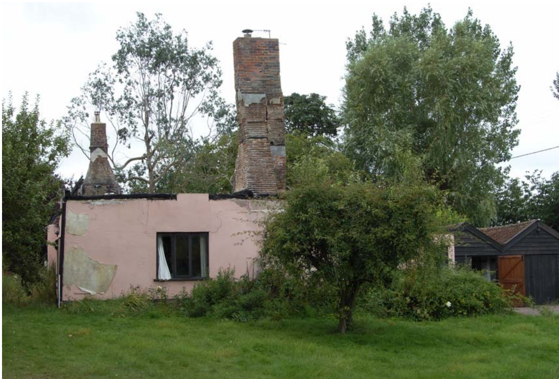
A2.1 External elevation H-N from east prior to demolition
