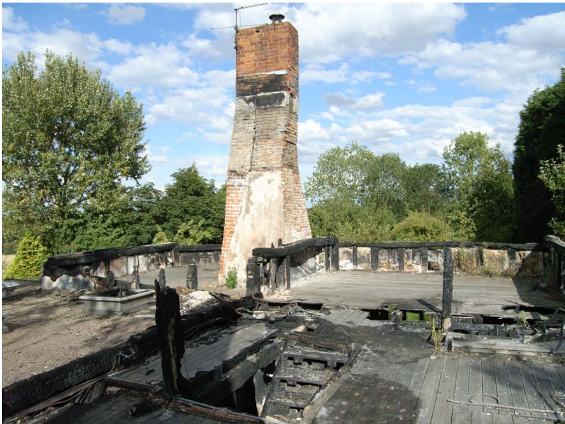
A2.4 Upper storey of structure G-H-M-N from west showing 17 th century chimney to right with secondary chimney to left.
