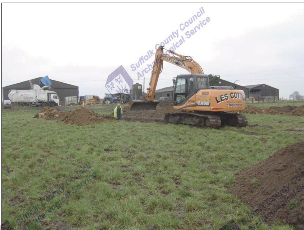
View of evaluation in progress
