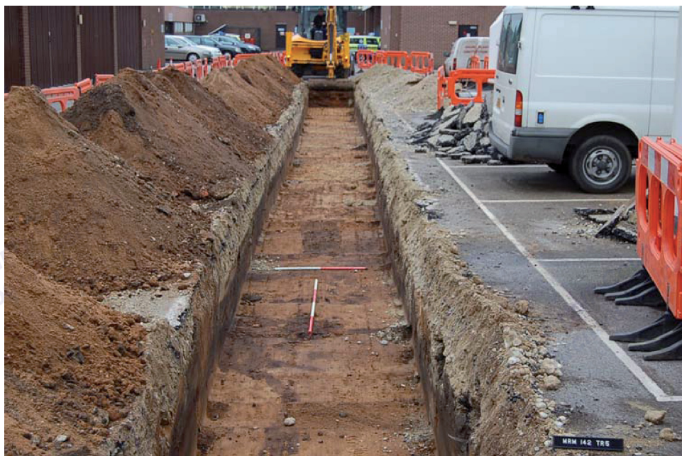
Plate 2. Trench 5, facing southeast
