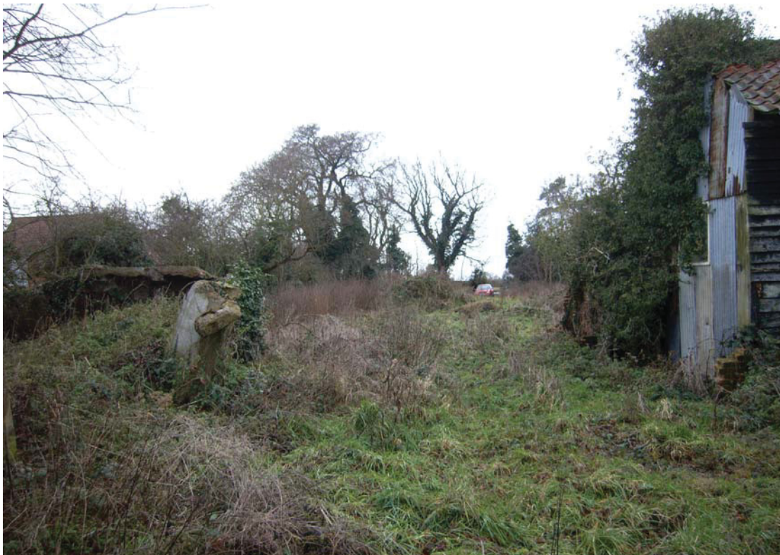
A2.2 General view of site from east showing site of demolished maltings in centre with southern gable of barn to right and remains of WWII gun emplacement to left
