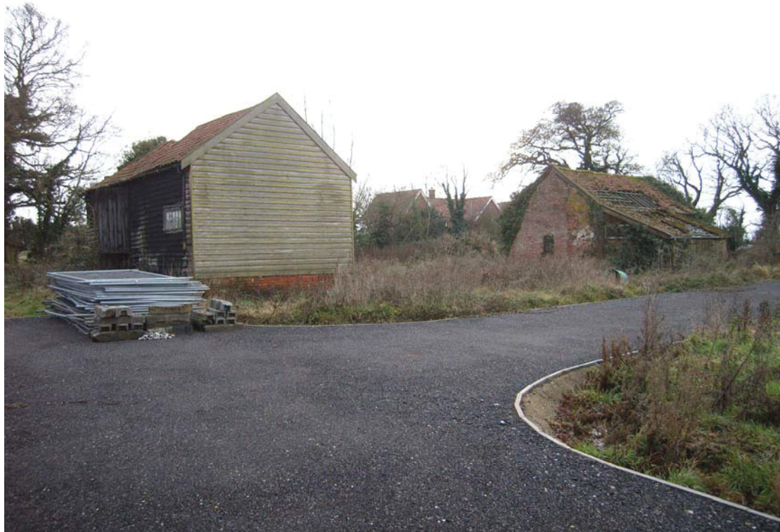
A2.3 General view of site from north showing barn (2) to left, stable (1) to right & modern housing estate in rear
