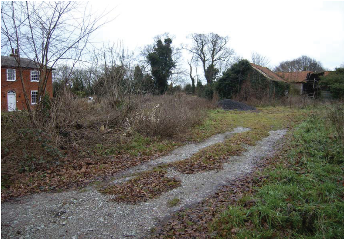
A2.1 General view of site from Trimley Road entrance to west, showing house (3) to left with stable (1) & barn (2) in centre and site of demolished maltings (4) to right
