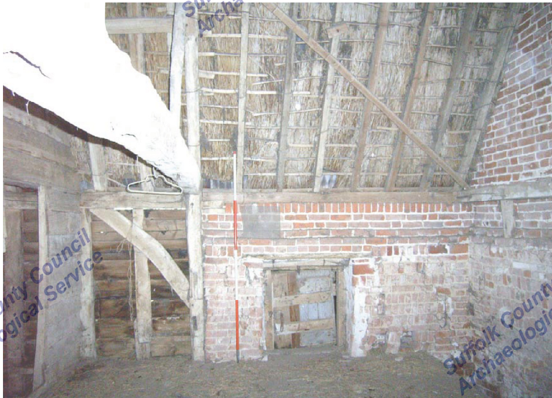
A2.6 Southern internal elevation of hay loft above 19 th century stable (2) showing loading door & corner of 17 th century barn & stable to left
