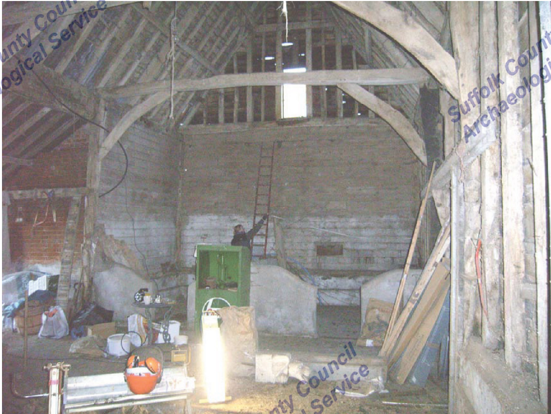
A2.9 General view of barn interior from west showing original arch-braces to tie-beams with internally boarded eastern gable in rear
