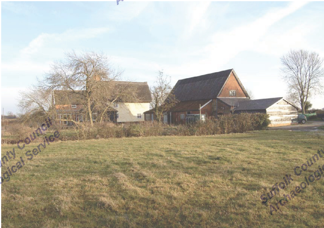
A2.2 General view of site from Horse Meadow to west showing house to left and barn right
