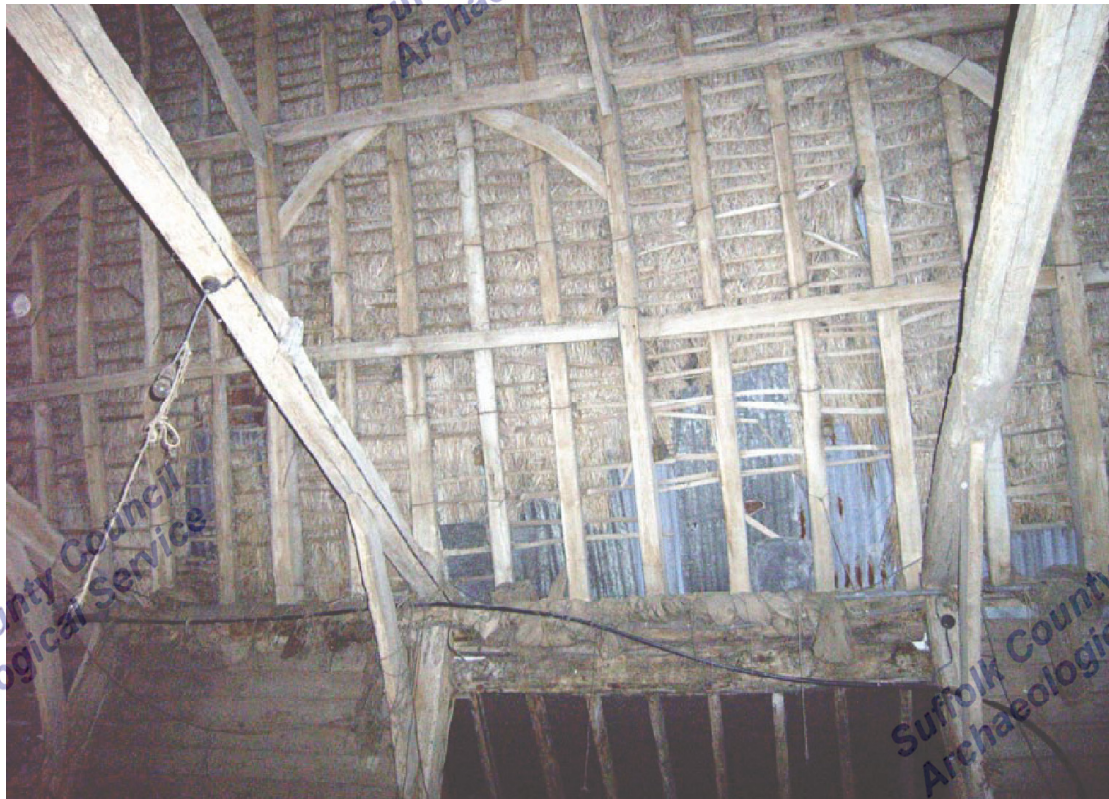
A2.8 Intact roof structure and arch-braced open trusses tie-beams flanking central northern bay of barn
