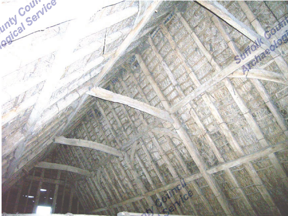
A2.7 Original roof structure of barn from west showing intact wind braces with upper tier of clapsed-purlins and lower tier of butt-purlins
