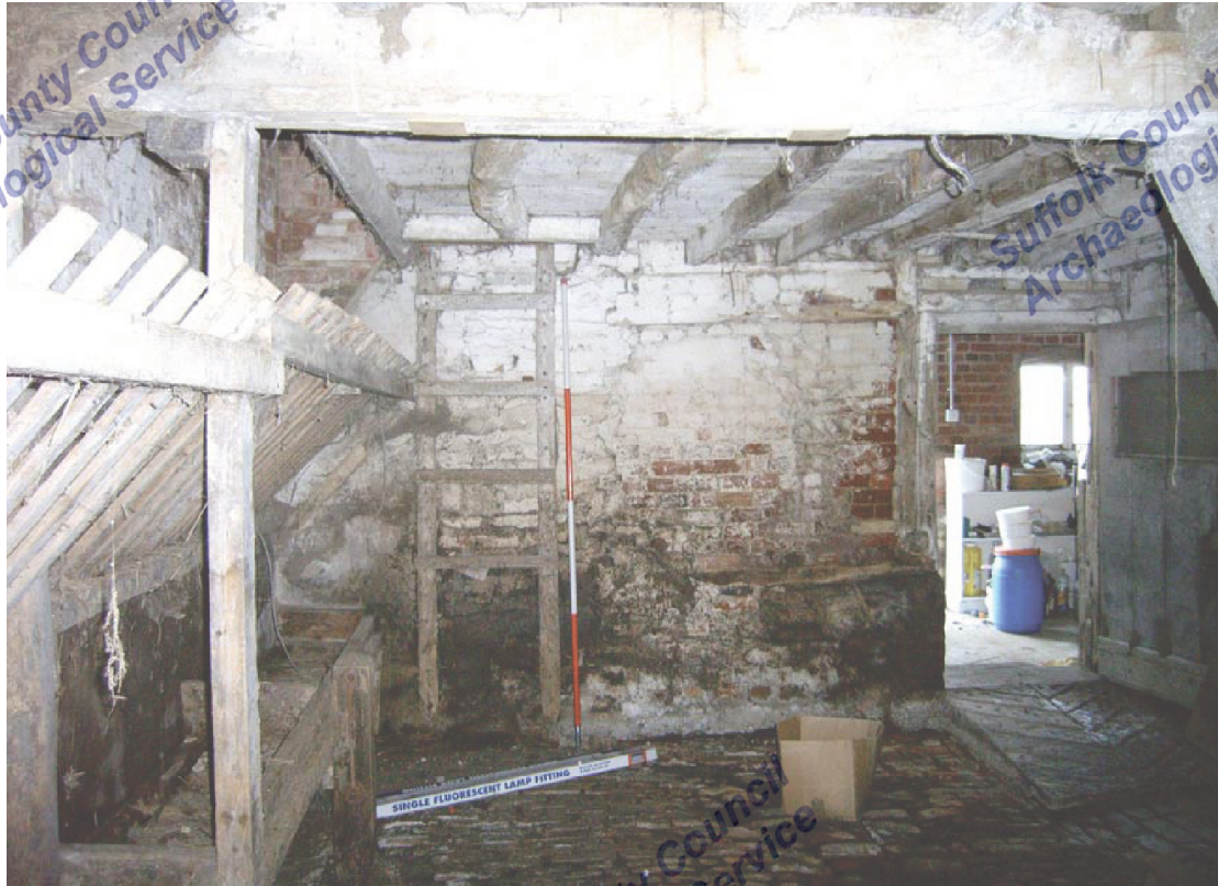
A2.5 Internal northern elevation of 19 th century stable (2) showing hay rack and manger against western gable to left (lowered for cattle), loft ladder and entrance to right. The entrance is in the same position as that of the 17 th century stable
