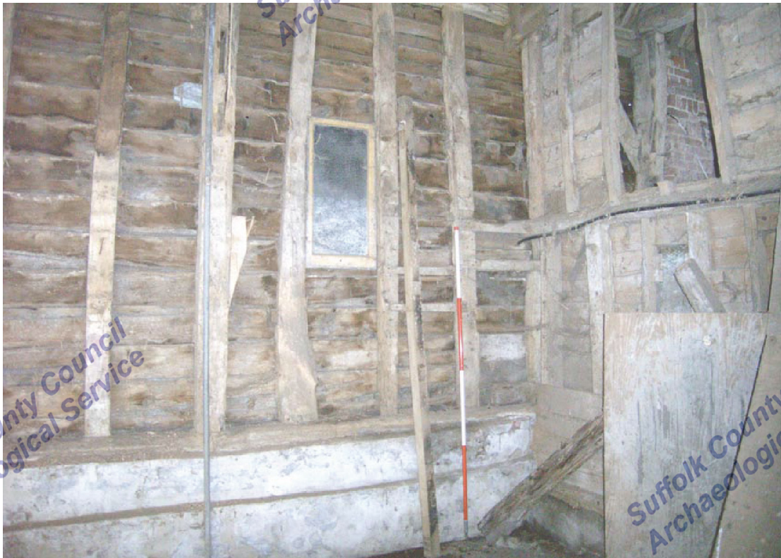
A2.10 Southern elevation of original stable bay, now within barn, showing mortise of removed partition rail in storey post to left with arch-brace mortise above
