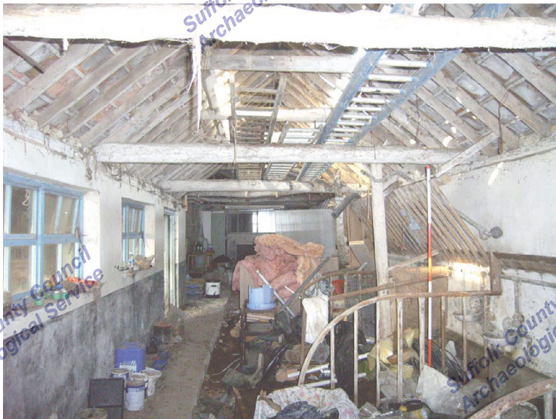
A2.4 Interior of brick shed to east of yard (7) south showing former open arcade to left and 20th century cattle stalls, hay rack and trough to right
