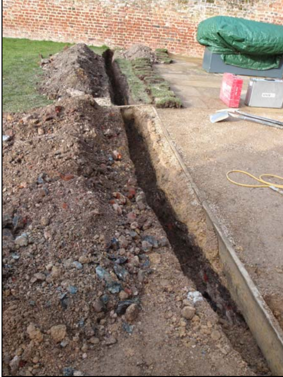
Plate I: General view of northern half of trench, looking north
