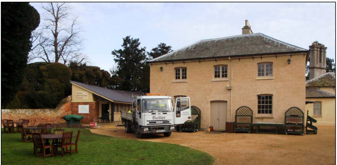
Plate V: general view of the west end of the Service Wing, looking northeast
