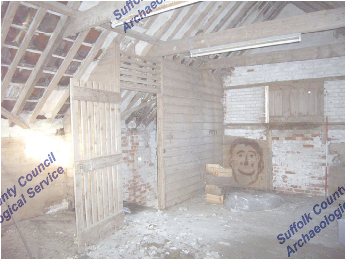
A2.4 Upper granary storey from south-west showing enclosed stair with slatted door and evidence of grain bins with axial passage against eastern gable to right
