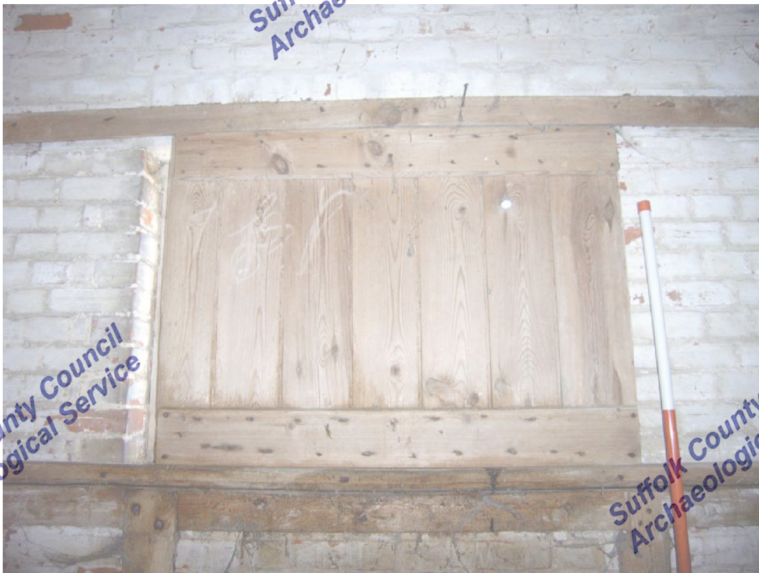
A2.6 Detail of deal sliding window shutter to internal eastern gable of upper storey
