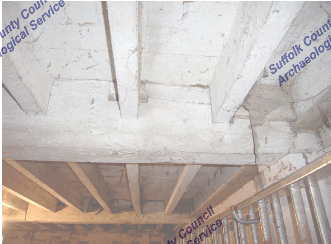
A2.7 Detail of ground-floor ceiling from west showing empty mortises in re-used 17th century binding joists
