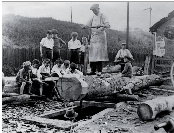
Plate I: a sawpit in use in the early 20 th century (source: Weald and Downland Museum website )
