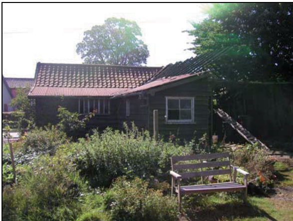
Plate III: View of former outbuilding, looking S
