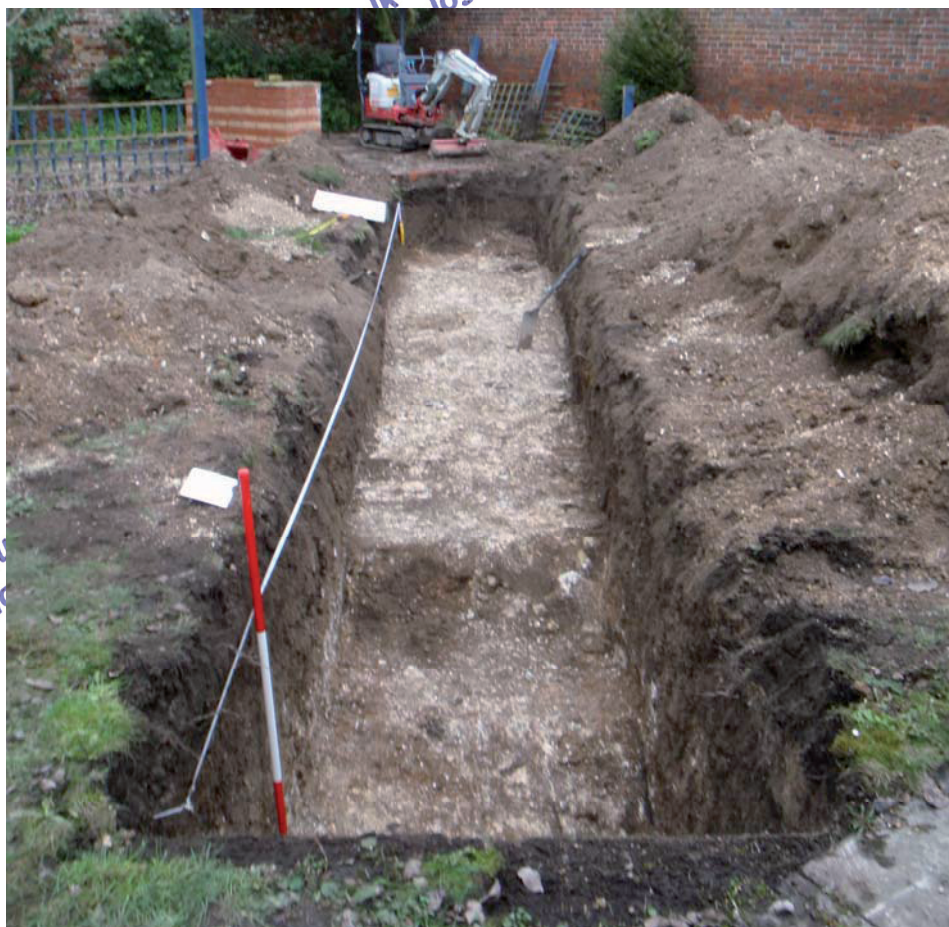
Figure 4. Evaluation trench looking north
