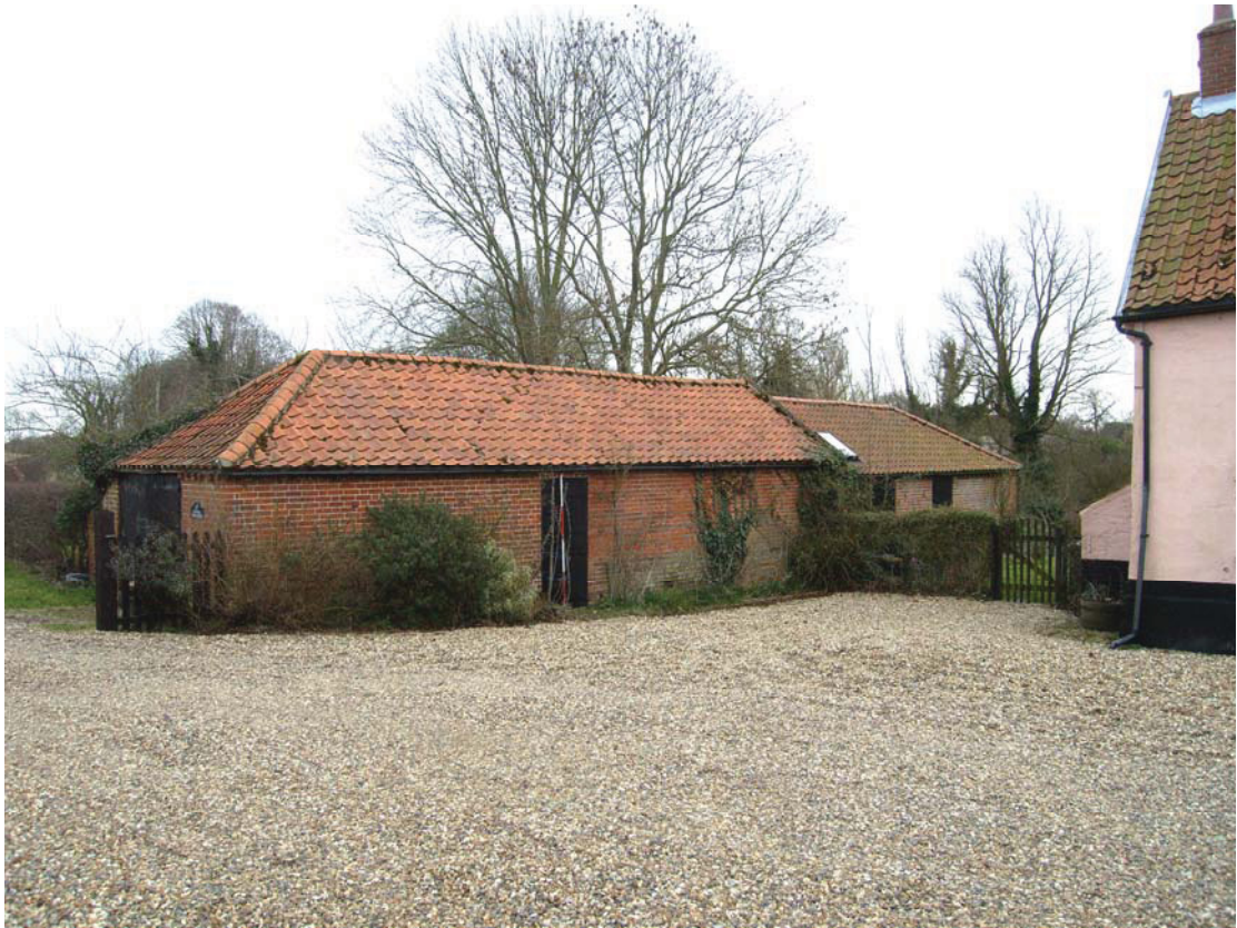
A2.3 Exterior from west showing corner of house to right
