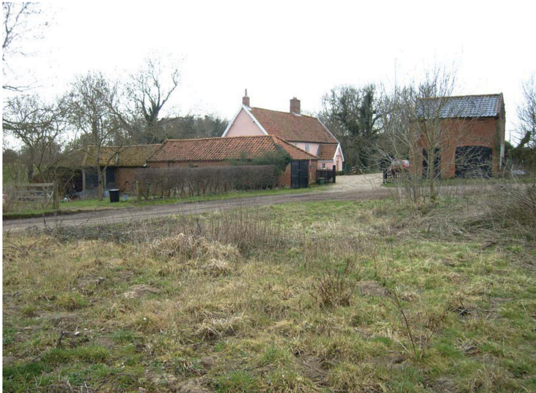
A2.1 General view of site from north-east showing range of brick sheds (1) to left, 16 th century house (2) in centre to rear & contemporary stable (3) to right.
