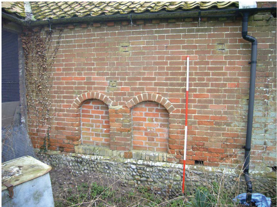
A2.6 External eastern elevation of shed B showing blocked arches
