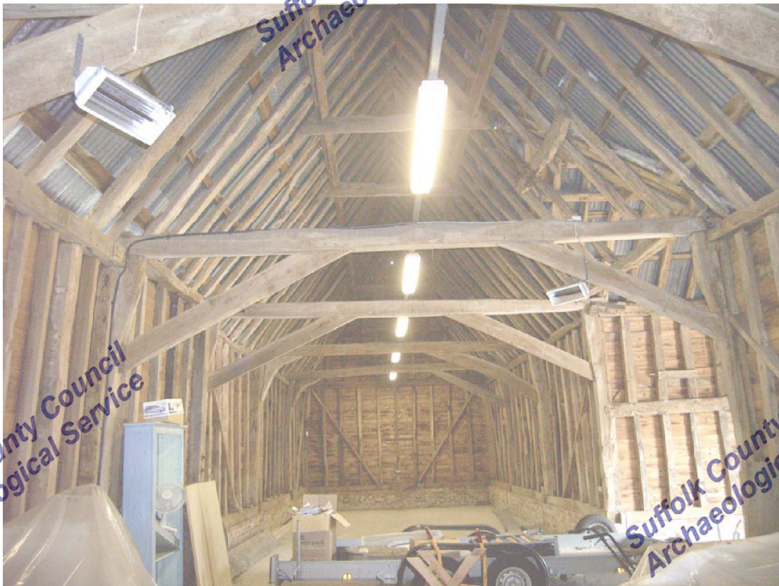
A2.4 General view of interior from south showing secondary clapsed-purlin roof with intact arch-braces to tie-beams and porch in bay C to right
