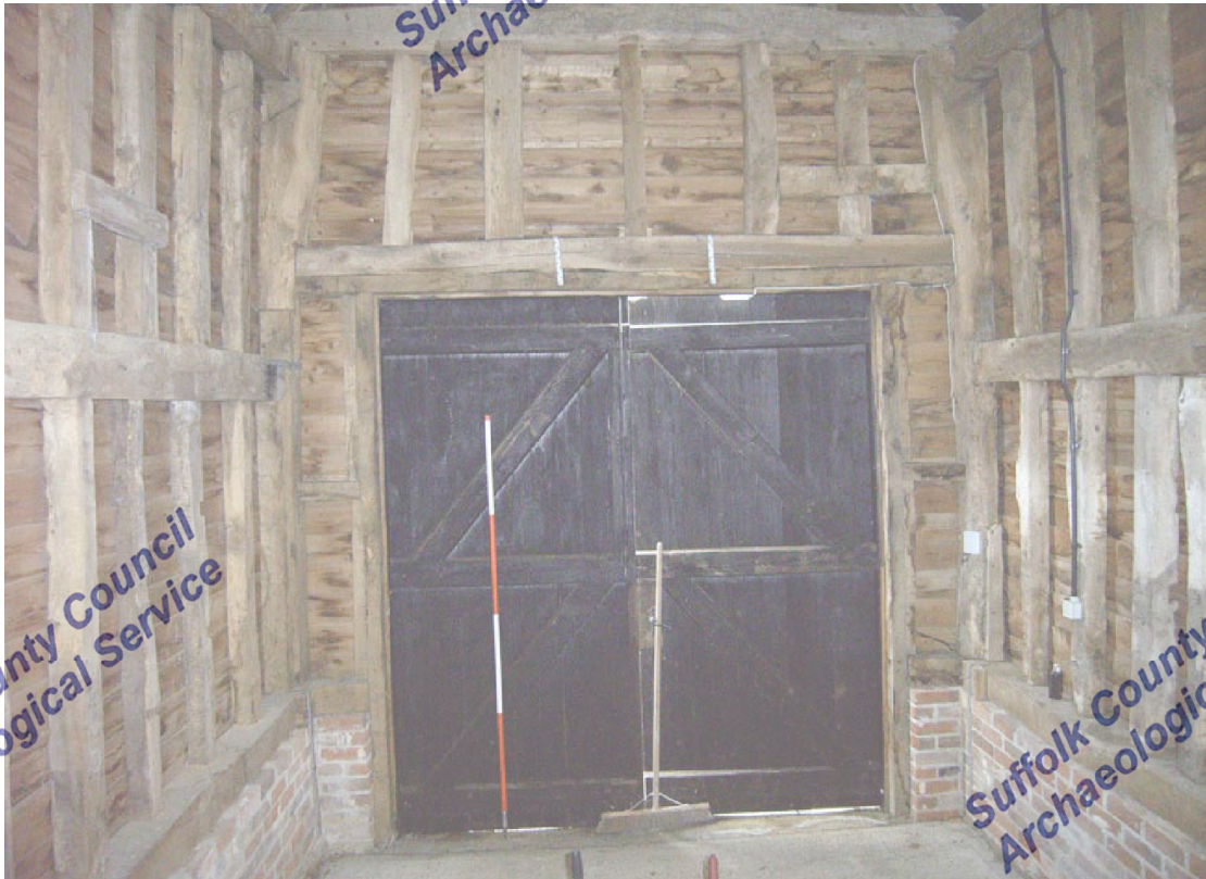
A2.6 Internal eastern elevation of porch (G) showing mid-rails in side elevations and mortises of original door jambs in tie-beam
