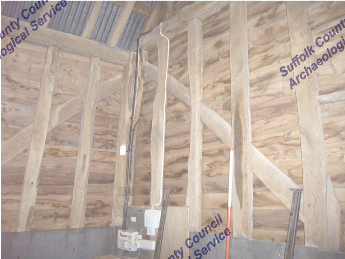
A2.5 South-eastern internal corner showing southern gable to right with original externally tenoned wall braces
