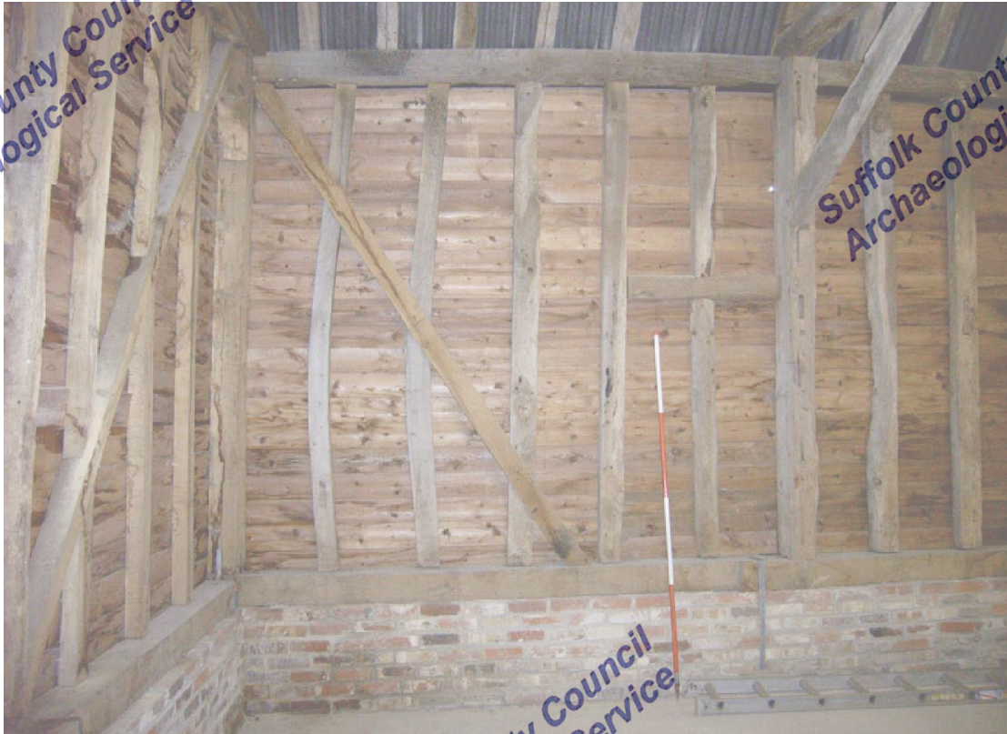
A2.7 Eastern internal elevation of northern bay (F) showing apparently secondary door lintel and secondary arch-brace replacing closed partition to right. External bracing removed. Rebuilt northern gable to left
