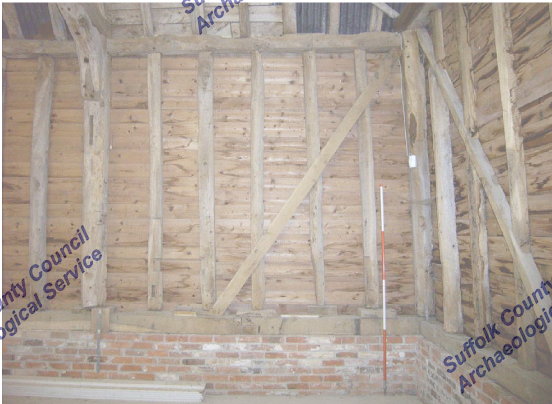
A2.8 Internal western elevation of northern bay (F) showing original studs (external wall braces removed) and plinth rebuilt
