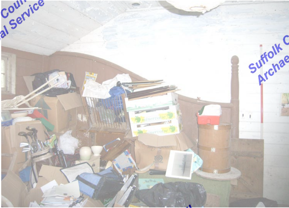
A2.7 Internal eastern elevation of stable (A) showing curved wainscot with turned finial and northern elevation to left
