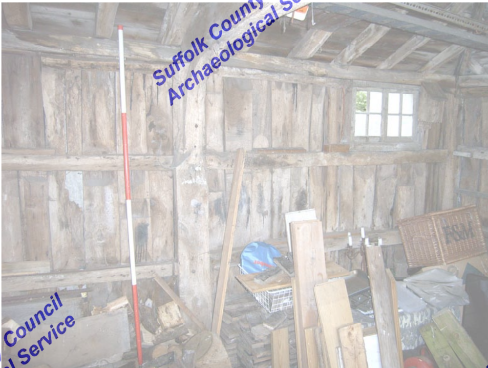
A2.8 Detail of board-and-rail construction of northern internal elevation of open shed (C) with bolted knee-brace to tie-beam. Eastern gable to right
