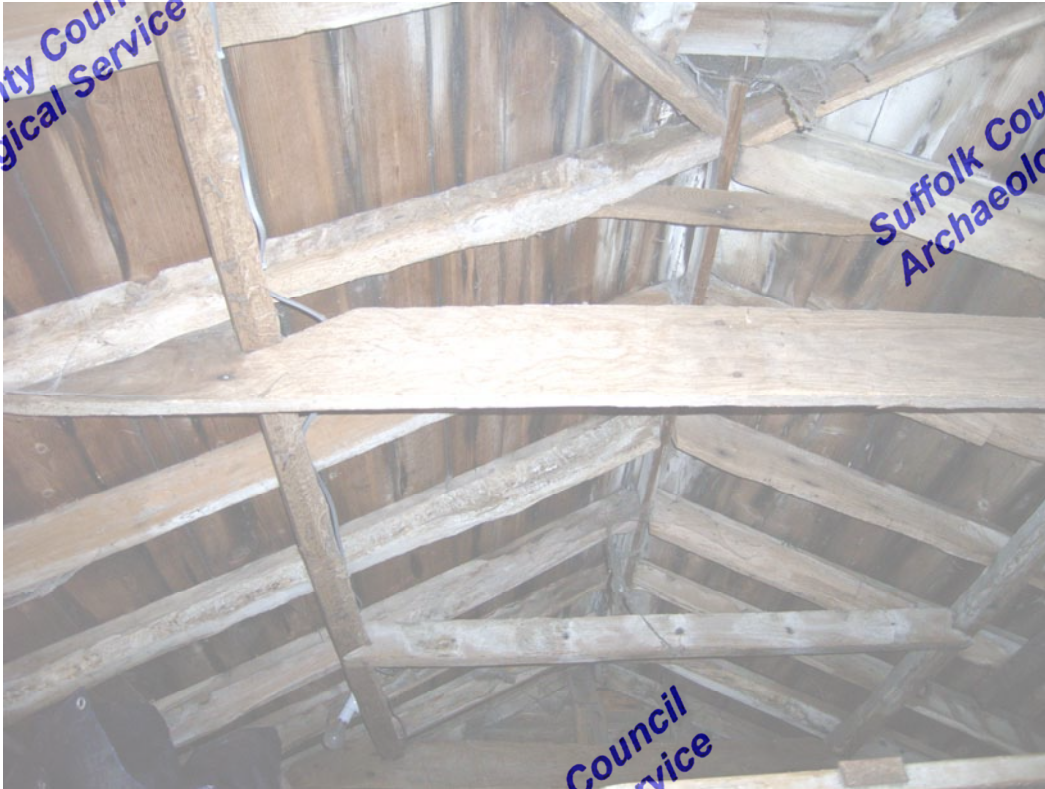
A2.9 Detail of original clasped-purlin roof structure with nailed collars seen from east in open shed
