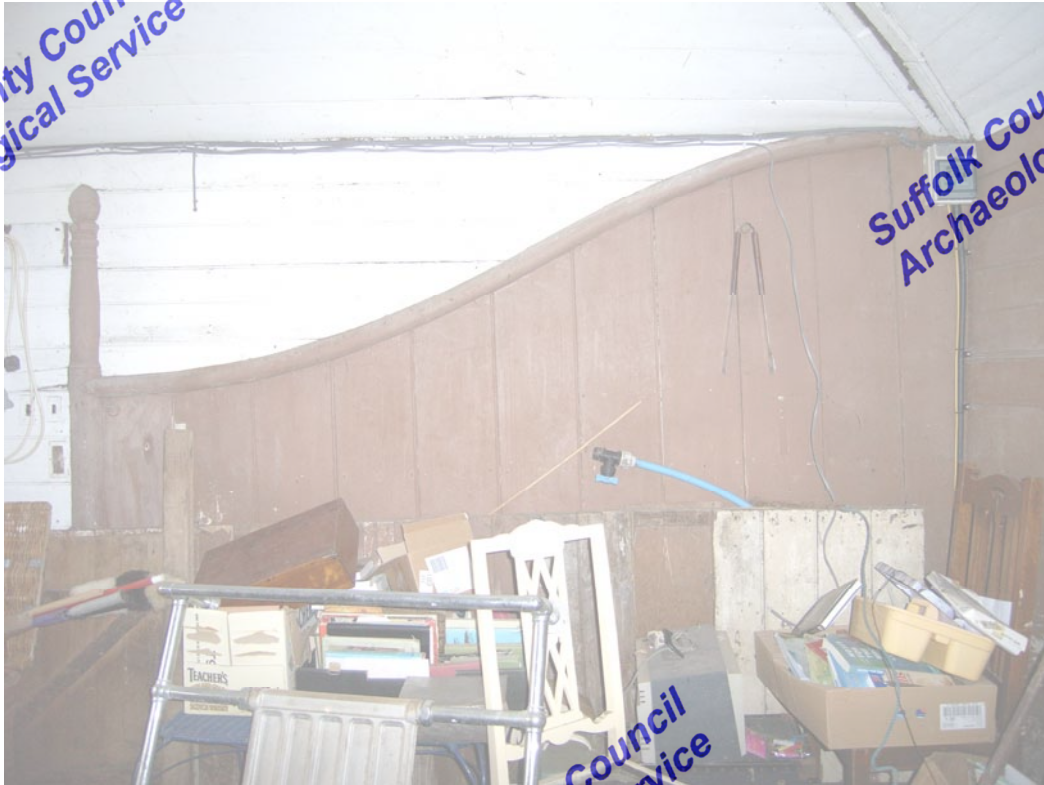
A2.5 Detail of curved stall wainscot to internal western elevation of stable (A)
