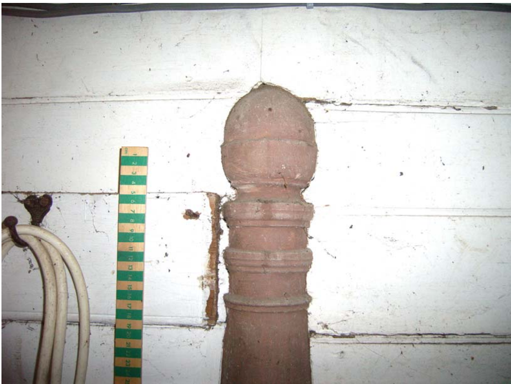
A2.6 Detail of turned stall finial against internal western gable
