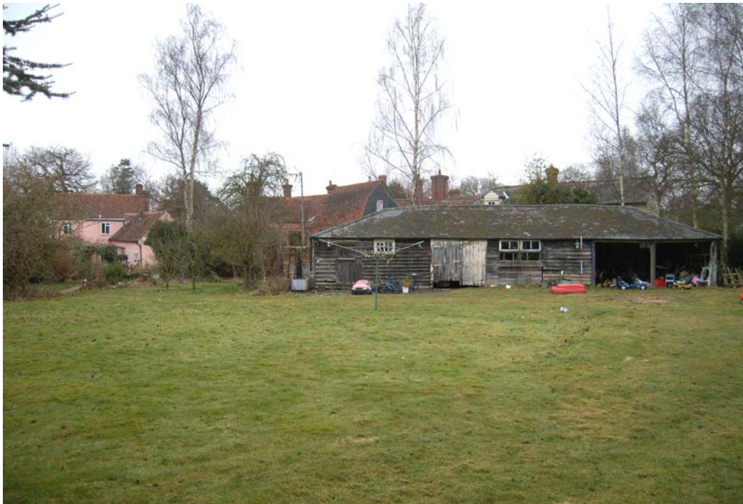
A2.1 General view of site from south showing Wren Cottage with its single-storied rear wing to the left and the outbuilding to the right. Compare Constable's painting below.
