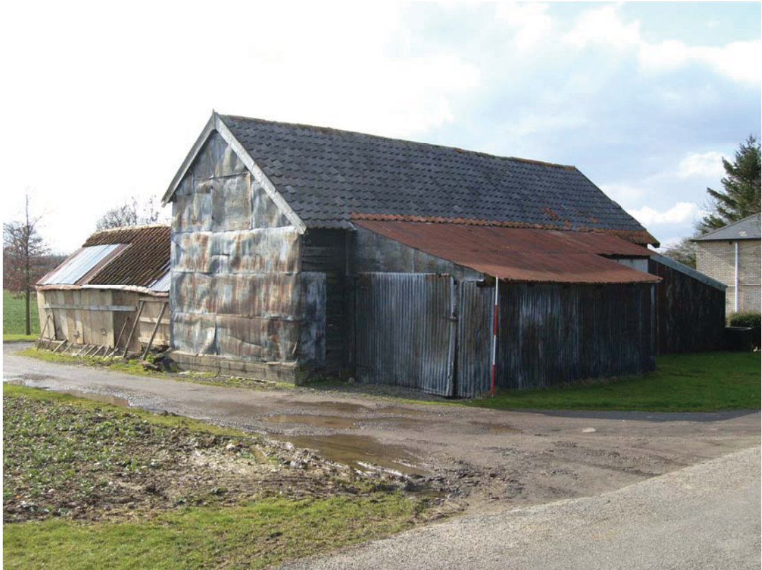
A2.3 Exterior of barn from north-east showing farmhouse in rear to right, showing 20 th century lean-to porch and sheds to right and 19 th century clay-lump shelter shed (C) to left
