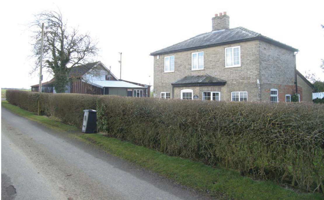
A2.2 General view from road to north-west showing Proctors Farmhouse to right and Proctors Barn to left
