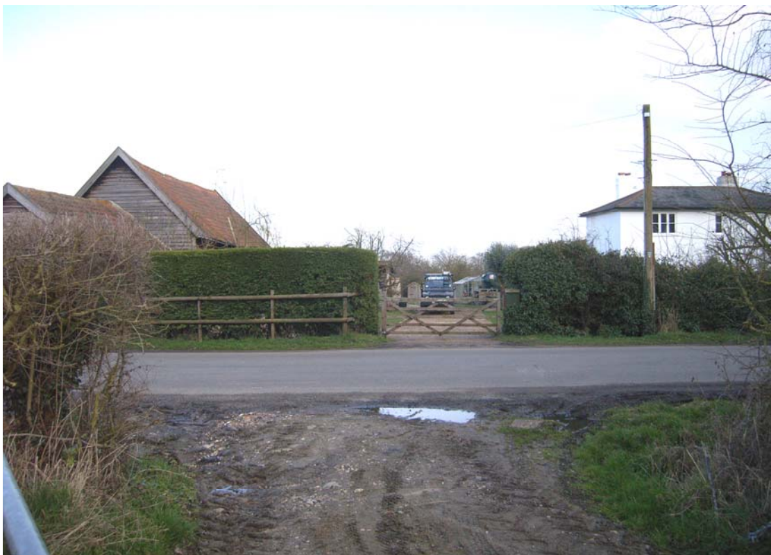
A2.2 General view of site from west showing proximity of farmhouse to right
