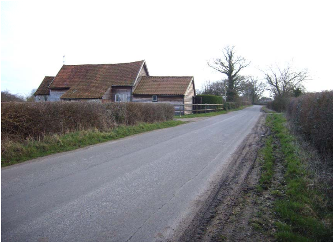
A2.1 General view of site from Potash Farm Road to north, showing barn (A/B) in centre with brick stable (C) to left and recently rebuilt shed (E) to right.
