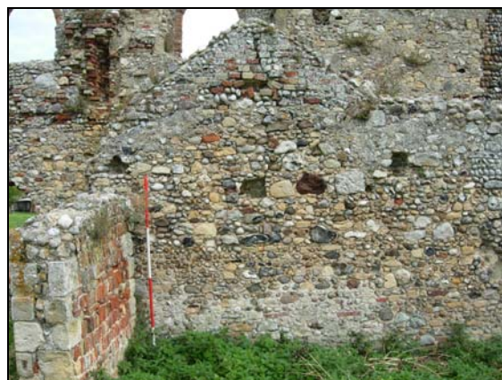
Plate 55 Wall 0052, south face with gable 0059
