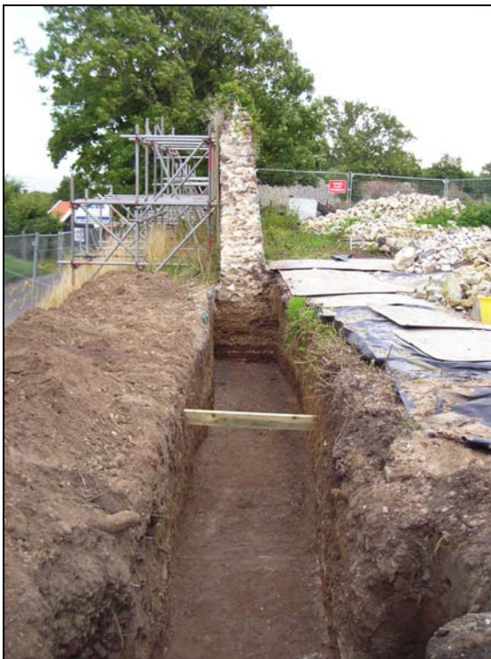
Plate 15 New footing trench, northern end
