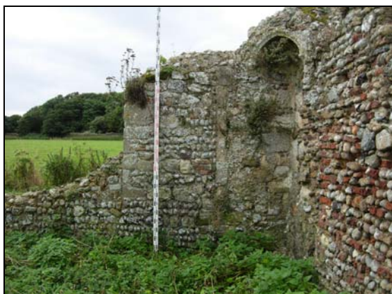
Plate 62 Wall 0056, west end internal face
