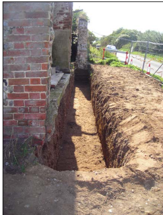
Plate 16 New footing trench, southern end
