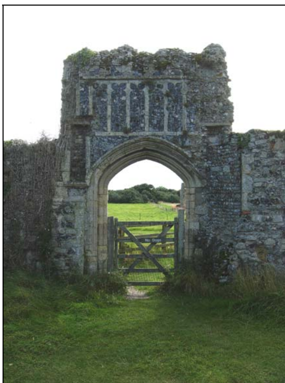
Plate 44 North gateway, external view
