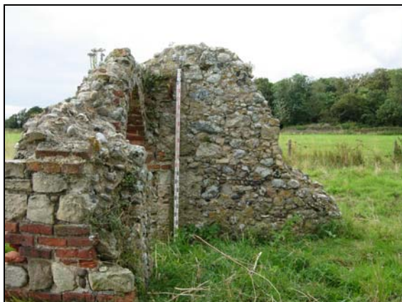
Plate 60 Wall 0056, east end internal face
