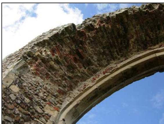
Plate 35 South gateway, internal view of arch, detail
