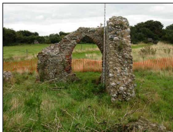
Plate 53 West wall 0057, internal view
