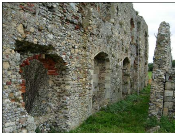
Plate 47 South face of wall 0050 from the west
