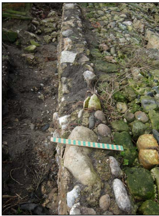
Plate 4 Toe on base of fallen wall section
