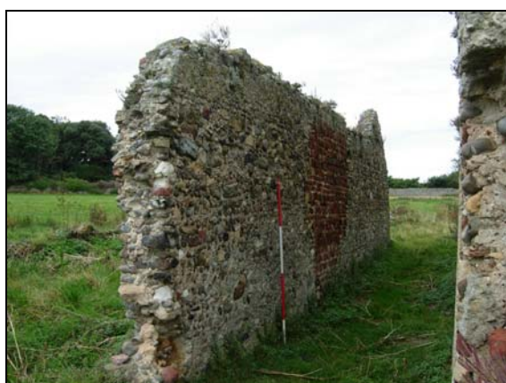
Plate 48 North face of wall 0052 from the east
