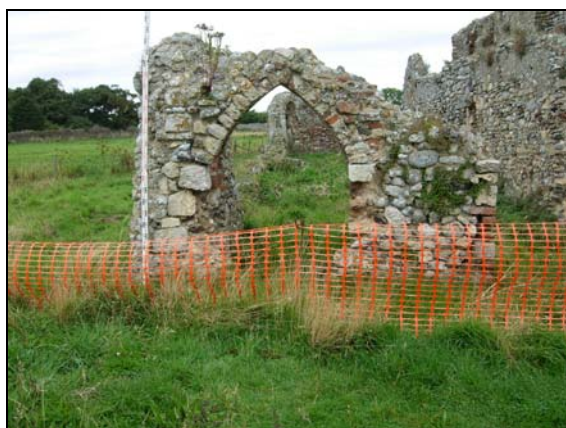
Plate 52 West wall 0057, external view
