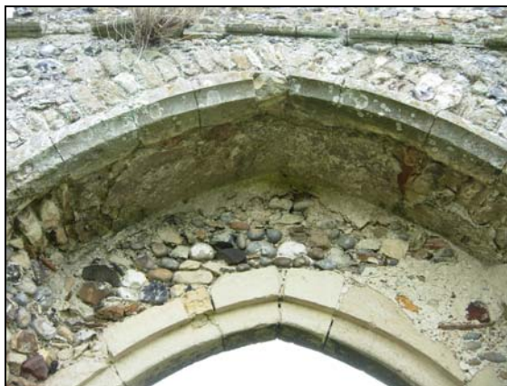
Plate 40 North gateway, detail of arch, internal
