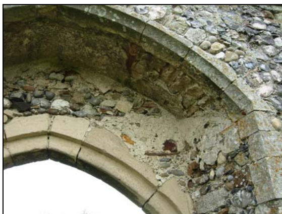
Plate 42 North gateway, detail of arch, internal
