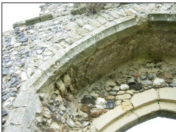
Plate 41 North gateway, detail of arch, internal
