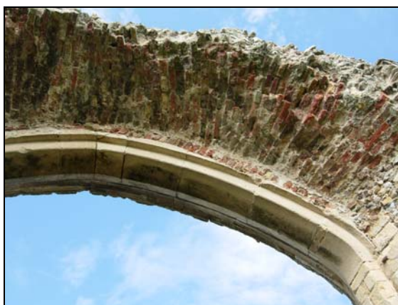
Plate 36 South gateway, internal view of arch, detail
