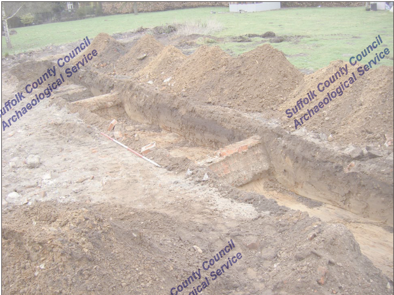
Plate 1. Wall footings and soakaway in Trench 2, looking north
