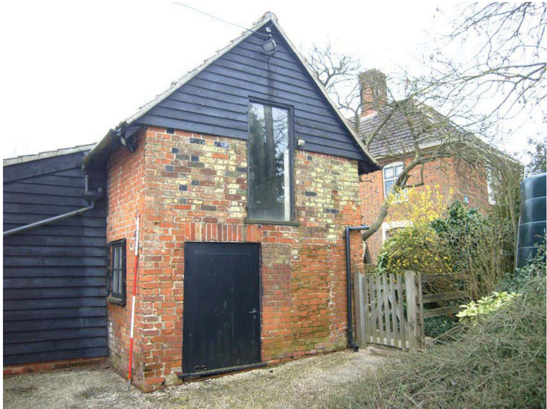
A2.3 Brick shed (1). Exterior of northern gable showing upper window of recent partial conversion and at least four phases of brickwork
