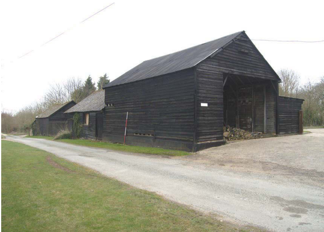
A2.2 General view of roadside sheds from west, showing the enclosed sheds (2) in foreground and the open shed (3) in the rear
