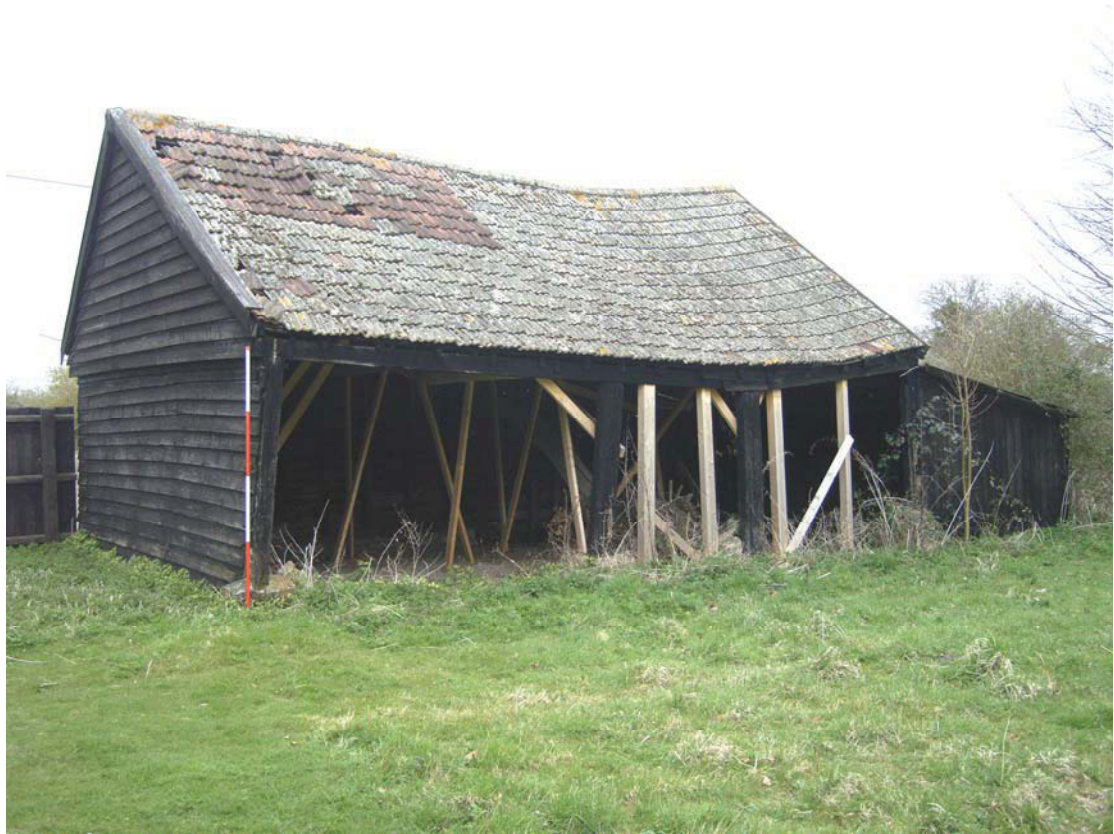
A2.9 Open shed (3). External southern elevation showing western gable to left.
