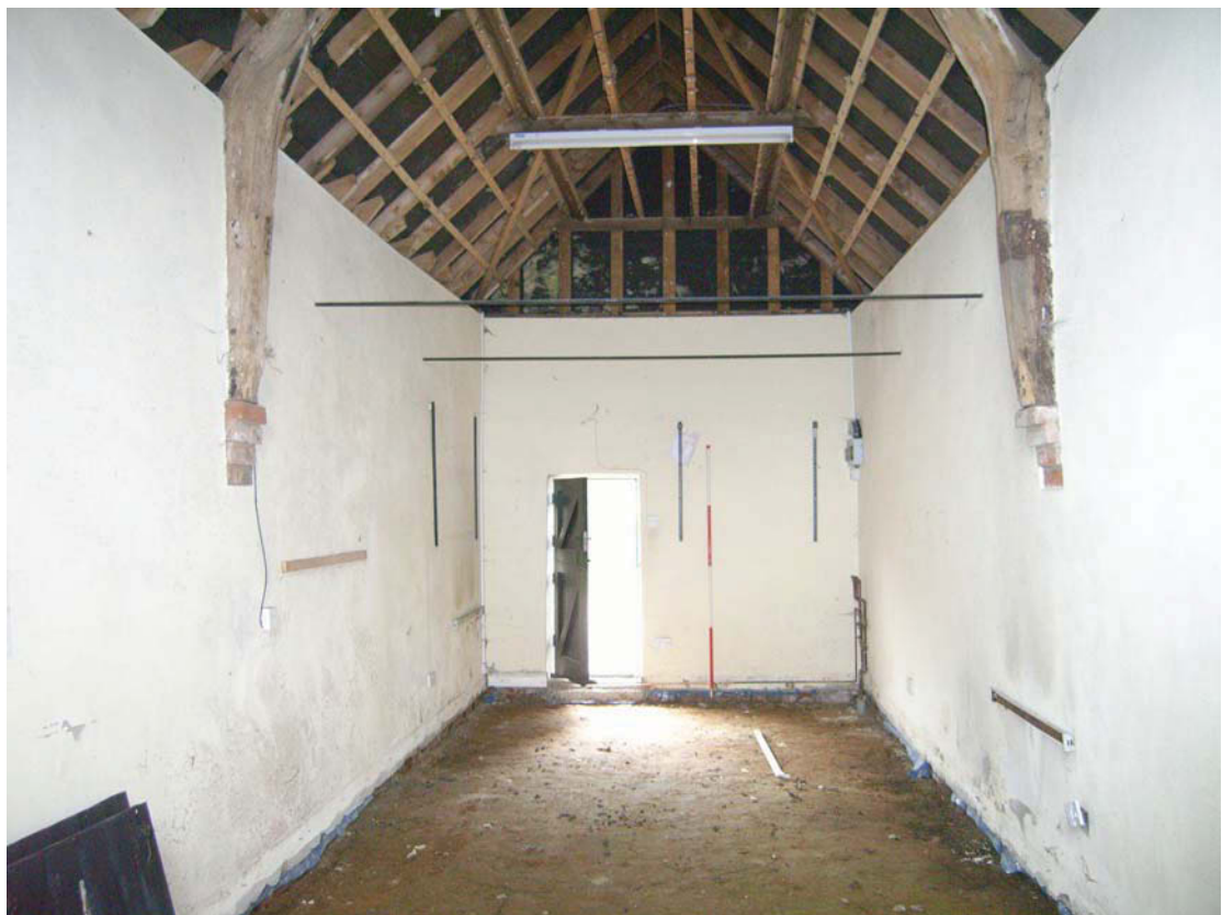
A2.4 Brick shed (1). Gutted interior from north
