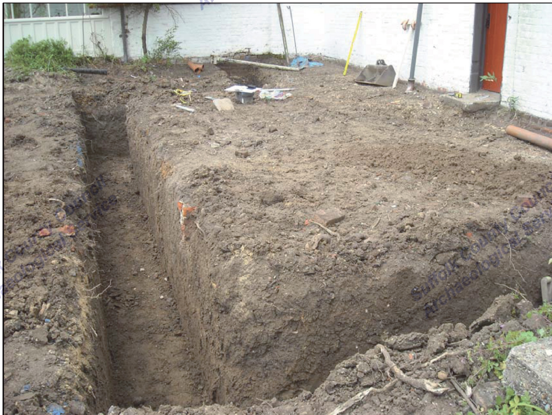
Plate 2. Footings trench from south-east
