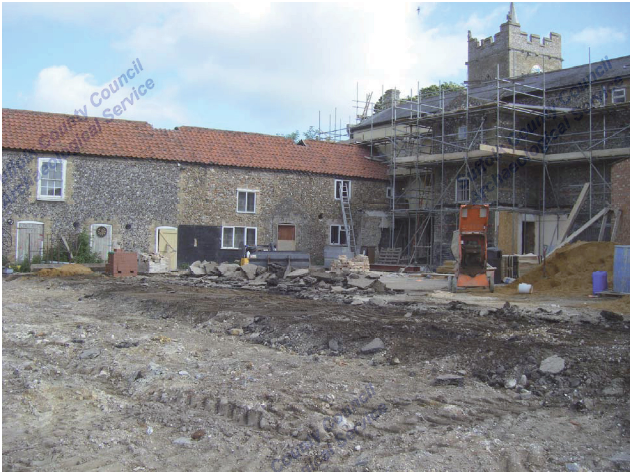
Figure 6. Cromwell Inn and courtyard looking north-east, pre-excitation of trench
