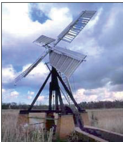
Plate 14: An extant example of a trestle mill
