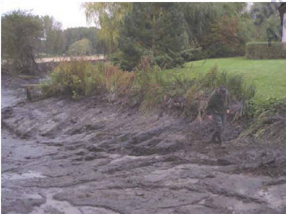
Plate 7. North east corner during de-silting, looking south west
