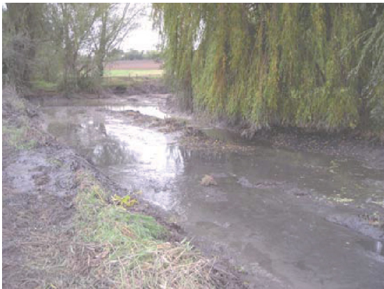
Plate 5. Southern end of the east arm during de-silting, looking south
