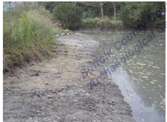
Plate 10. West end of northern arm after de-silting, looking west
