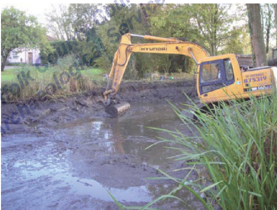
Plate 1. North west corner of moat during desilting, looking south east
