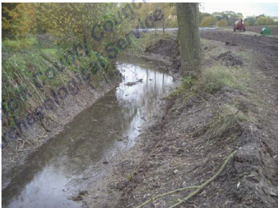
Plate 9. South west corner of moat after de-silting, looking south
