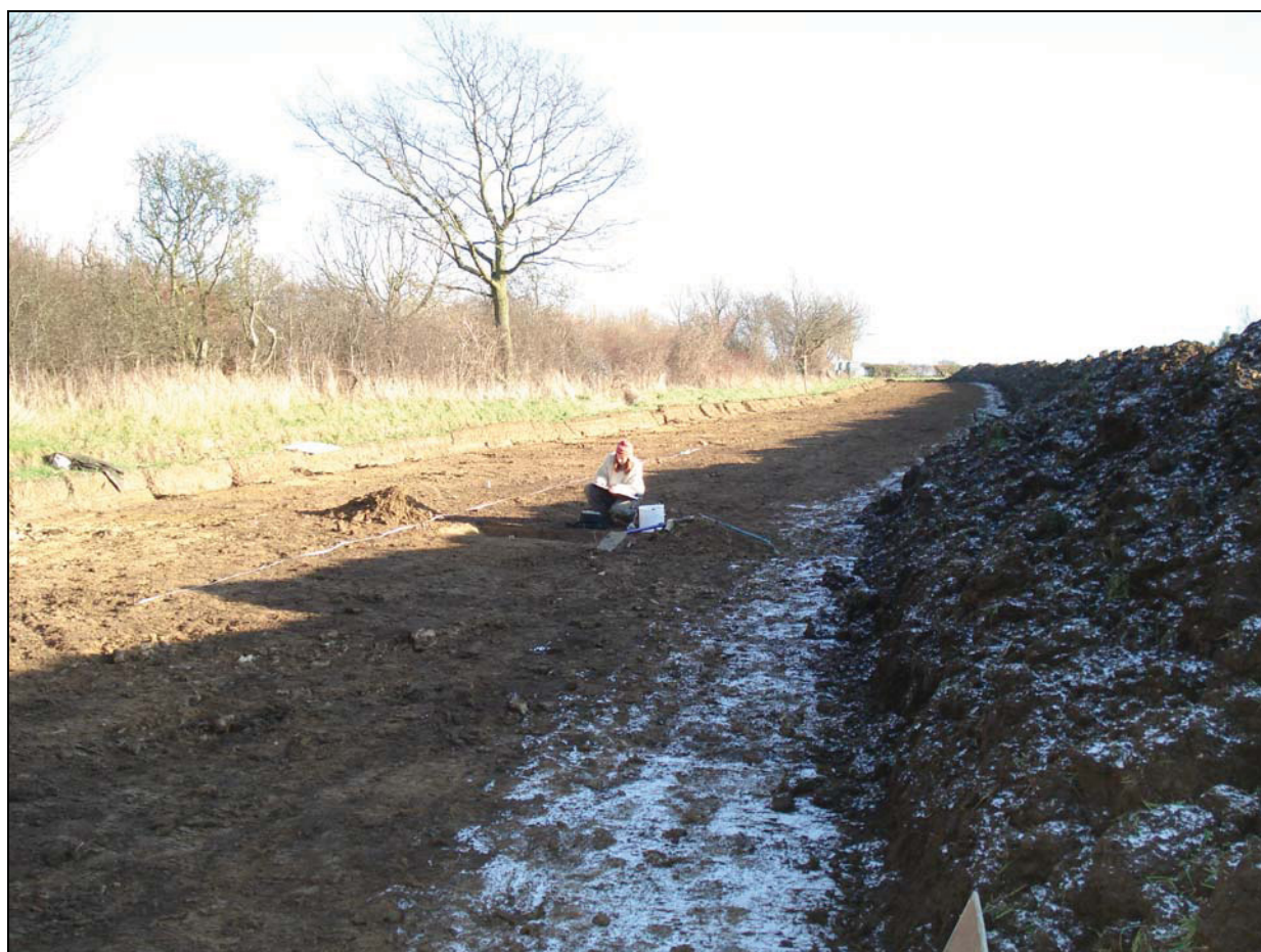
Plate 1. Excavation area, facing east
