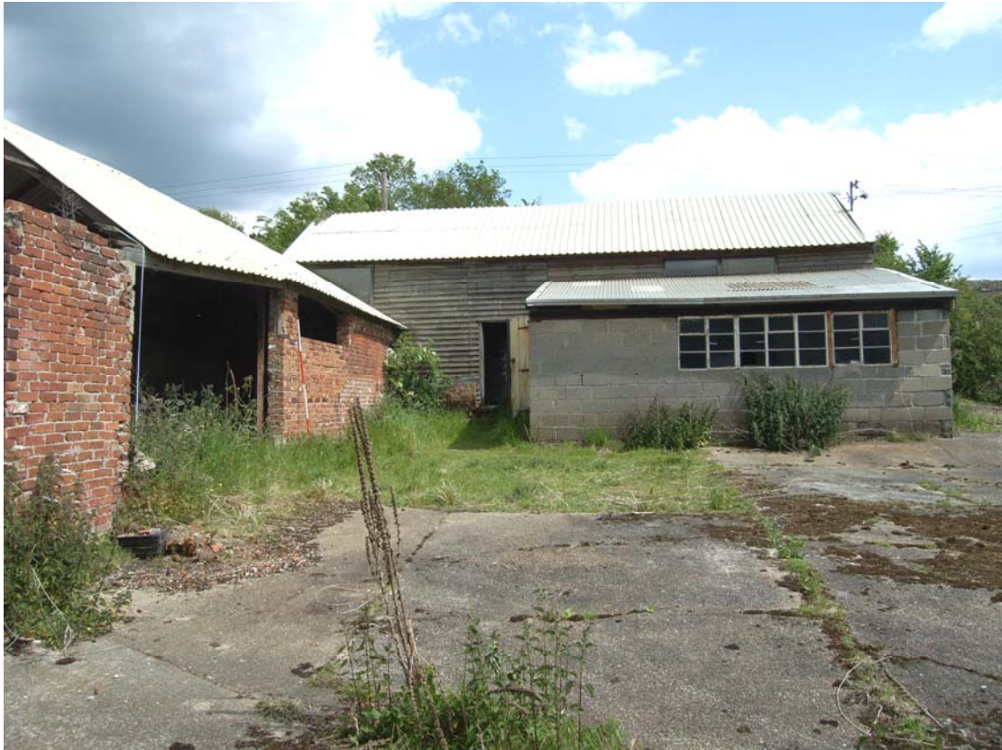
A2.9 Western external elevation of timber-framed and weatherboarded barn (4) showing brick shed (3) to left & block-work lean-to shed (5) to right
