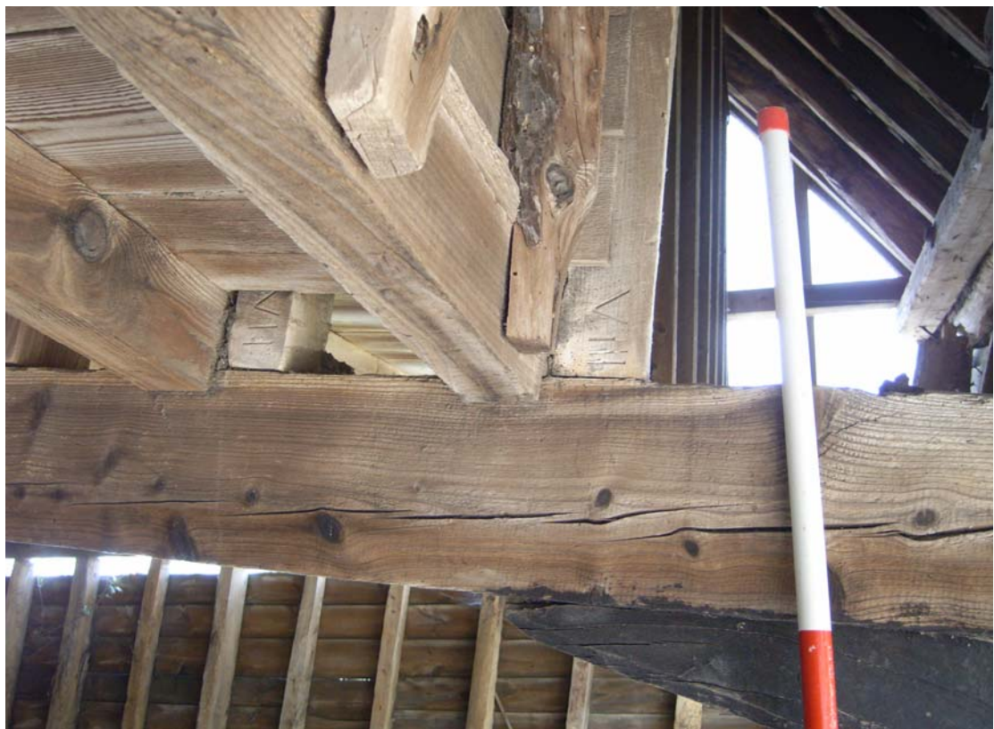
A2.8 Detail from south of granary floor showing carpenters' numerals to internal studs
