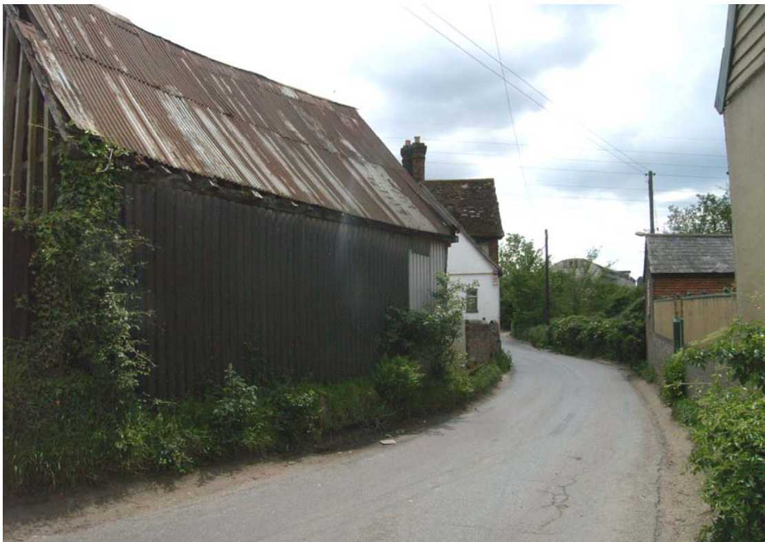
A2.4 Western external elevation of the granary seen from Paper Mill Lane to north-west, showing corrugated iron roof and cladding with farmhouse in rear
