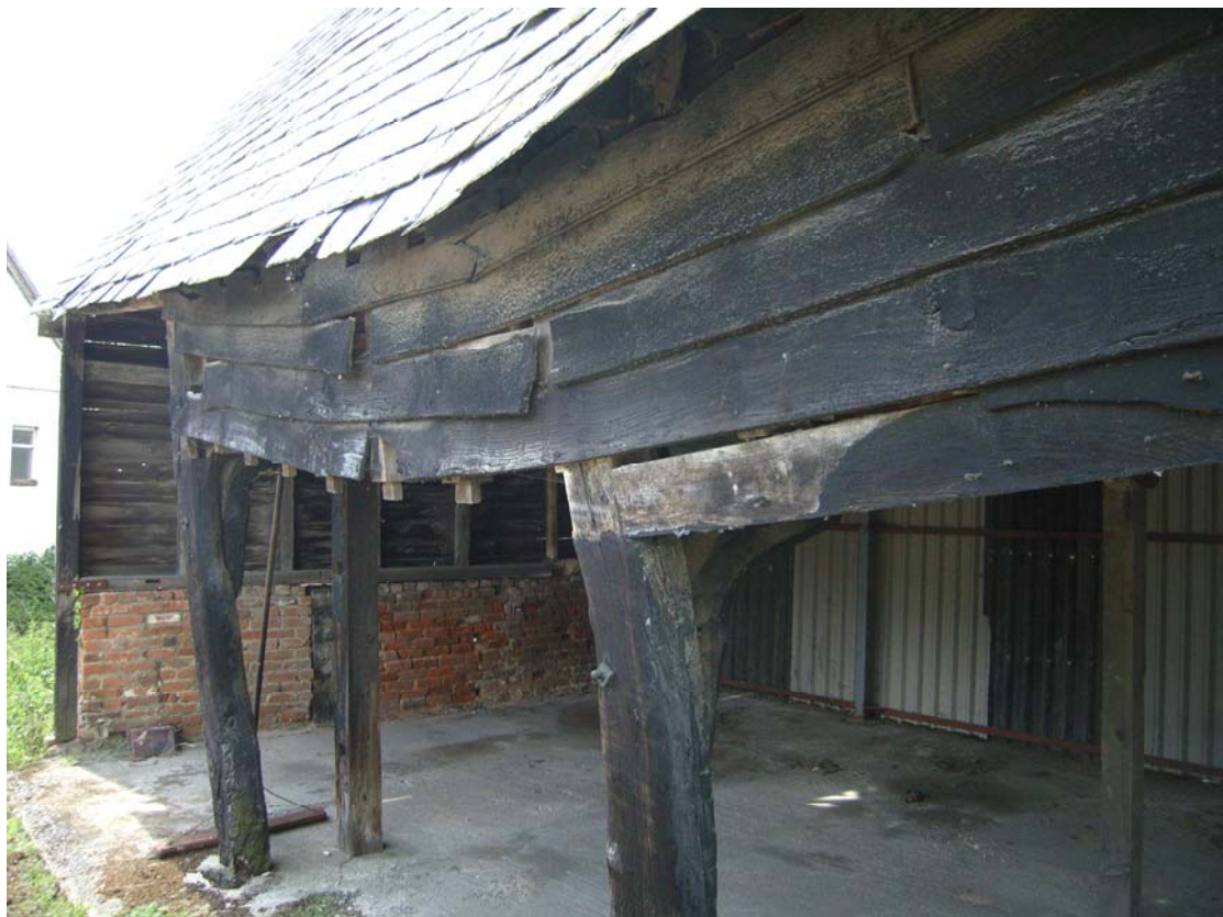
A2.6 Detail of external eastern elevation of granary from north-east showing tarred weatherboarding to granary storey and removed mid-rails to central and southern bays
