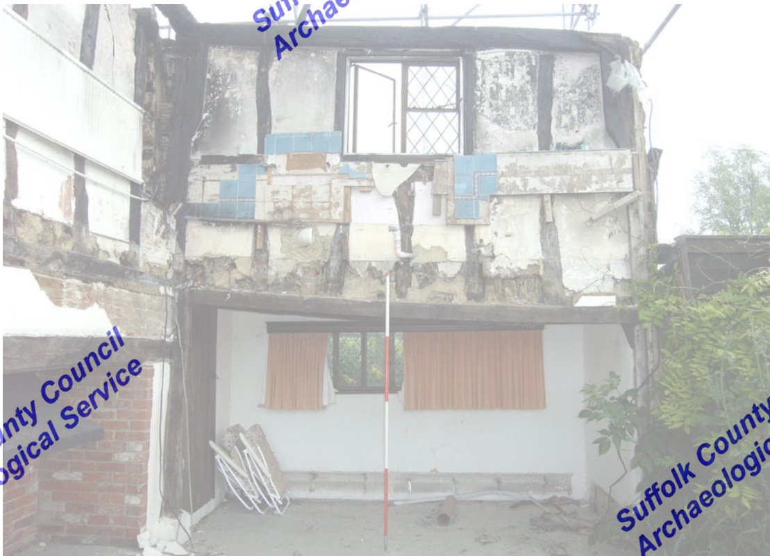
A2.6 Internal elevation of rear cross-wing gable C-D, showing an original first-floor window without a shutter rebate and extensive sooting to all studs and daub
