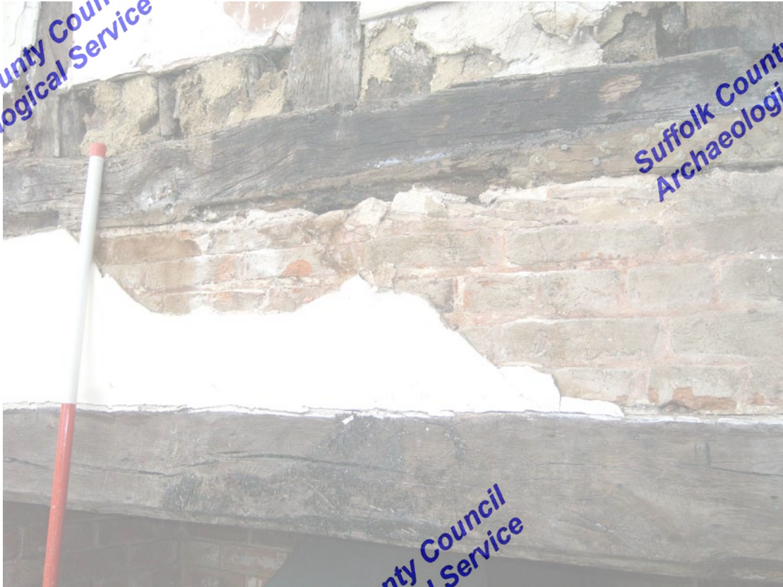
A2.5 Detail of mid-rail in bay E-C showing well-preserved reddled 17 th century brickwork and an unusually narrow medieval window shutter rebate
