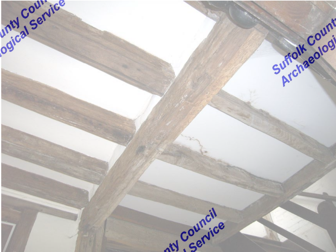
A2.11 Ceiling of entrance lobby from south showing mortises of 17th century door in mid-rail with stair trap to right and re-used roll-moulded timbers of modern porch to left
