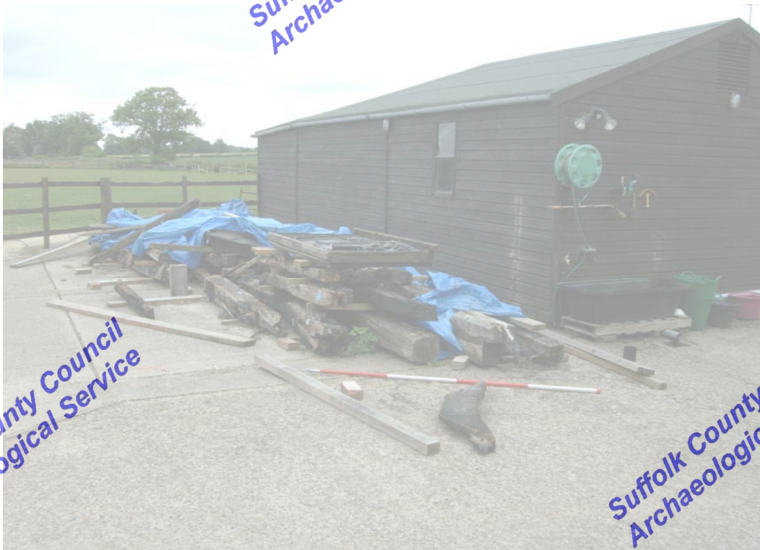
A2.12 Substantial pile of dismantled timbers to south of site, labelled for re-assembly but not fully examined. Note the tie-beam arch brace in the foreground (probably from truss J-K).
