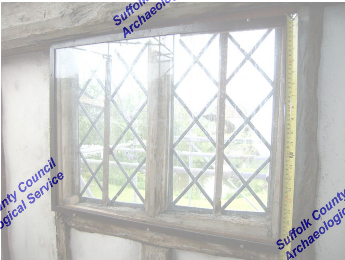
A2.10 Detail of original ovolo-moulded first-floor window in western elevation of chimney bay, retaining mullion and diamond-section wooden saddle bars
