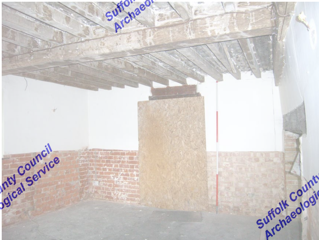
A2.8 Ground floor of 17th century hall from west, showing intact ceiling and secondary door in elevation A-B with fireplace to right and blocked door in northern gable to left
