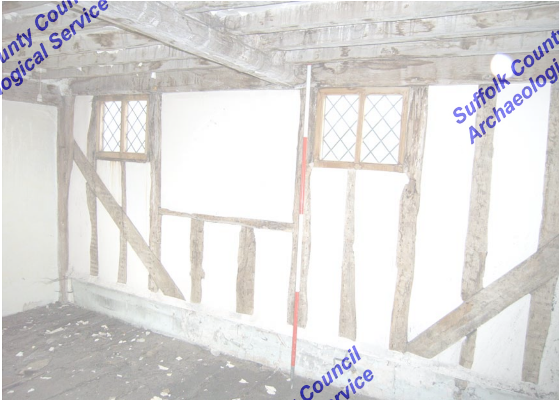
A2.9 Internal elevation of northern gable G-A of hall chamber, showing original ceiling joists and off-centred tripartite window with original sills but modern mullions
