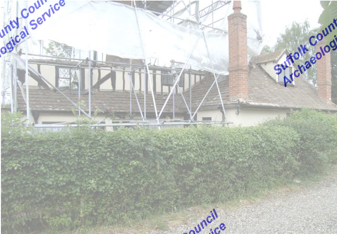
A2.3 Rear elevation from east showing the symmetrical braces of the medieval cross-wing's hipped gable to the left and the intact 17 th century four-light ovolo-moulded window to the right
