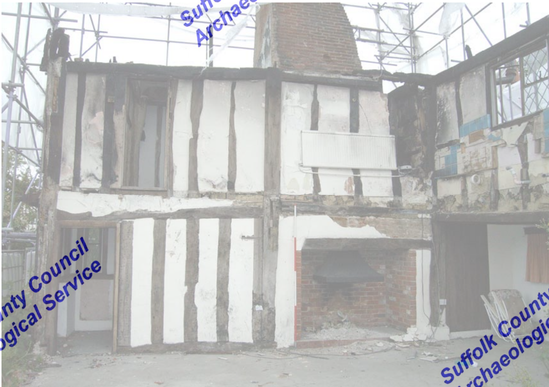
A2.4 Internal northern elevation of the medieval cross-wing (J-E-C), showing the 17 th century chimney to the right. The structure originally continued by at least one bay to the left. The right-hand bay was originally partitioned and its internal studs are soot-encrusted
