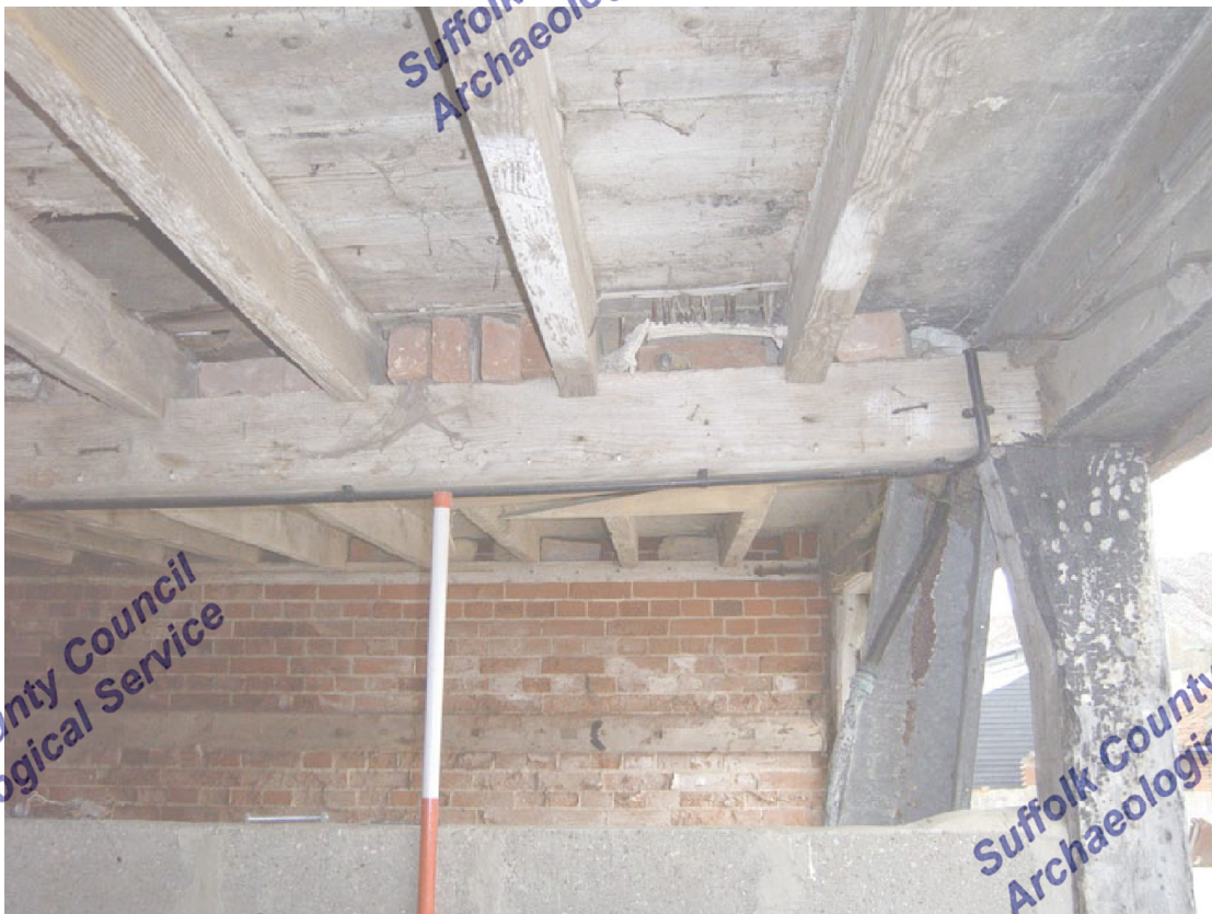
A2.6 Detail of softwood ground storey ceiling from south, showing post of open arcade to right
