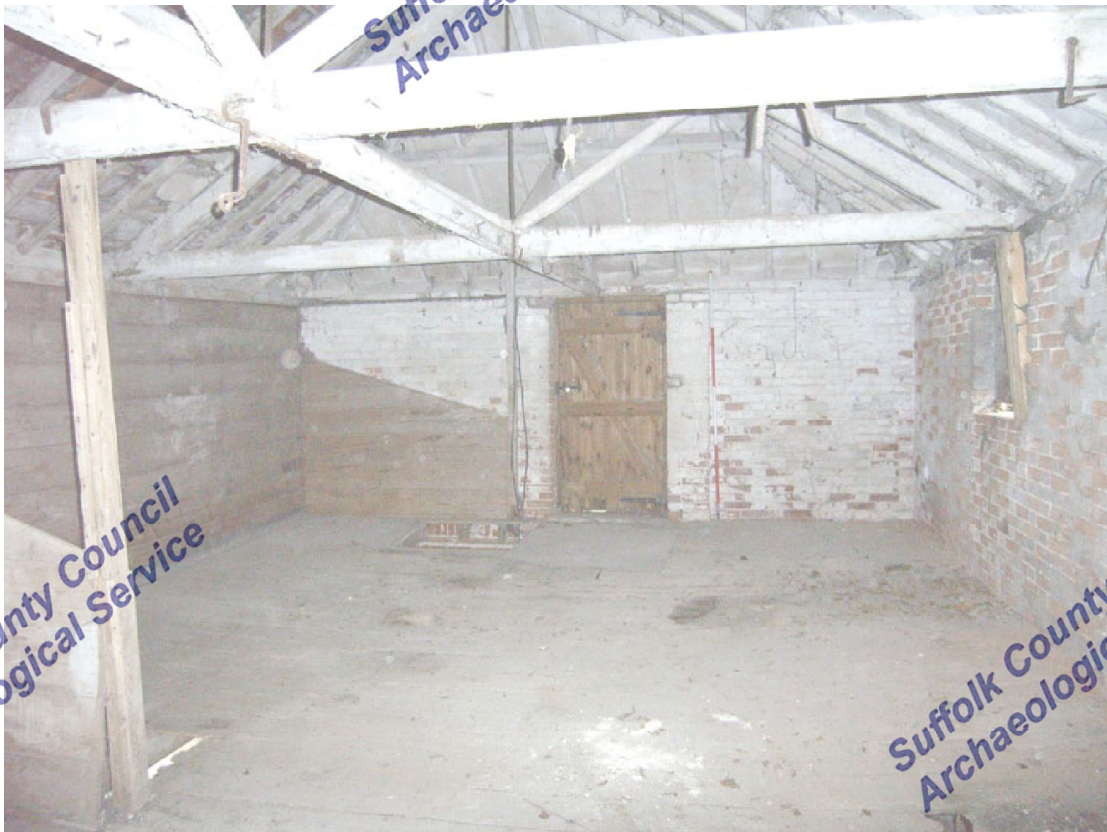
A2.8 Interior of granary showing original gable entrance door adjacent to existing internal stair trap
