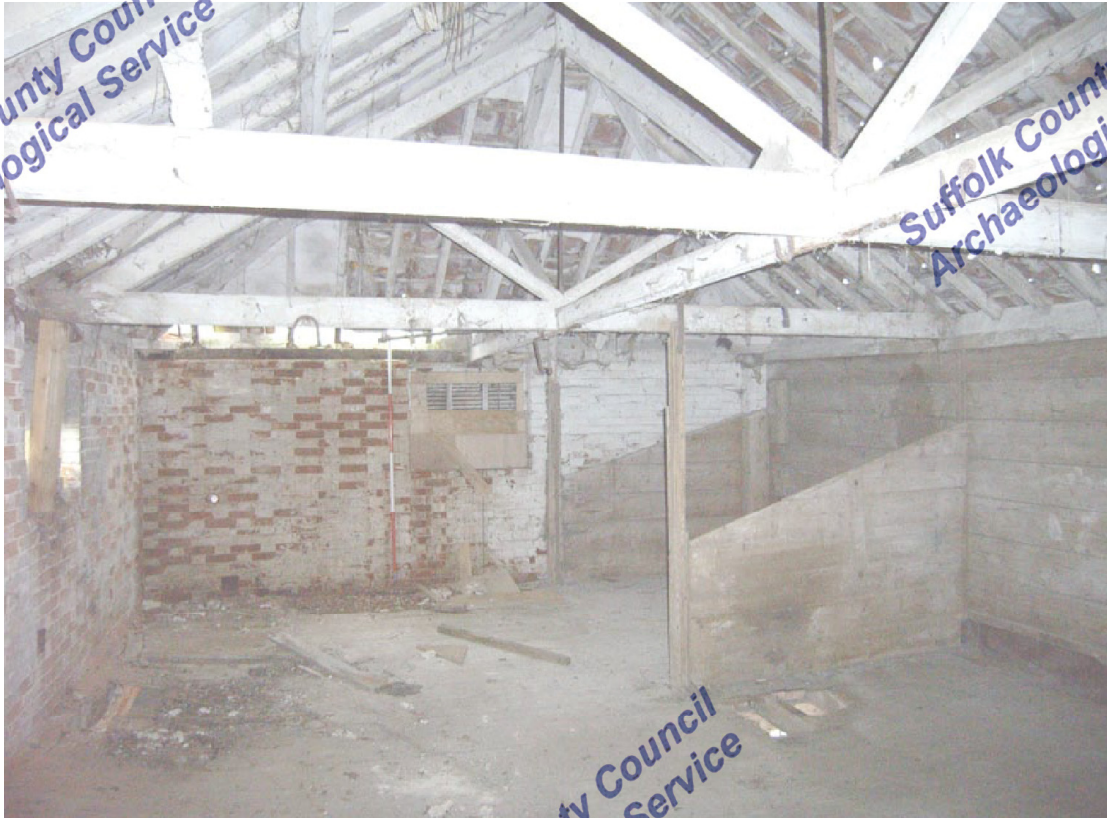
A2.7 Interior of granary on upper storey from south, showing boarded grain bins to right and central window in northern gable blocked externally by secondary shed
