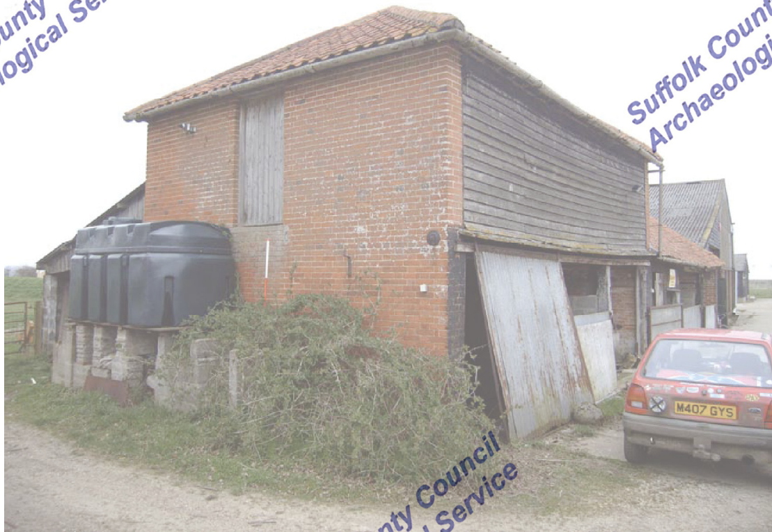
A2.3 Exterior from south-east showing original granary door in southern gable
