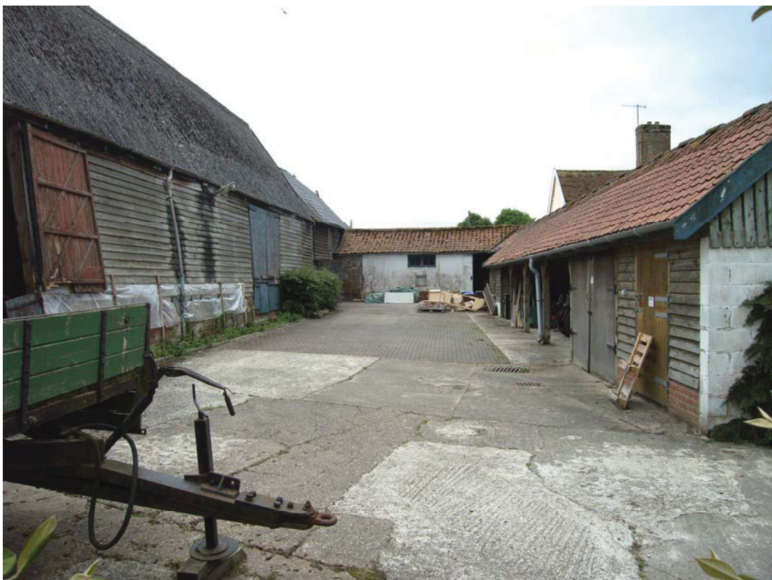
A2.2 General view of yard from north showing barn (A) to left and much rebuilt shelter shed (D) to right.
