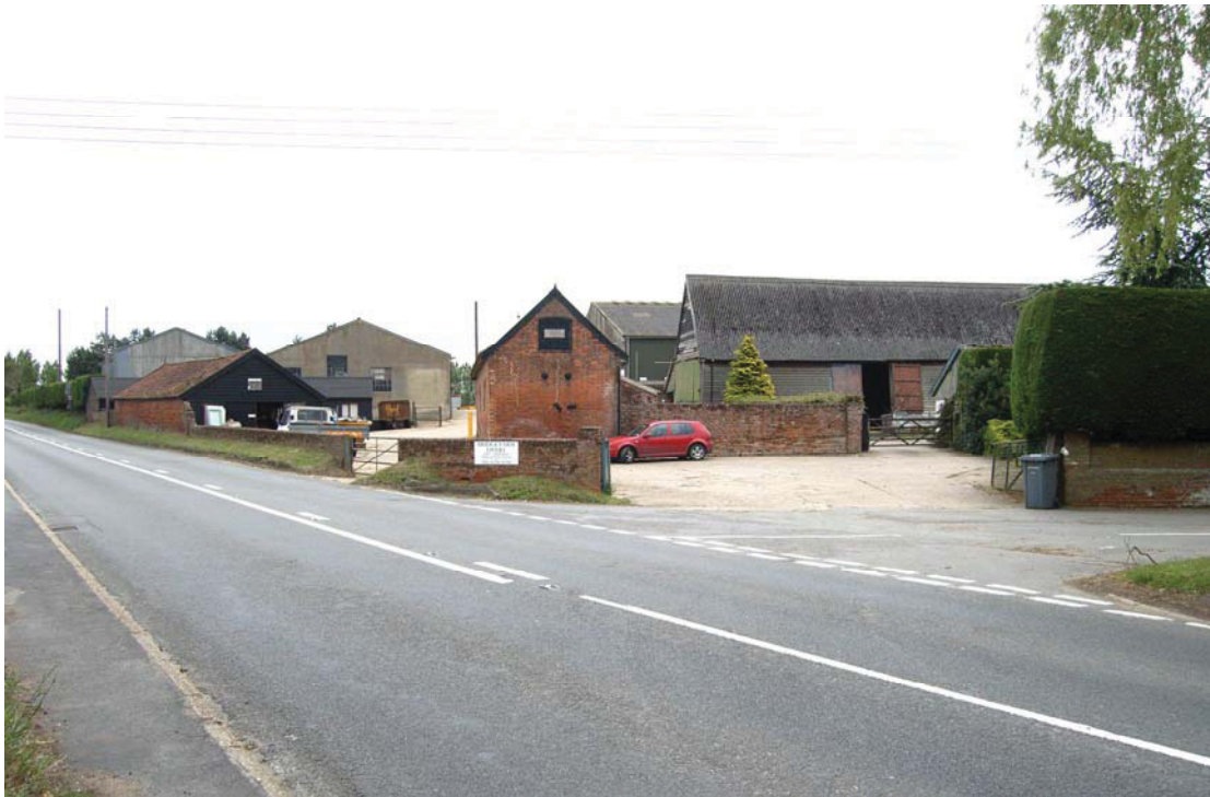
A2.1 General view of entrance to site from main road (B1078) to north-west, showing barn to right with converted brick shed and 20 th century buildings to left
