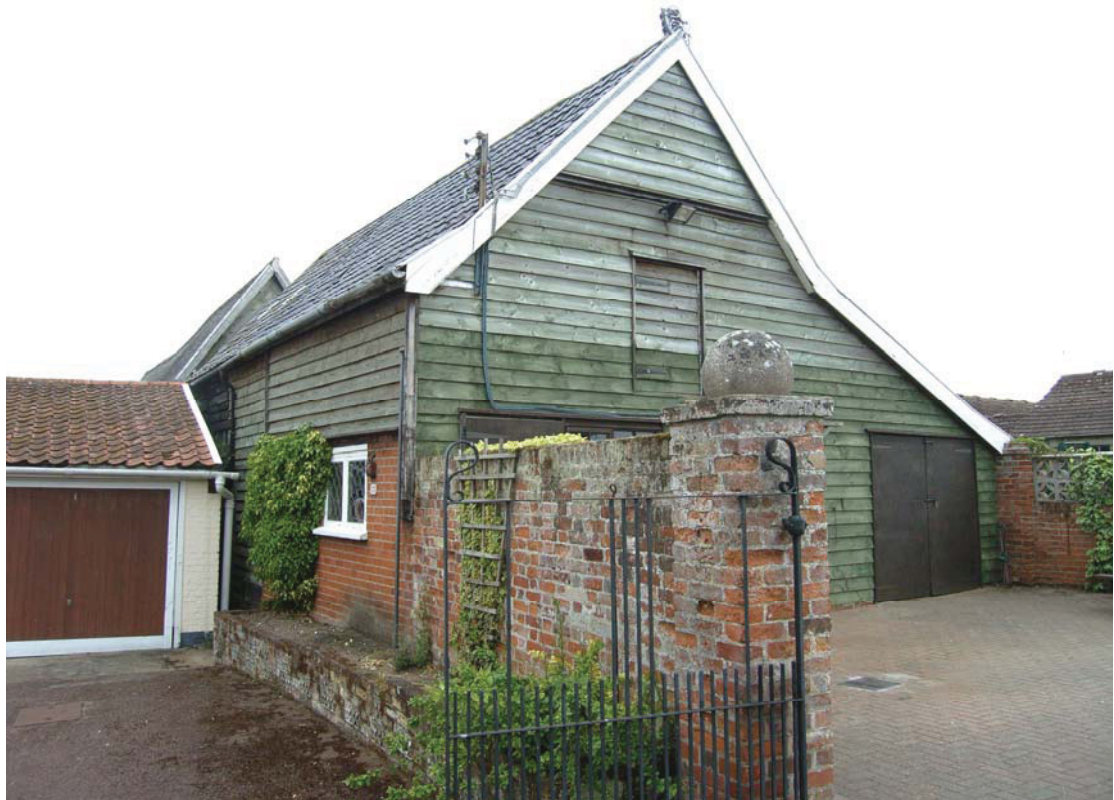
A2.10 Exterior of granary (B) from south-east showing the rebuilt western elevation to the left with blocked loading door in the gable
