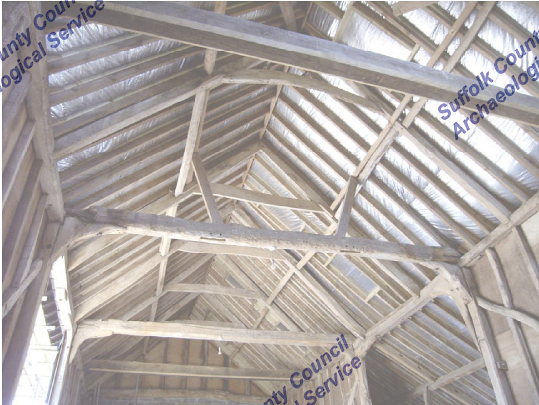
A2.5 Butt-purlin roof structure from south showing re-used tie-beam with arch-brace mortises.
