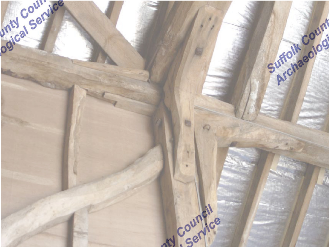
A2.7 Detail of original bolted knee-braces, pegged and tenoned primary brace and face-halved and bladed scarf joint to north of lean-to porch
