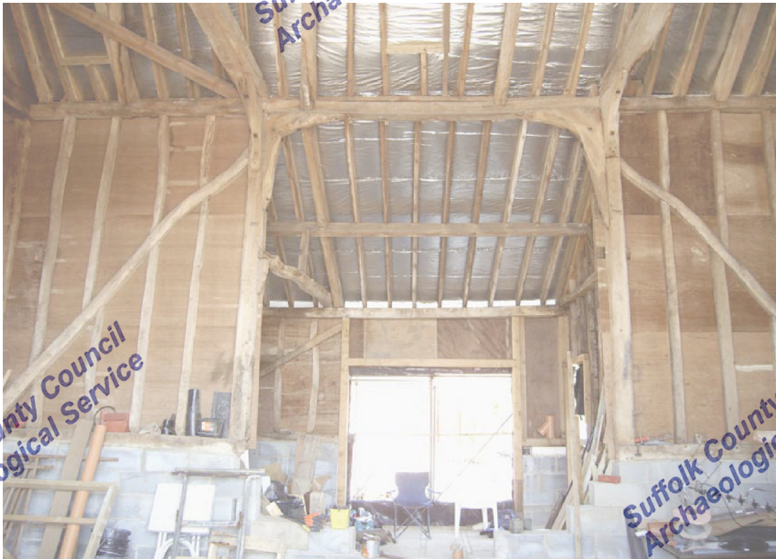
A2.6 Internal eastern elevation of central bay showing access to lean-to porch and position of original external door (jambs and lintel renewed).
