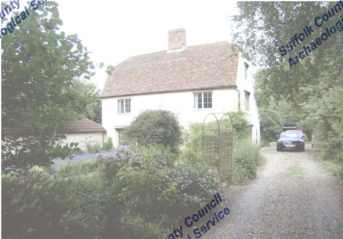
A2.1 Approach to site from south-west, showing the facade of Picknotts house with the barn in rear to right and the single storied shed belonging to the Thatchers to left
