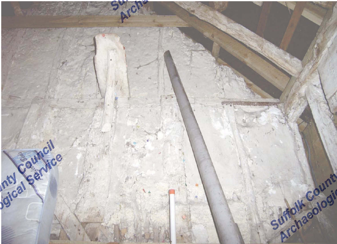
A2.6 Detail of internal partition from northern shed showing projecting hook with wattle-and-daub infill.
