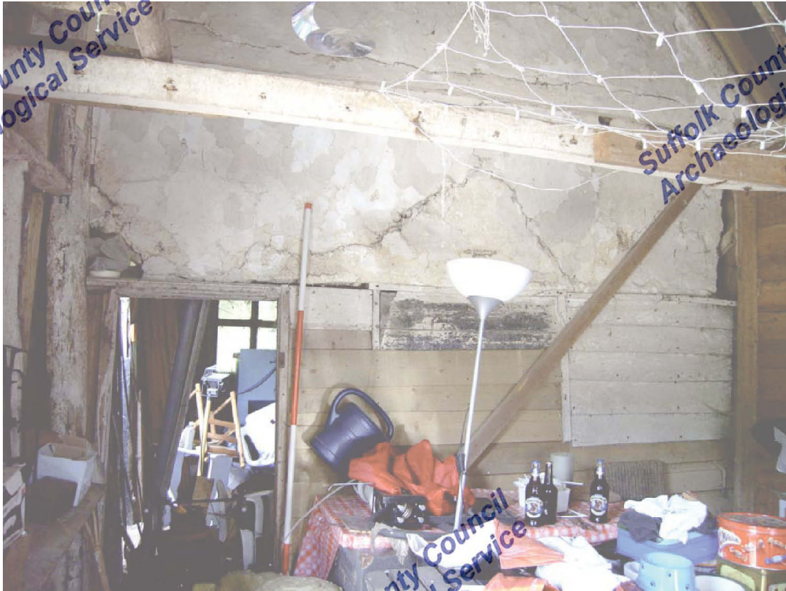
A2.7 Internal partition seen from southern shed showing blocked central window and connecting door to left
