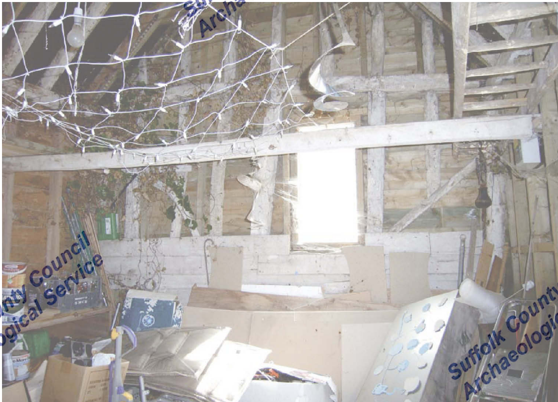
A2.8 Internal southern gable showing original studwork with primary bracing and bentwood hook to left of modern window
