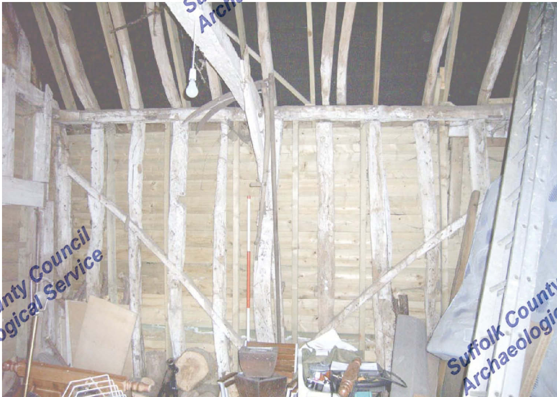
A2.4 Internal rear elevation of northern shed showing original studs and primary bracing with open truss in centre
