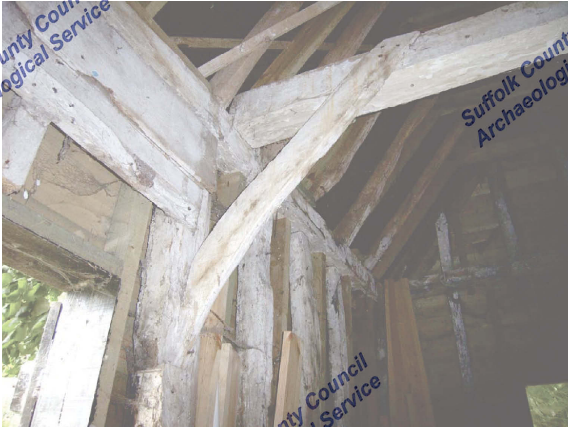
A2.5 Detail of from south of open truss in northern shed, showing tenoned and pegged junction with wall post and nailed attachment to tie-beam, with external door to left.
