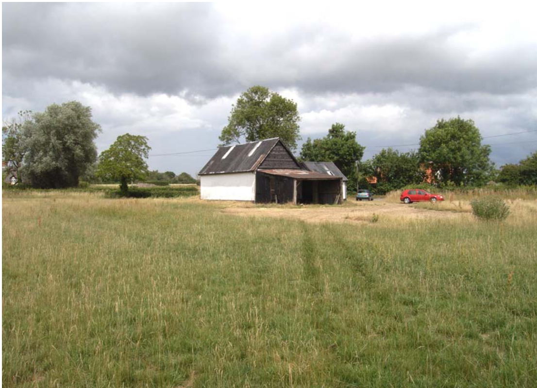
A2.1 General view of site from south-west showing isolated location of barn at field edge
