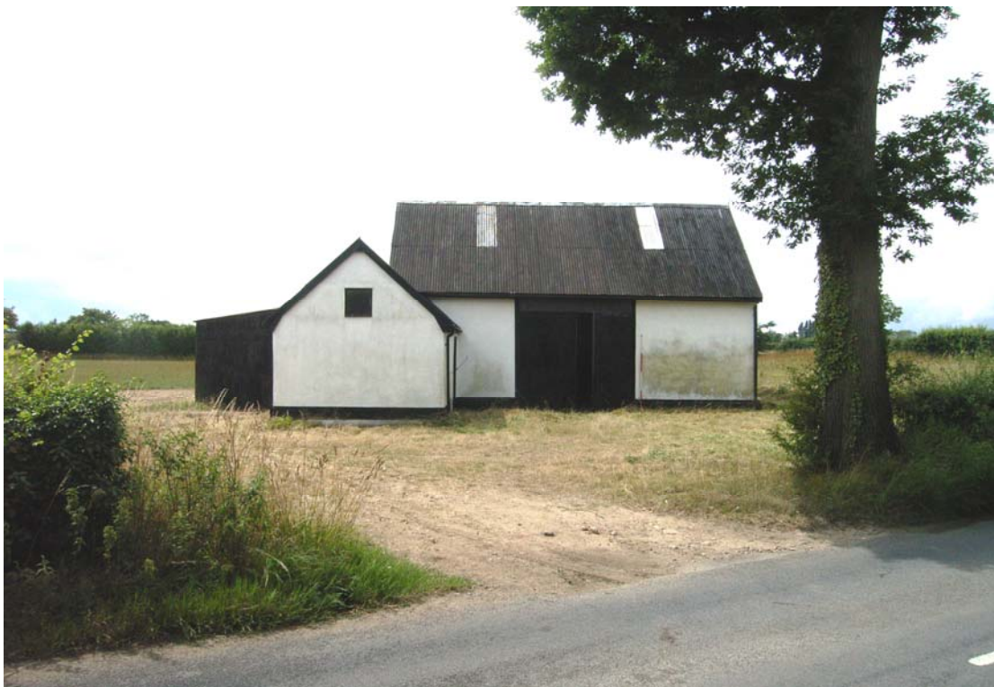
A2.2 General view of barn from Mellis Road to east, showing modern doors to the original barn entrance and the clay-lump shed to the left
