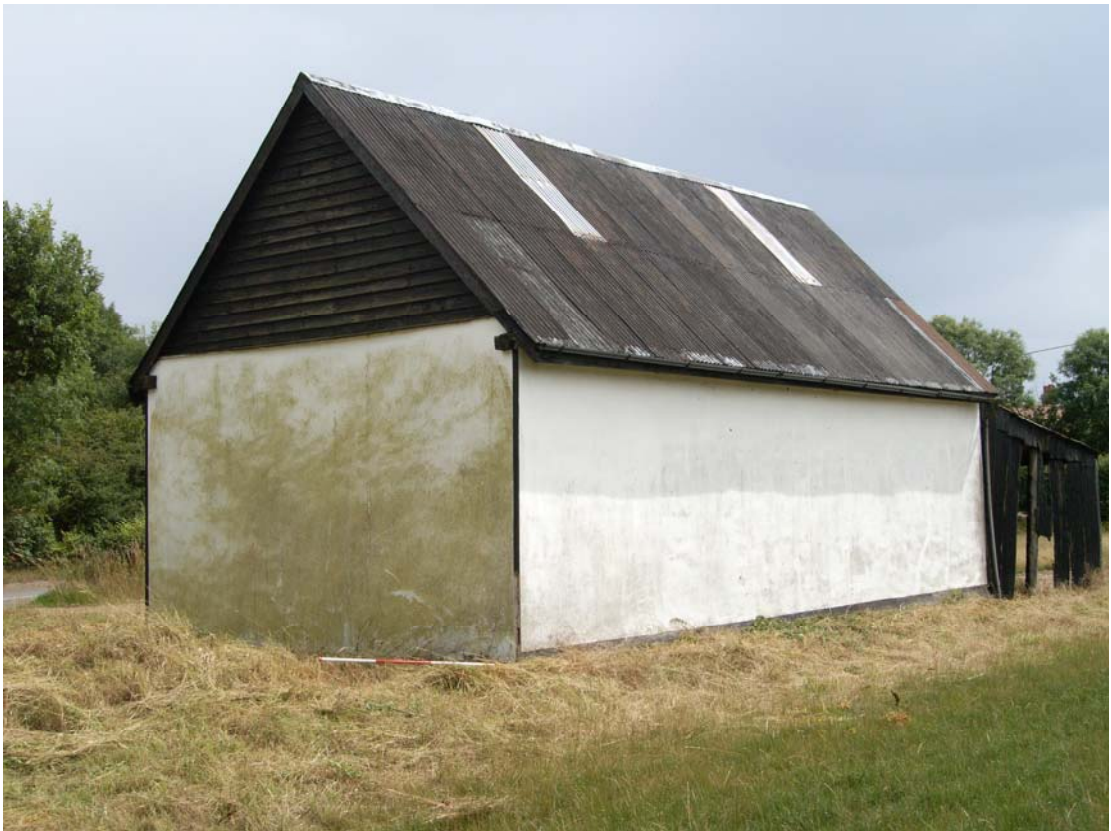
A2.4 Exterior from north-west showing modern render and corrugated iron roofing
