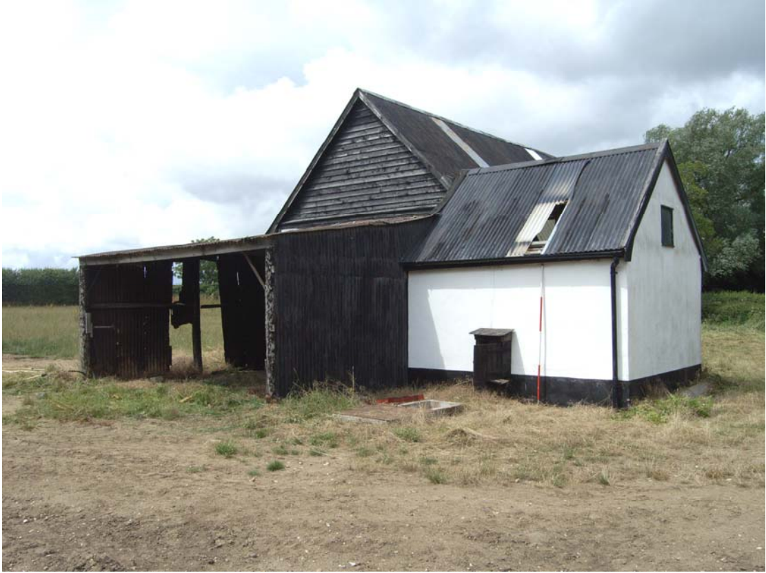
A2.3 Exterior from south-east showing clay-lump shed to right and lean-to shed to left with southern gable of barn in centre
