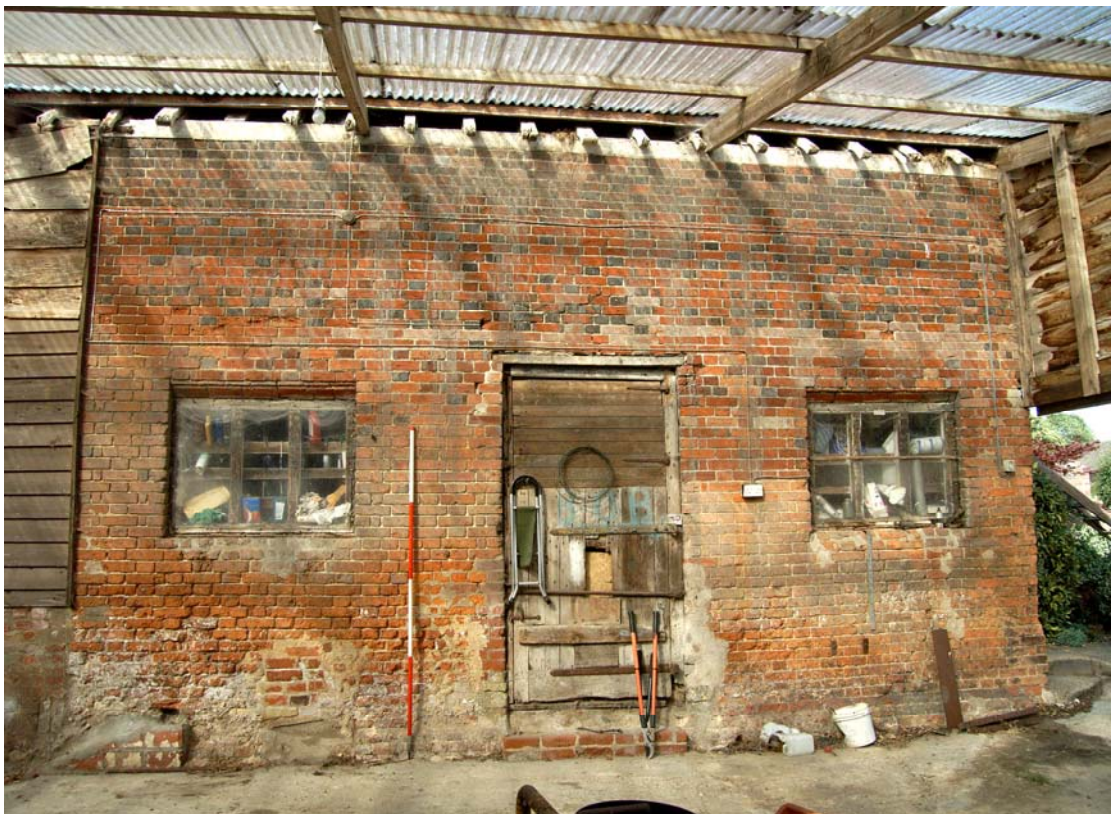
A2.4 External south-western facade of brick stable (1) from covered yard showing original door and windows
