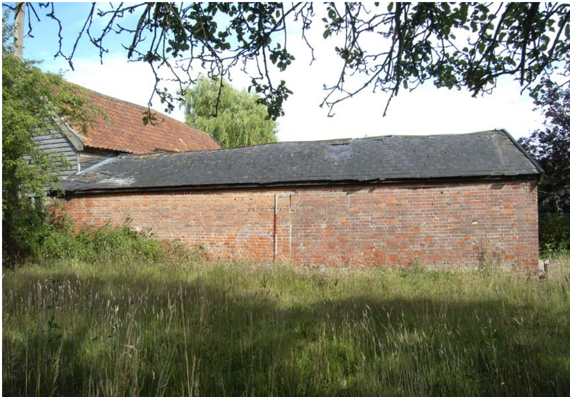
A2.10 External north-western elevation of the shelter shed and loose box (3 & 4) showing the north-western gable of the timber stable (2) left and the joint in the brickwork to the right of the scale rod
