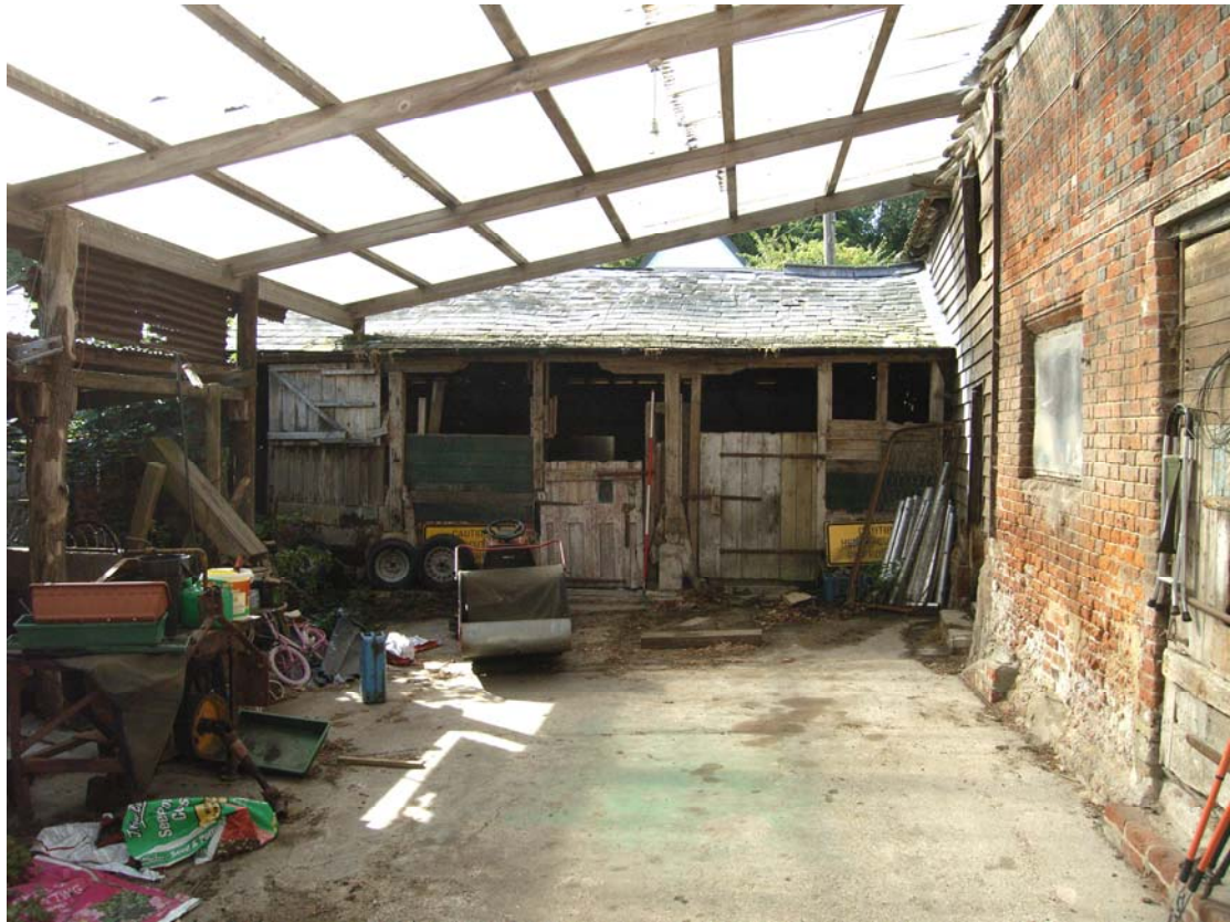
A2.11 Covered yard from south-east showing the open-sided shelter shed (3) with two original arcade posts and later loose-box doors in rear
