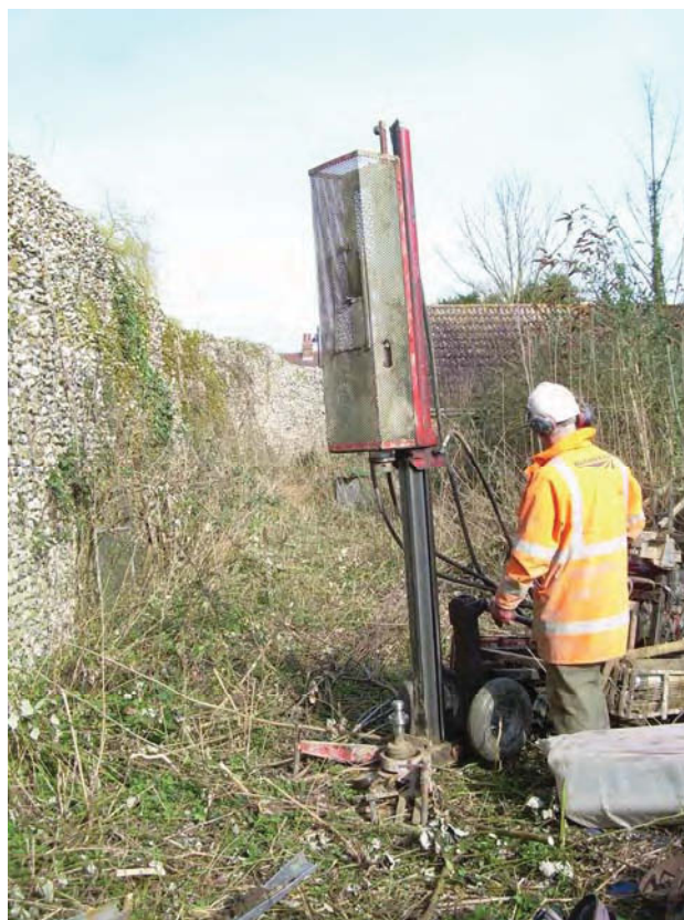
Plate 2: Site A coring rig
