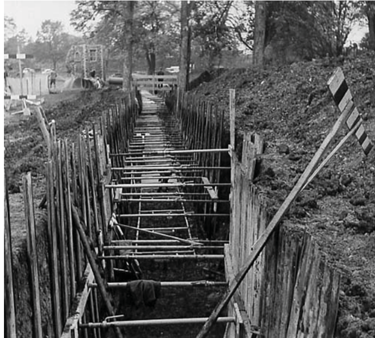
Figure 12. Excavations to lay or relay the main sewers in 1961/2
