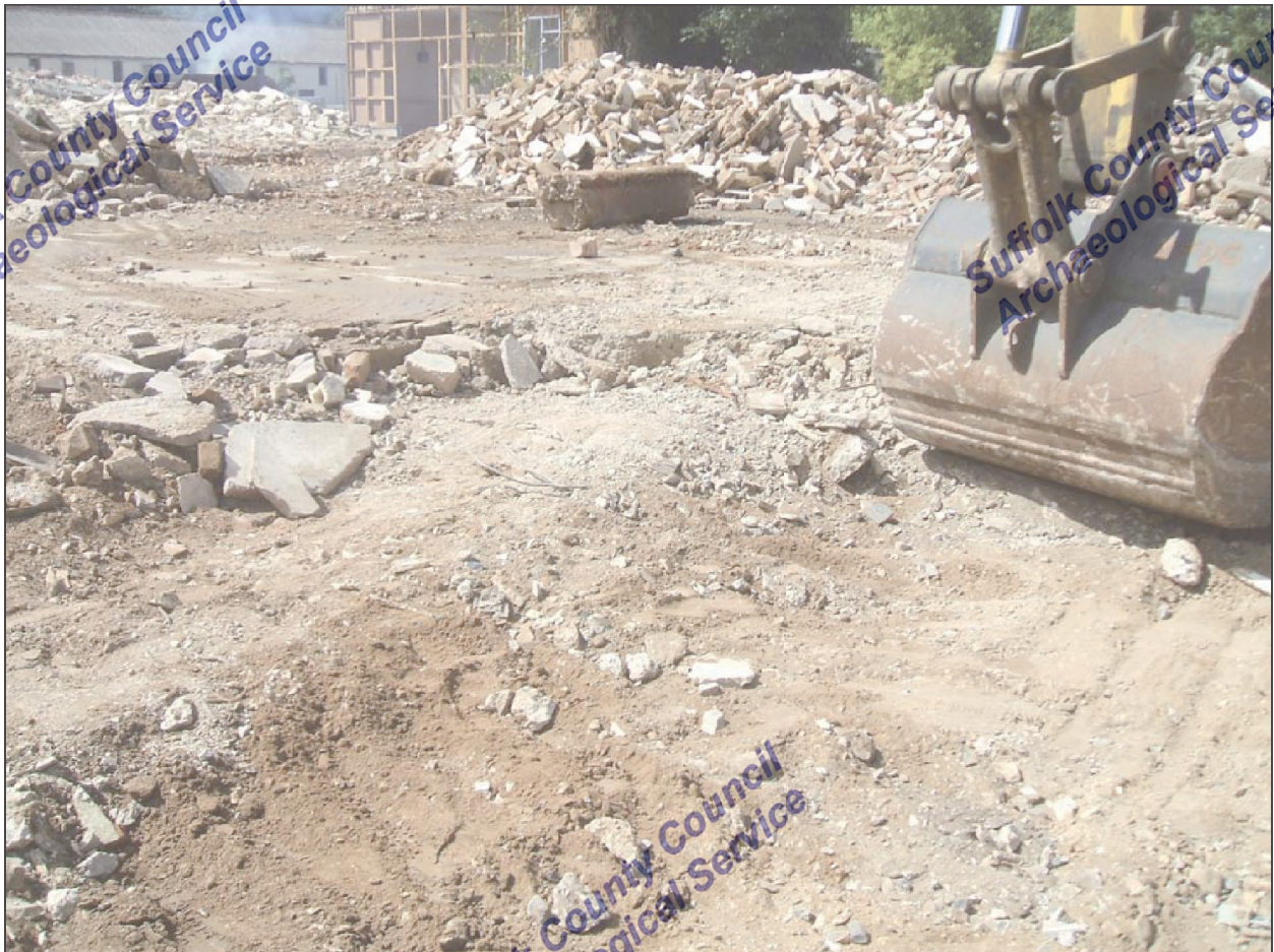
Plate 1. Monitoring removal of concrete slab foundations
