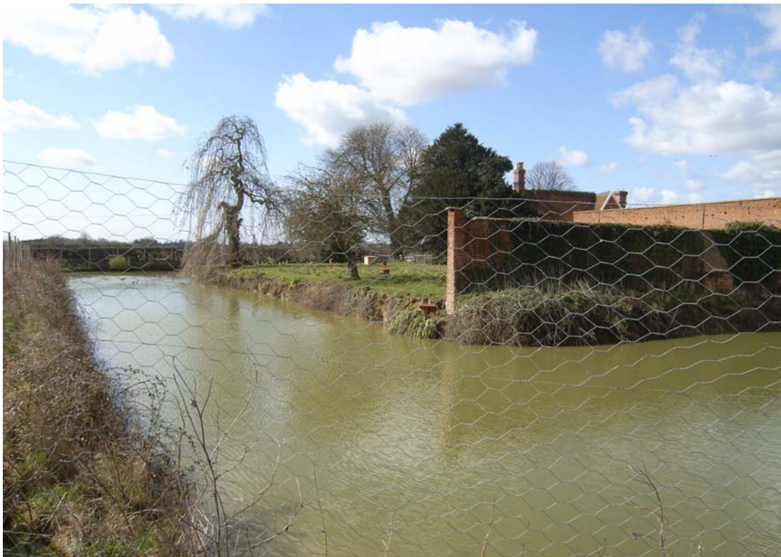
A2.2 General view from north-east across moat showing proximity of farmhouse in rear to left and high wall of eastern shelter shed (12) in rear to right
