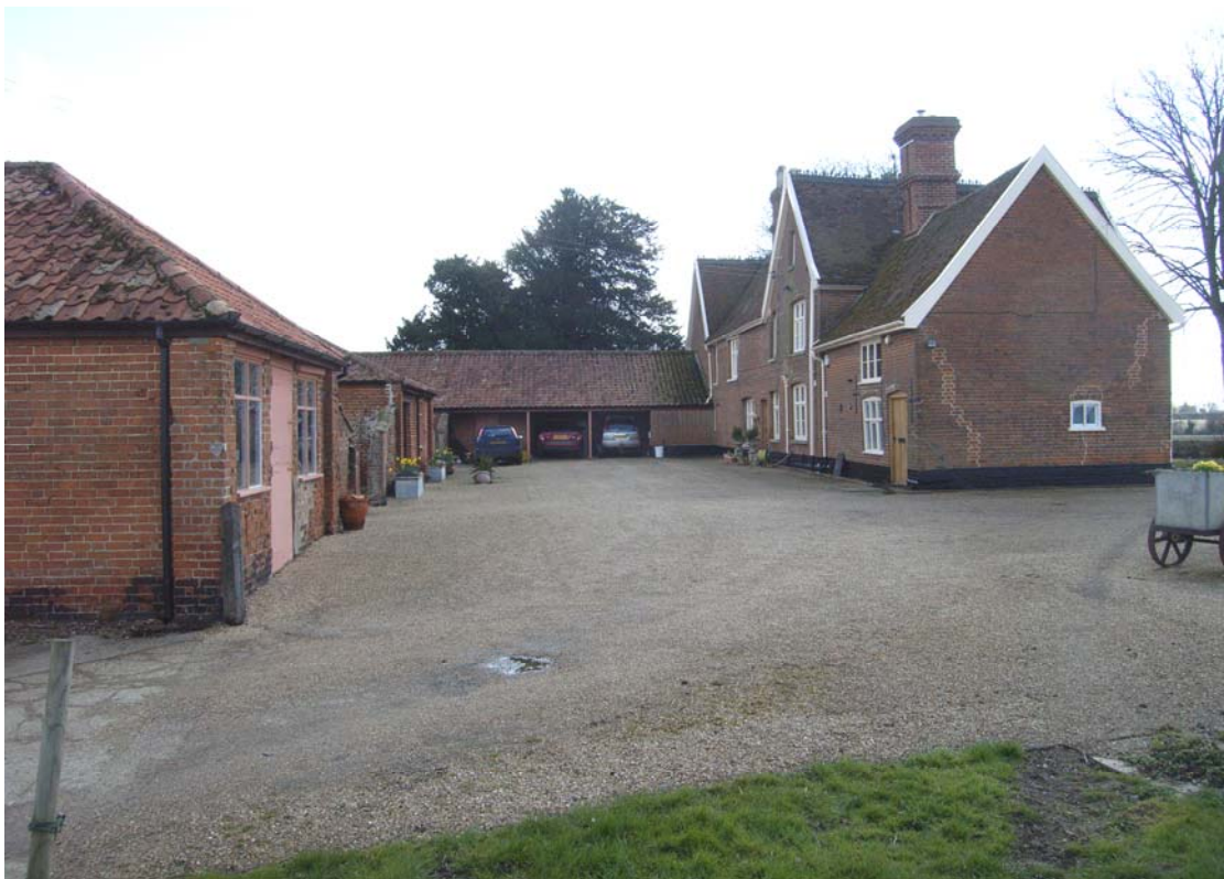
A2.4 Southern gables of yard sheds from west, showing proximity of farmhouse to right
