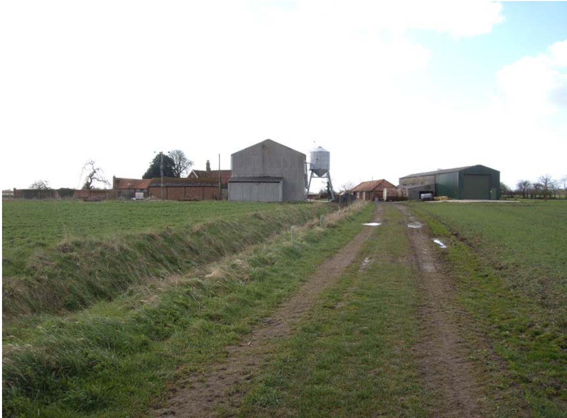
A2.3 General view of site from field to north-east showing modern sheds and silo in centre foreground with yard complex and farmhouse to left and detached cartlodge to right
