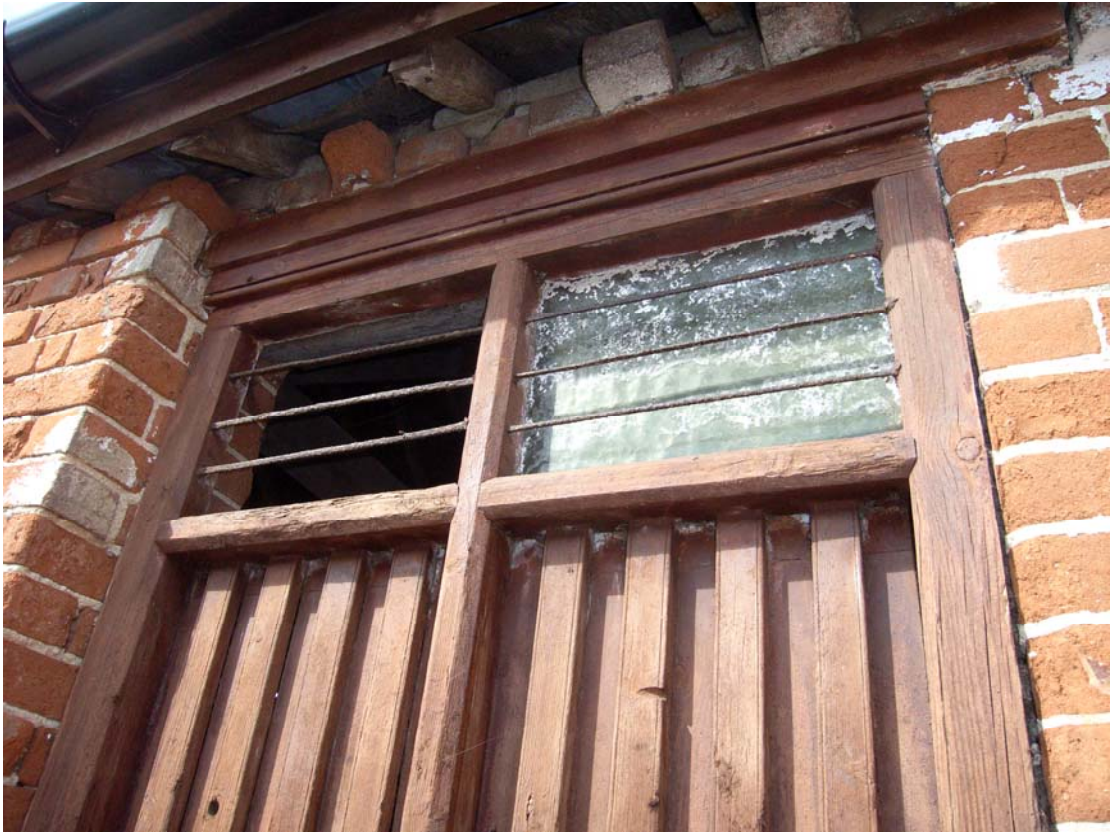
A2.7 External detail of original window to shed 3 from yard to east, showing glazed upper lights with vertical louver beneath
