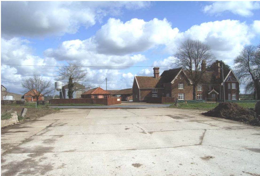
A2.1 General view from concrete hard-standing on site of demolished early-19 th century farm buildings to south-west, showing listed farmhouse to right with yard complex in rear and detached former cartlodge to left
