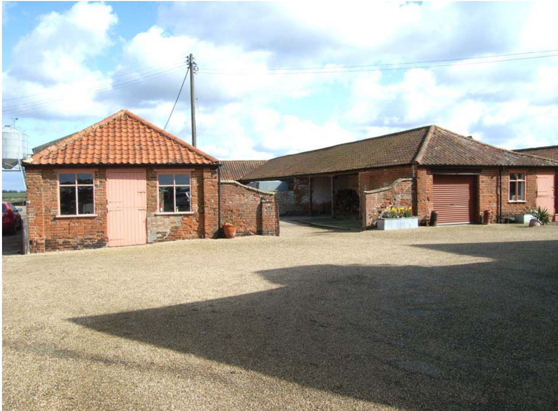
A2.5 Southern gables of yard ranges from south-east, with feed store (1) to left, central range to right and entrance to yard A in centre.
