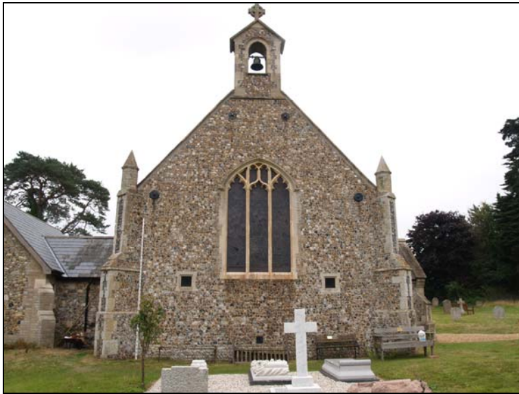
Plate 5 W. wall of nave
