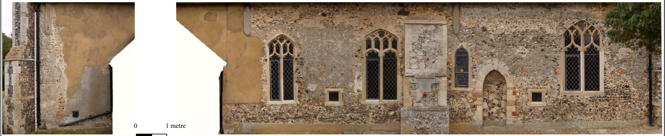
Plate 11 South nave & chancel wall, composite photograph
