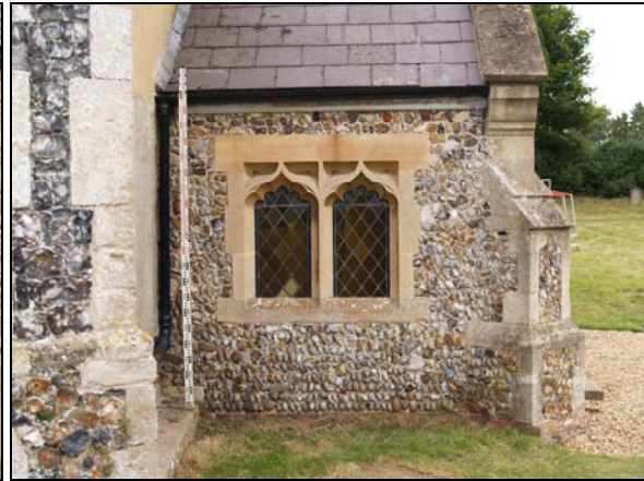
Plate 7 Porch W. wall
