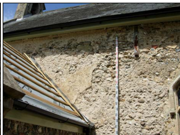
Plate 15 Detail of south wall east of porch
