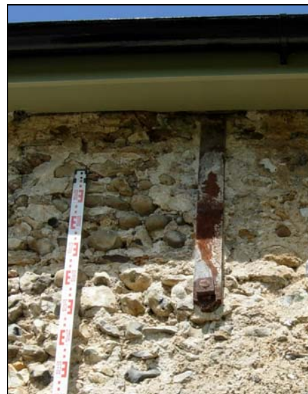
Plate 13 Detail of wall tie 0140
