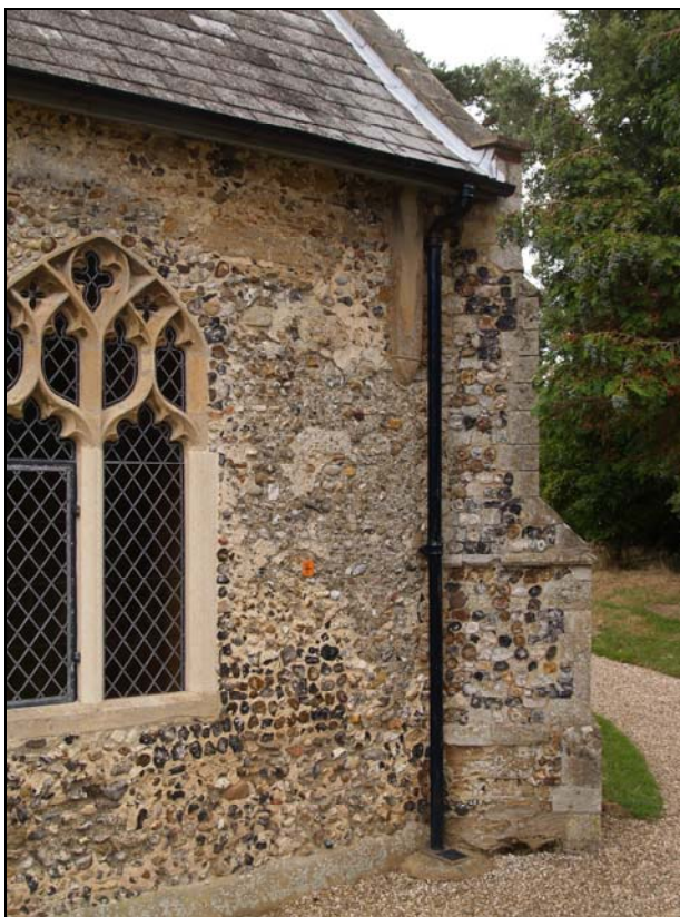
Plate 4 S. chancel wall, bracing element 0178
