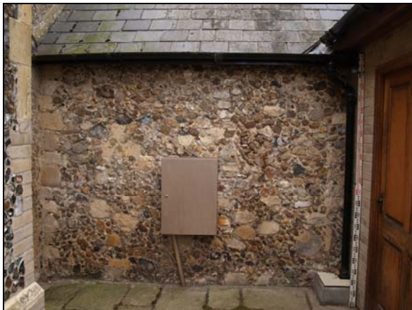
Plate 8 Victorian vestry, E. wall
