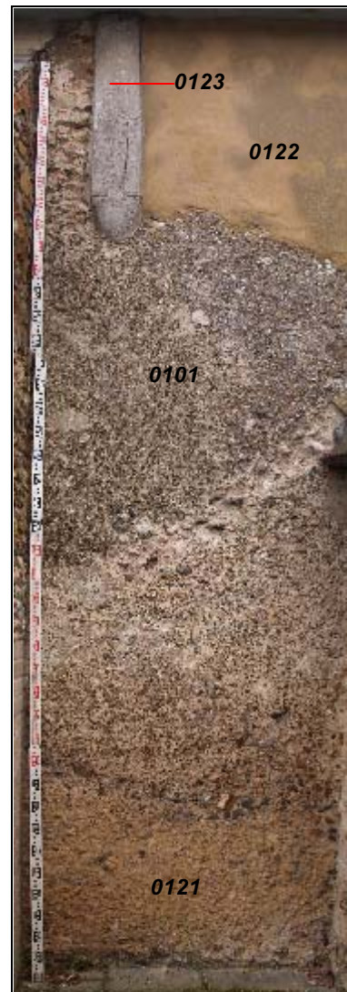
Plate 2 N. nave wall between buttress 0112 & vestry
