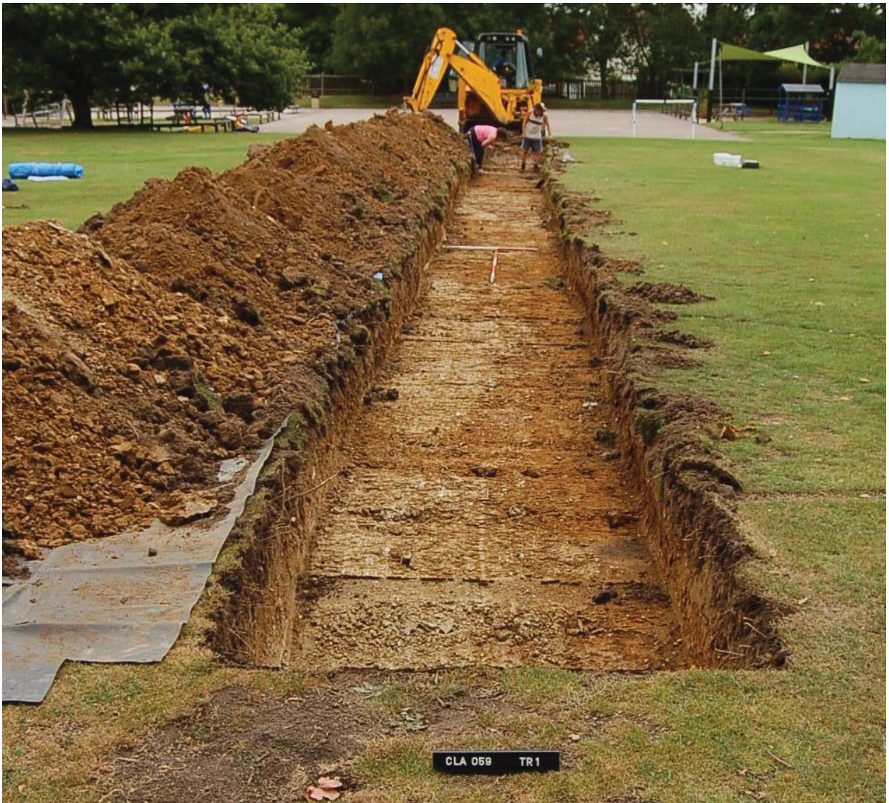
Plate 1. Trench 1, facing east (1m and 2m scales)
