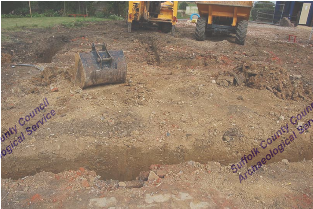
Plate 1. Site view across new footings, facing north
