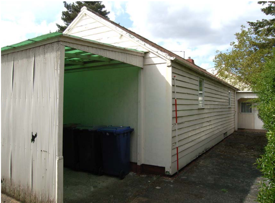
A2.2 External eastern elevation from south-east, showing lean-to shed (12) to left
