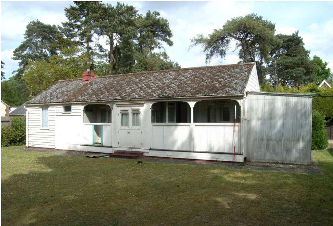
A2.1 External western elevation from garden to rear, showing verandas flanking 'French' double doors extruded from railway carriage and kitchen extension beyond chimney to left
