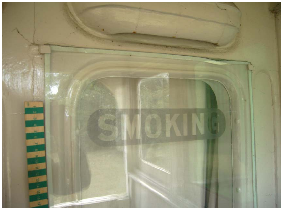
A2.6 Detail of etched SMOKING label to southern window of bedroom (1) seen from veranda (4)
