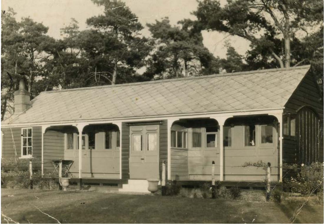
A2.13 Western external elevation in circa 1950, before the construction of the WC (7) and the containment of the verandas (6 & 4). Note the outline of the carriage in the southern gable to the right and the position of the original chimney. Photograph provided by current owners.
