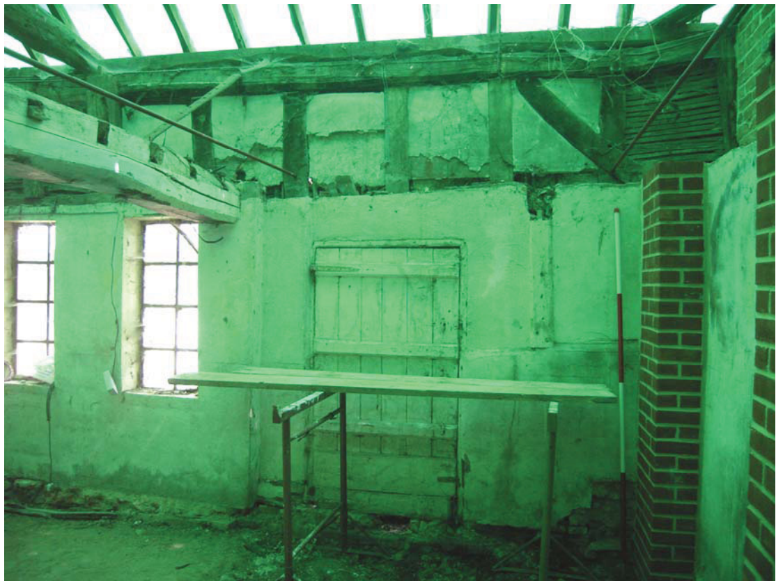
A2.6 Eastern end of northern internal elevation (bay A1) showing heavily sooted studs and internal corner brace – the lower part of the timber frame is hidden by 19 th century render.
