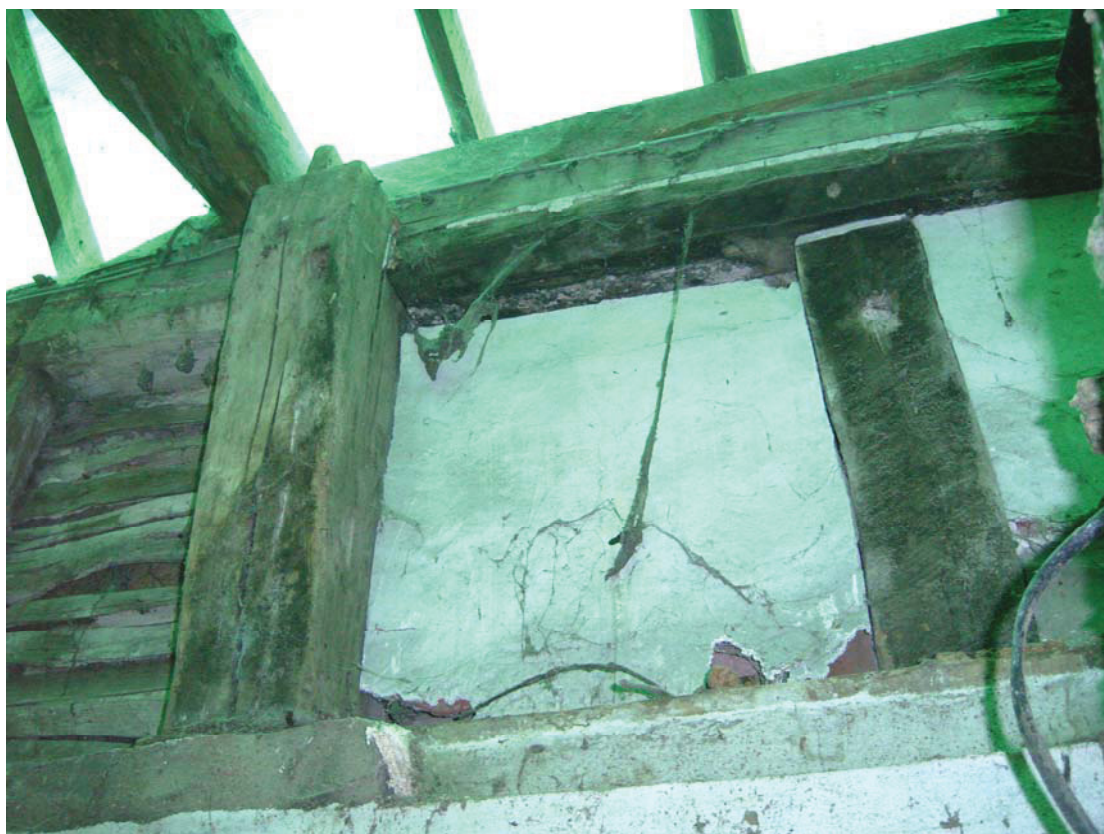
A2.7 Detail of jowled storey post dividing the sooted studs of bay A1 (right) from the unsooted studs of the central bay A2 (left). The storey post is sooted to its right-hand edge only, and contains notches for the wattle and daub of a missing lateral partition.
