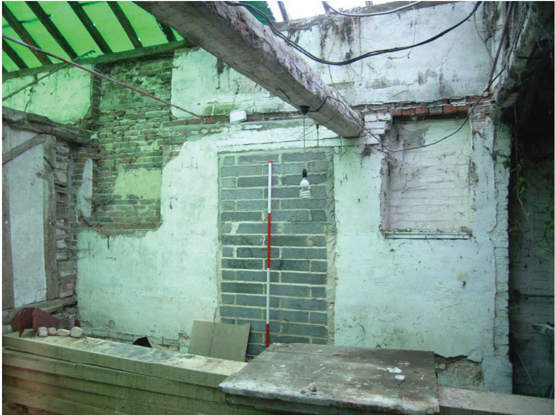
A2.11 Southern internal elevation of bays A3 (left) & B showing blocked 19th century door flanked by incised apotropaic circles and windows.
