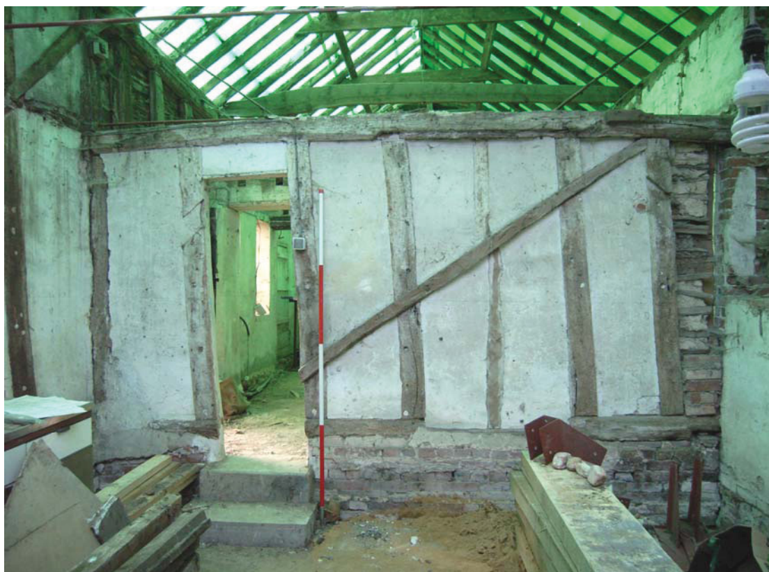
A2.9 Original 'service' partition seen from west (bay A3) showing existing door to left and blocked original door to right (the diagonal brace is secondary).
