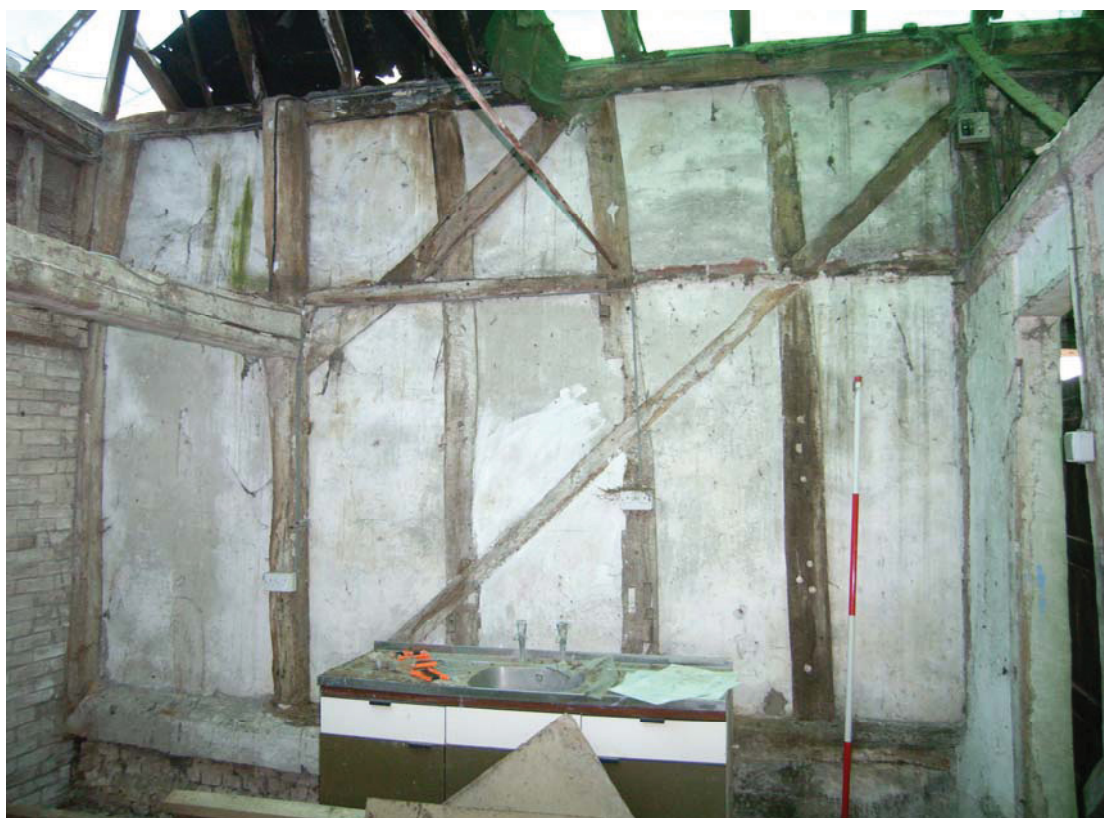
A2.10 Internal northern elevation of western bay (A3) showing original service partition to right and narrow 17 th century extension (B) to left.
