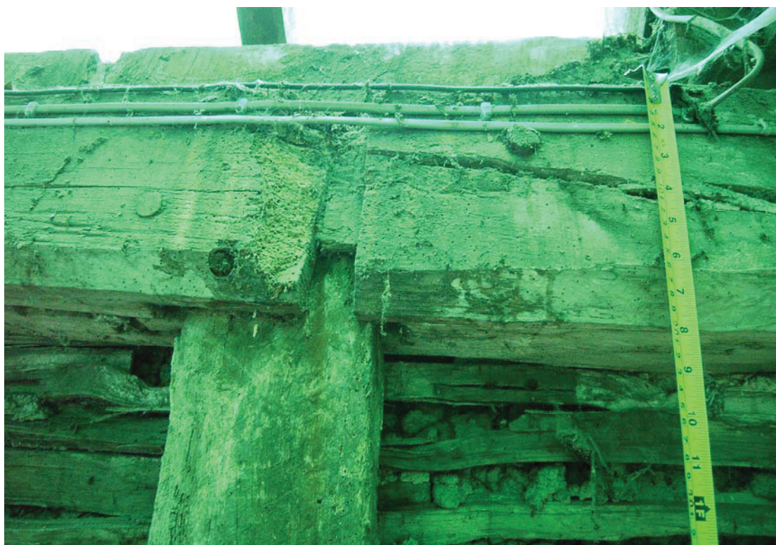
A2.8 Detail of unusual scarf joint in northern roof plate of central bay (A2). (Short face-halved joint with housed blade.)
