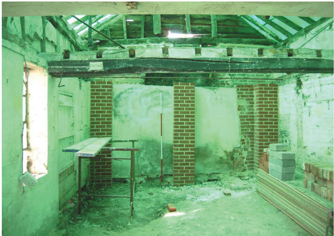
A2.4 General view of interior from west showing binding joists of 17 th century inserted ceiling and position of former fireplace against eastern gable (green tint caused by colour of tarpaulin covering stripped roof)
