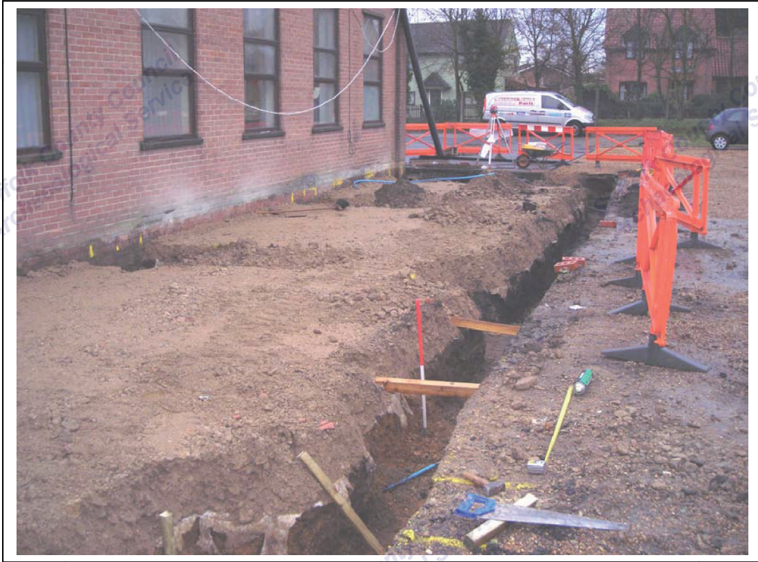
Plate 1. View of excavated extension footprint, looking SE
