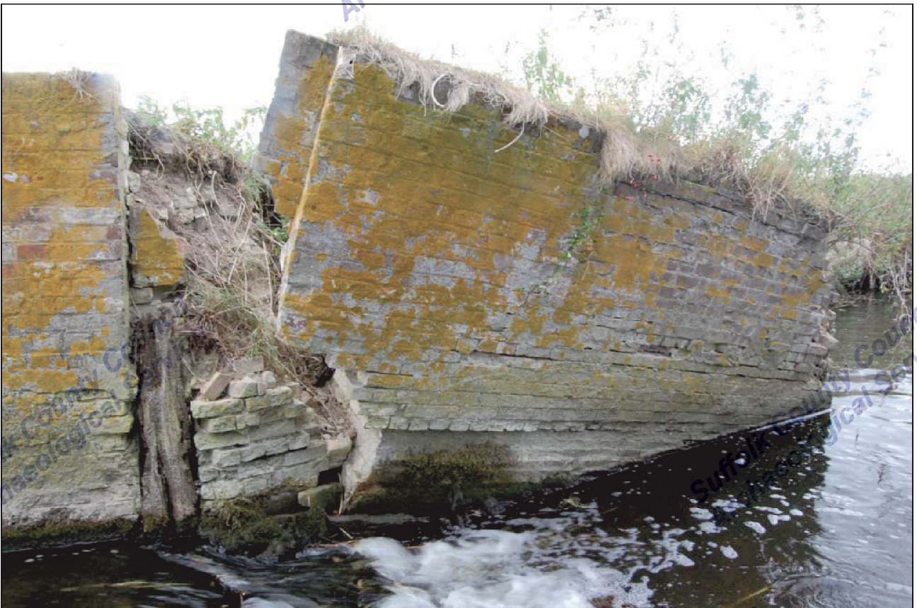
4. B-type walls, LKD 034, southern structure, western side
