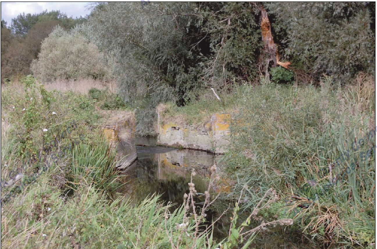
6. LKD 034, northern lock structure, looking NE
