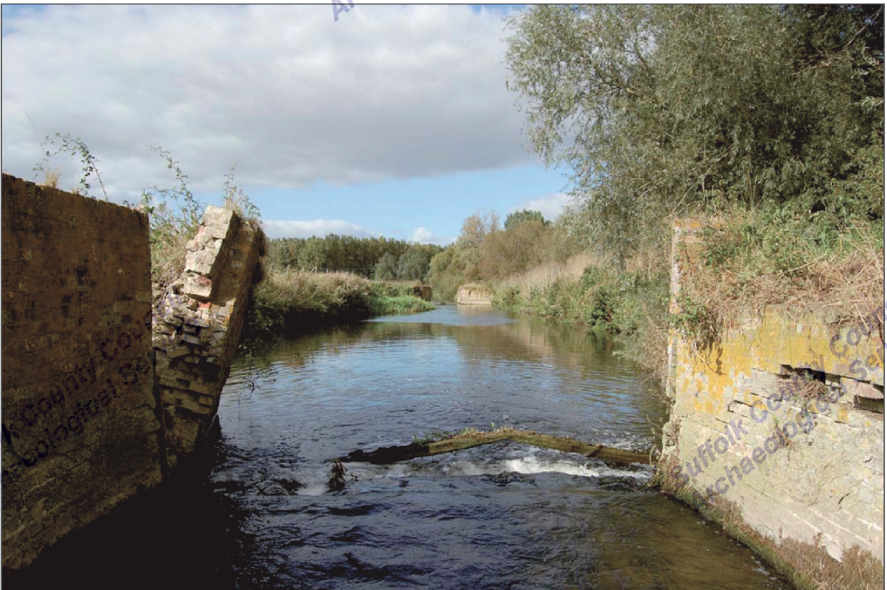
10. LKD 034, from southern lock structure, looking to northern structure
