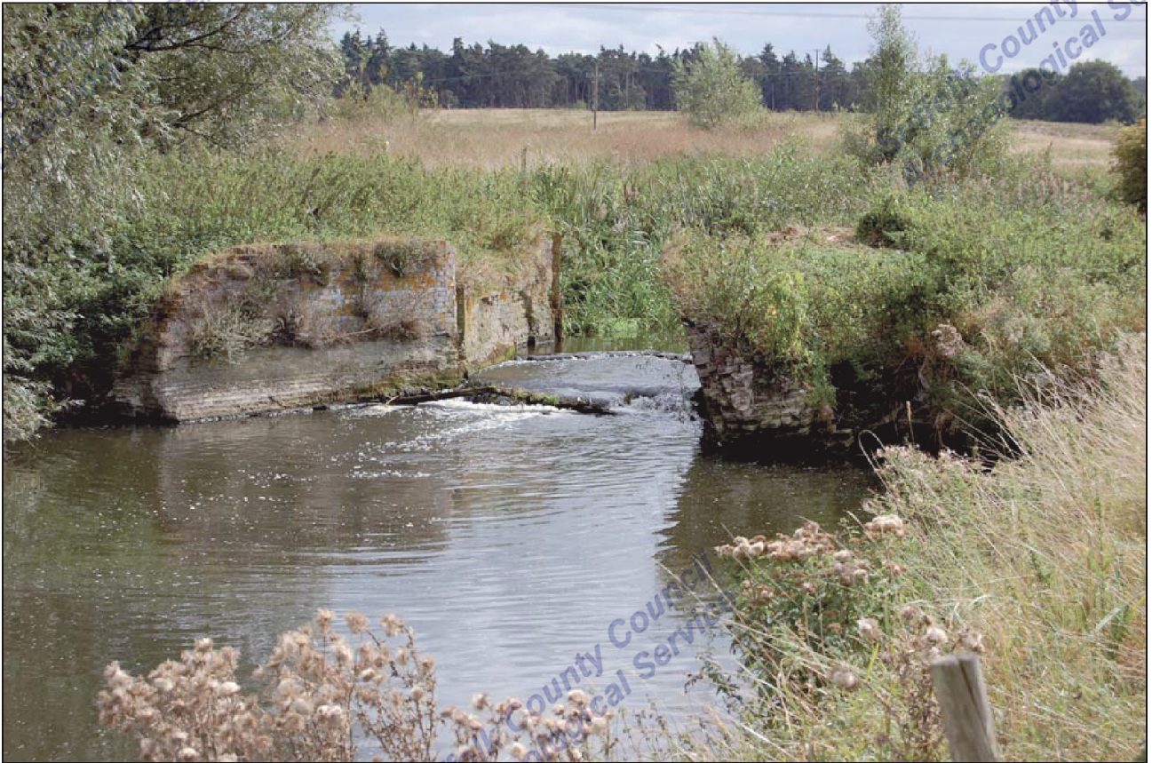
5. LKD 034, southern lock structure, looking SE
