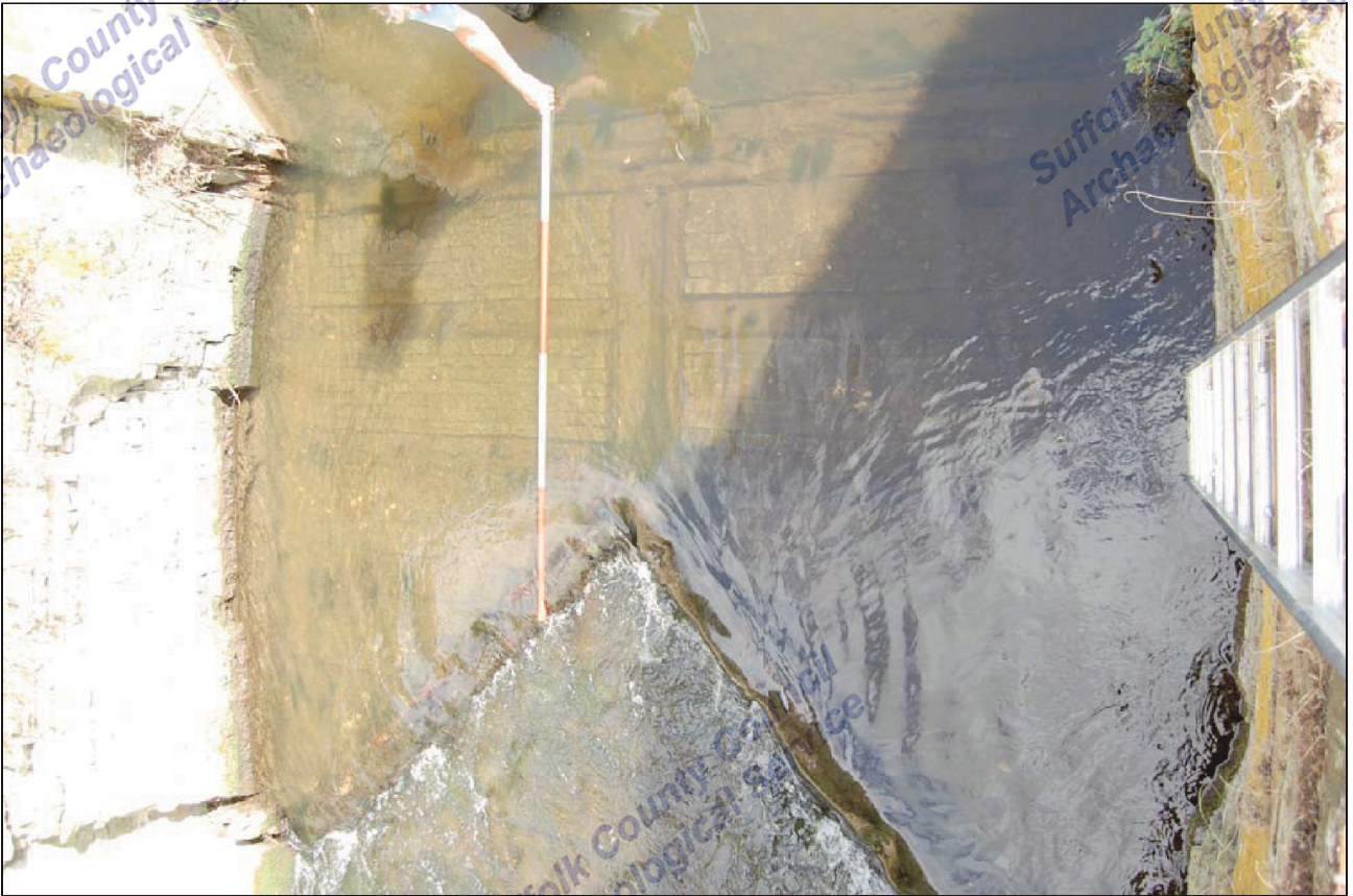
7. LKD 034, Base of lock structure
