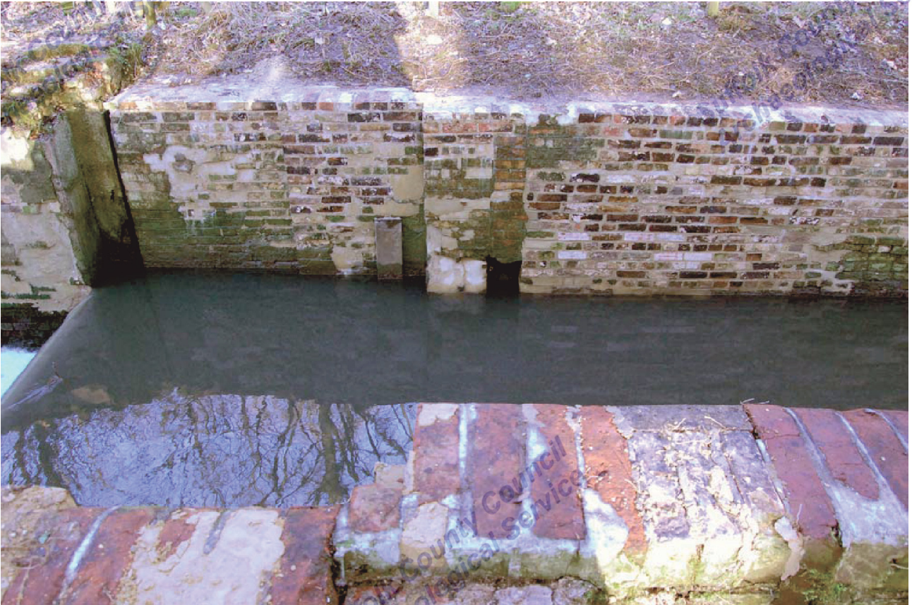
15. CUL 046, northern end, eastern wall timber recesses
