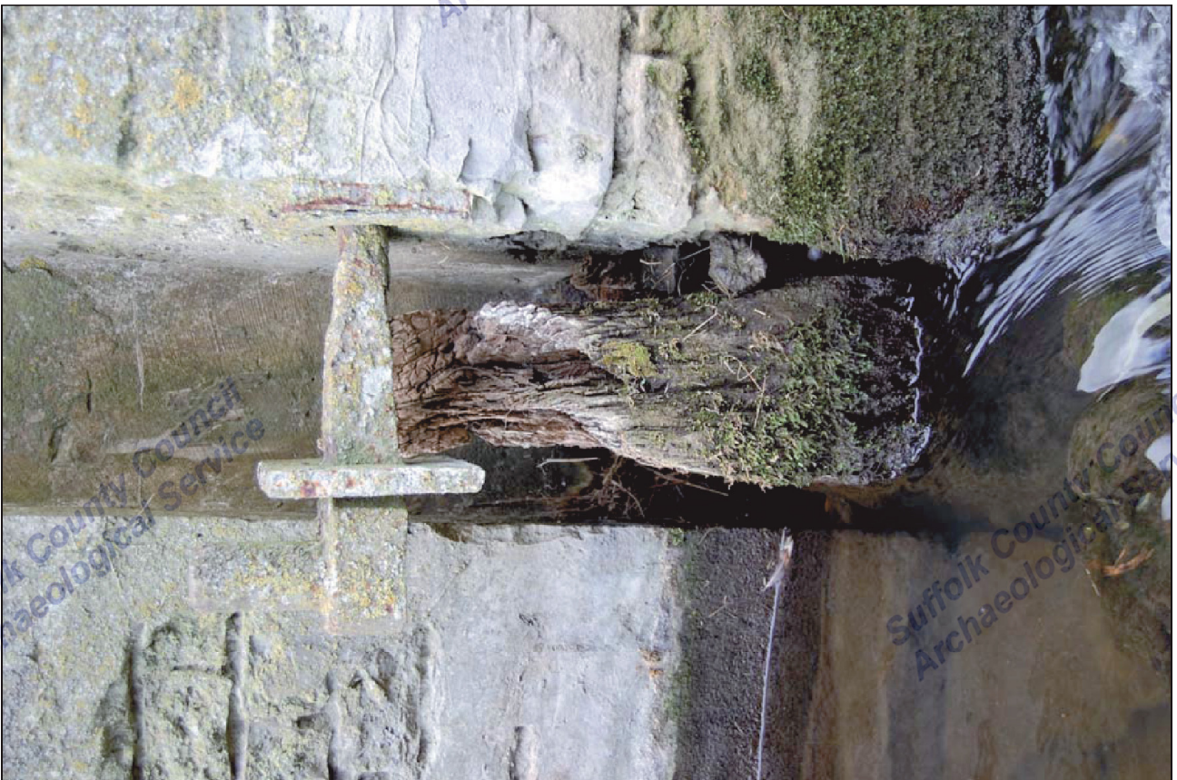
8. LKD 034, In-situ gate hinge, southern structure, western side
