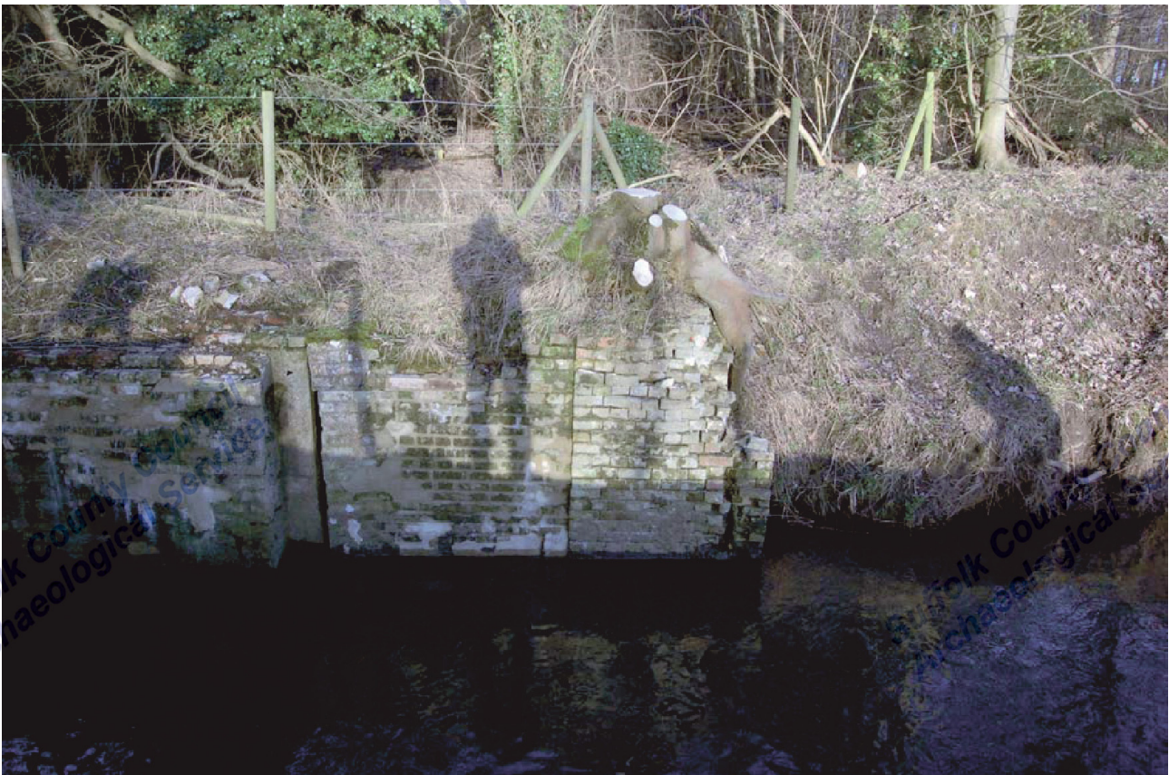
18. CUL 046, southern end, eastern side, timber recesses after cleaning
