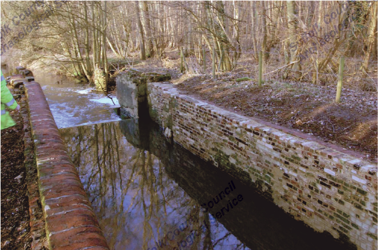
11. CUL 046, Lock structure, after cleaning, looking NE
