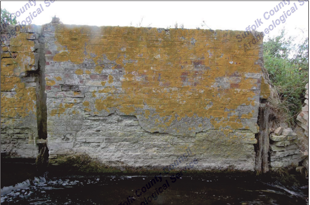
3. C2-type walls, LKD 034, southern structure, western side
