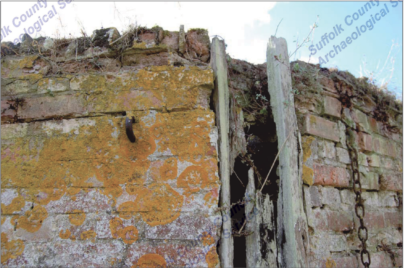
9. LKD 034, northern lock structure, western side, chain and hoop
