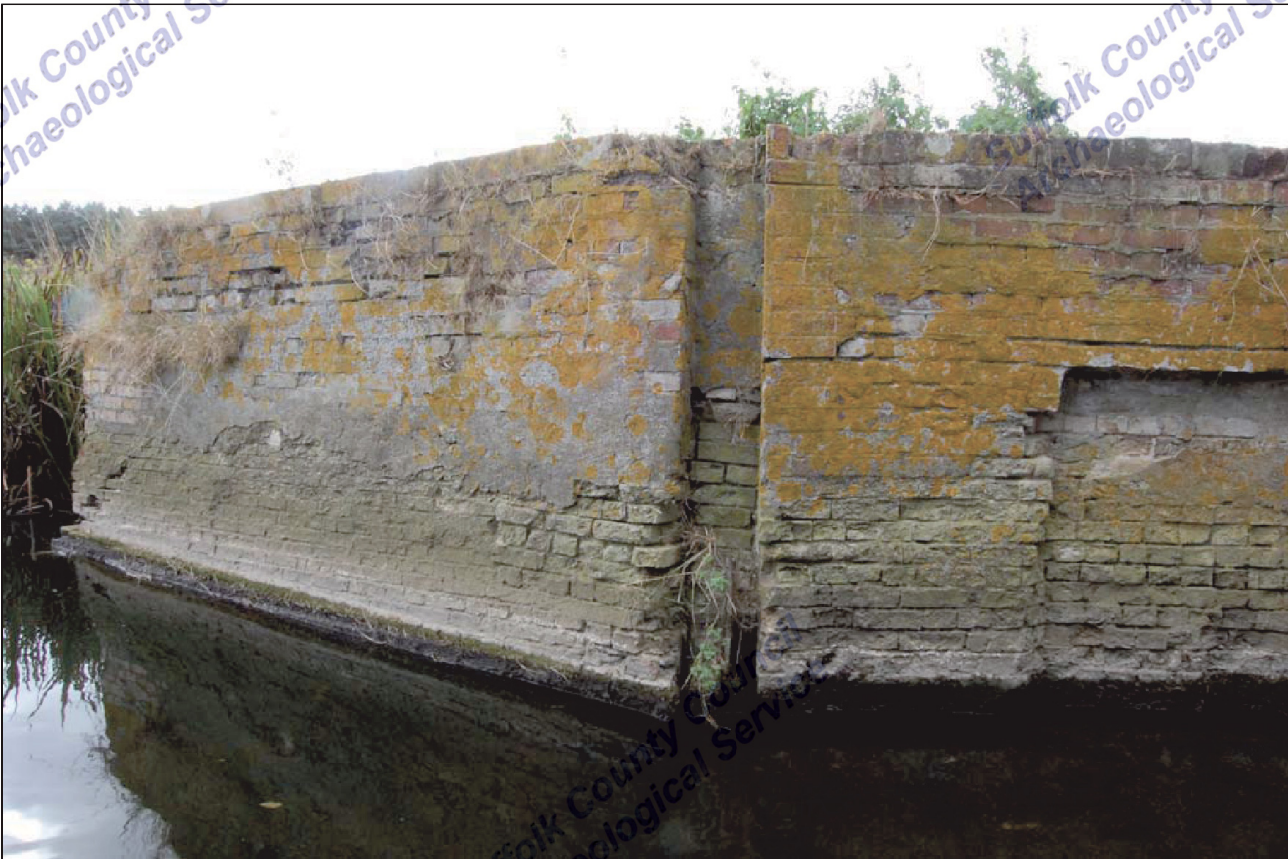
1. A-type wall, LKD 034, southern structure, western side
