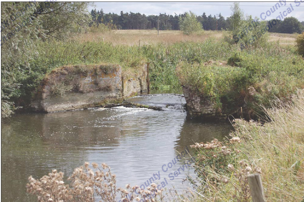
5. LKD 034, southern lock structure, looking SE
