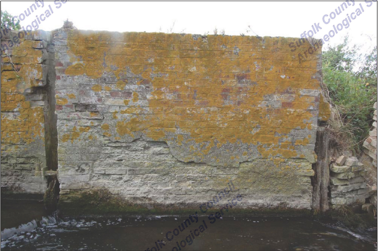
3. C2-type walls, LKD 034, southern structure, western side
