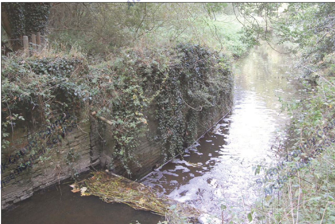
12. CUL 046, Lock structure, northern end, intact wall, looking NW
