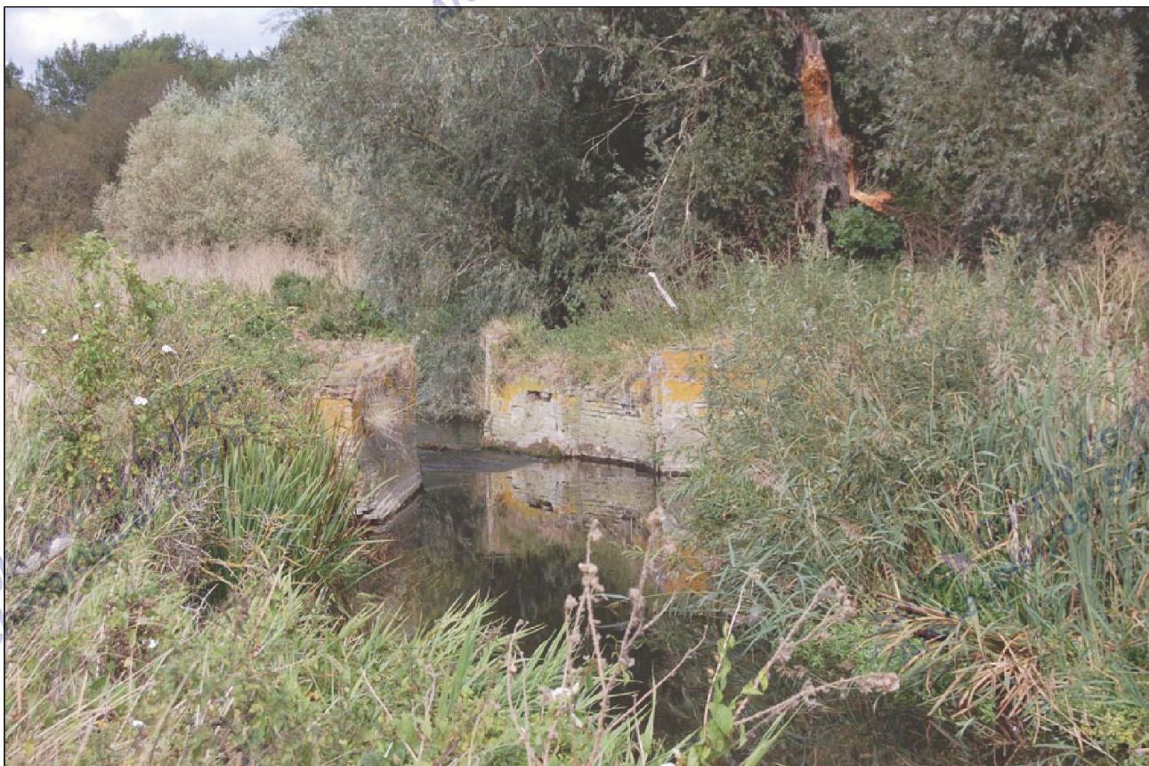
6. LKD 034, northern lock structure, looking NE
