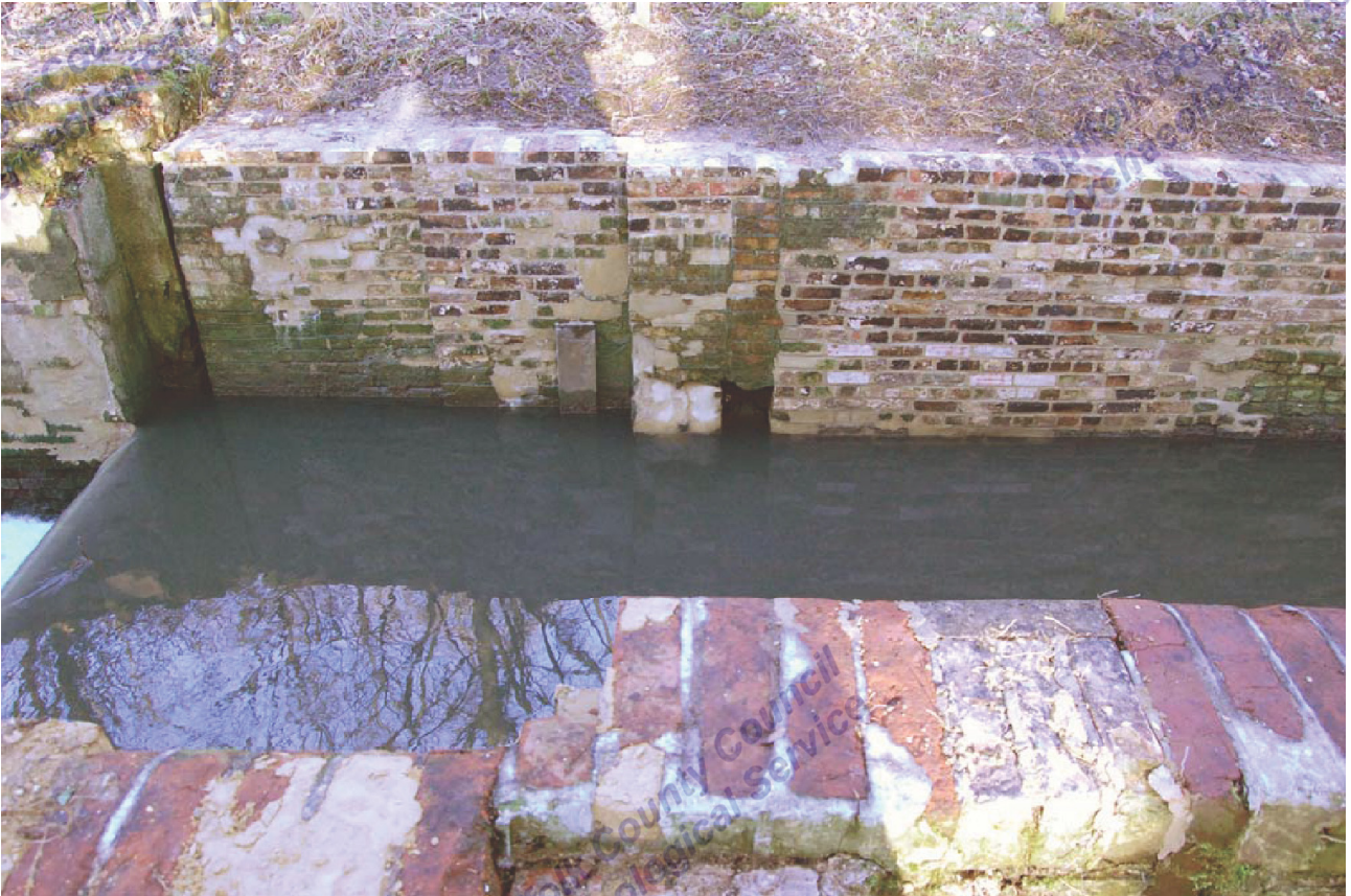
15. CUL 046, northern end, eastern wall timber recesses
