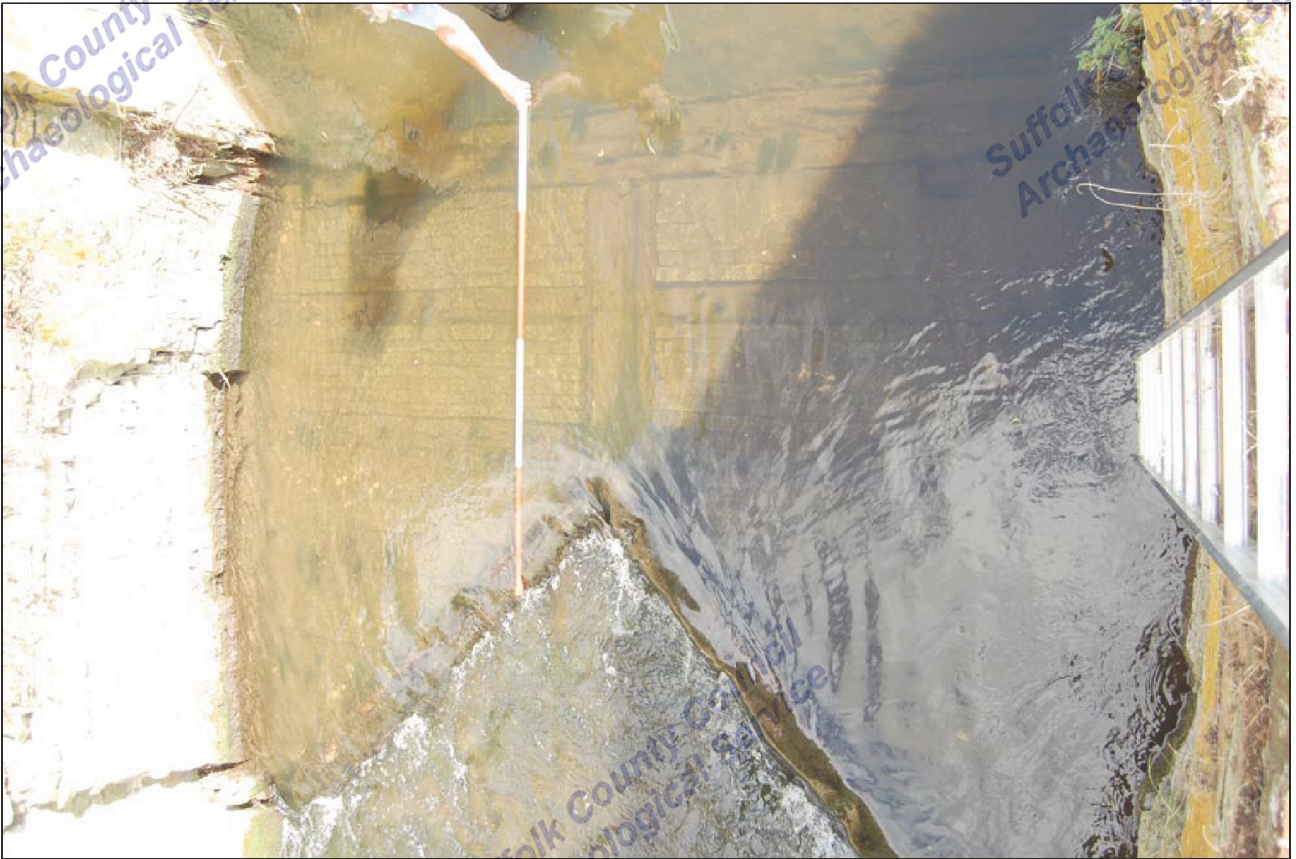
7. LKD 034, Base of lock structure
