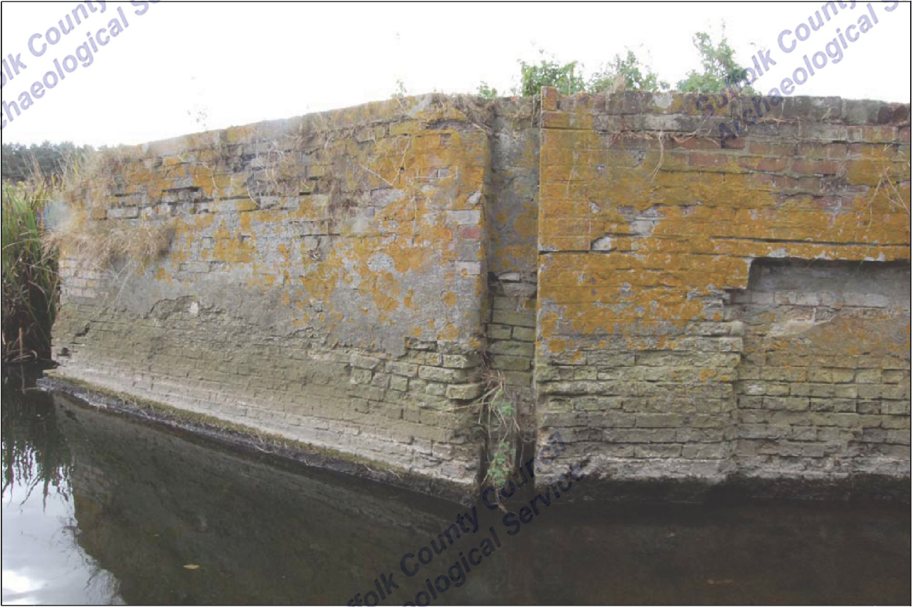
1. A-type wall, LKD 034, southern structure, western side
