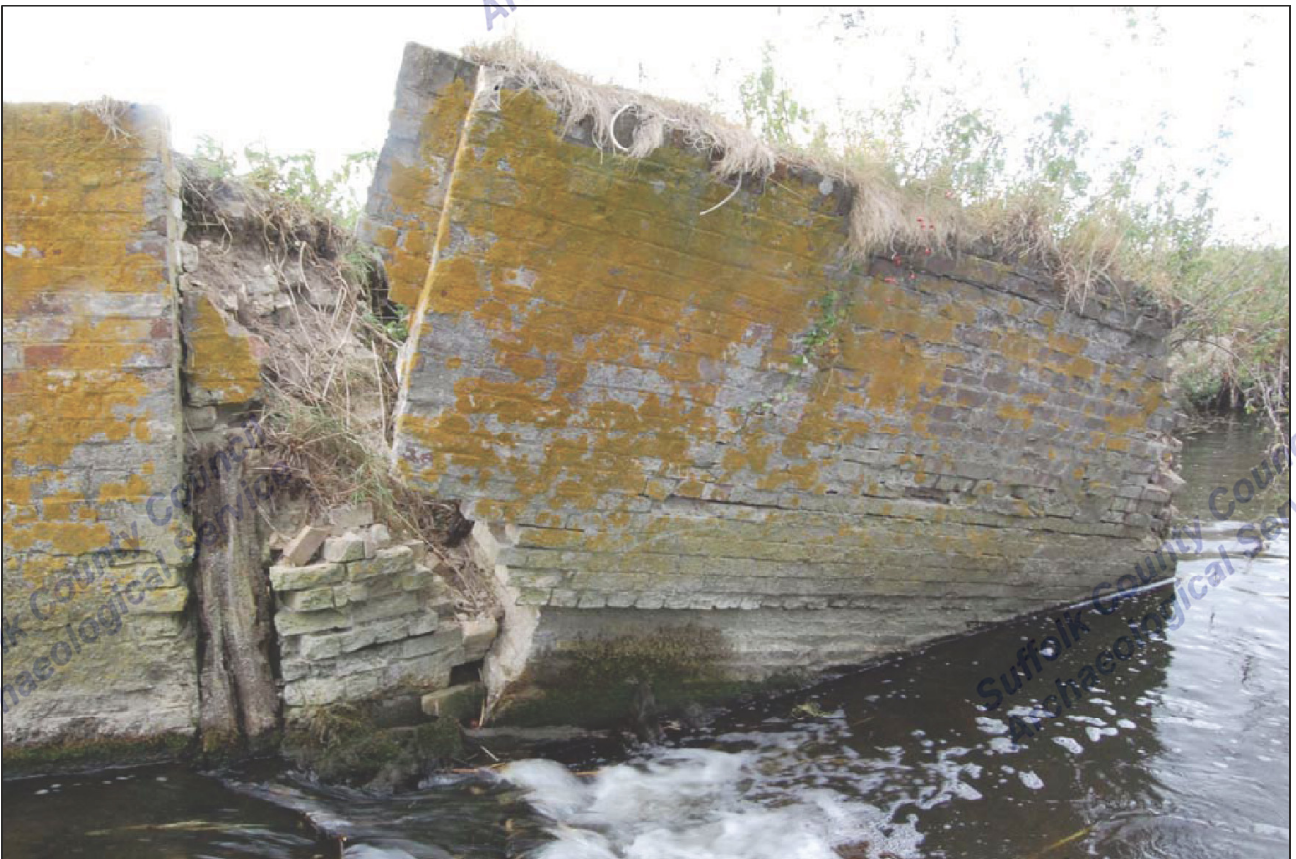
4. B-type walls, LKD 034, southern structure, western side
