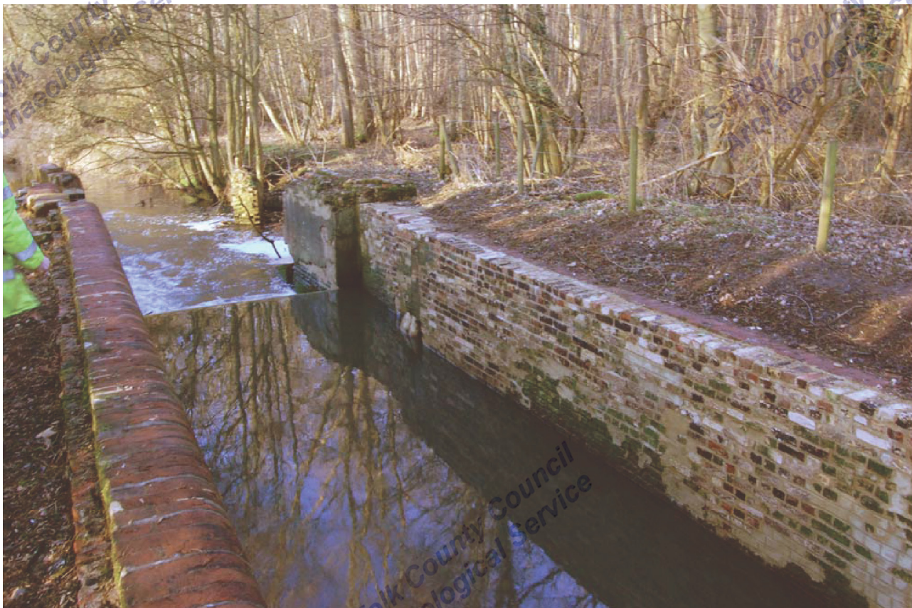
11. CUL 046, Lock structure, after cleaning, looking NE
