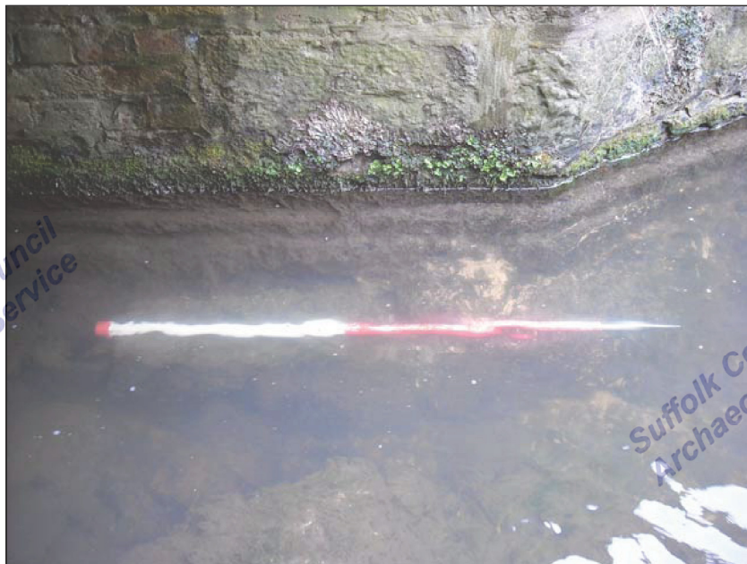
Plate 4. Stonework at the base of the bridge, facing south
