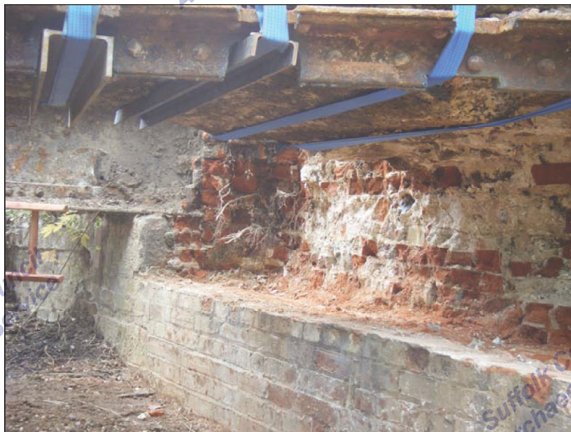
Plate 5. Exposed brick and flint construction piers, facing north-west
