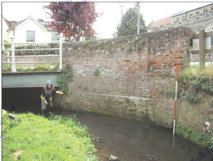
Plate 2. Brick revetment wall, facing south-east
