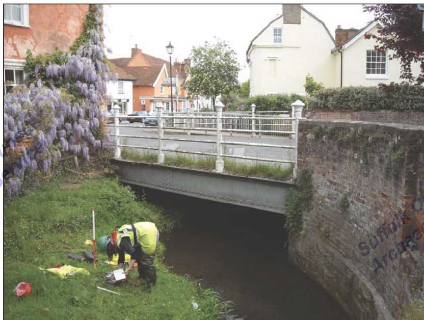
Plate 1. Boxford Bridge, facing north-east
