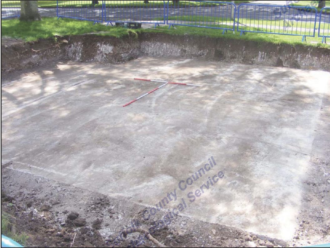
Plate 14. Water tank, looking south-east
