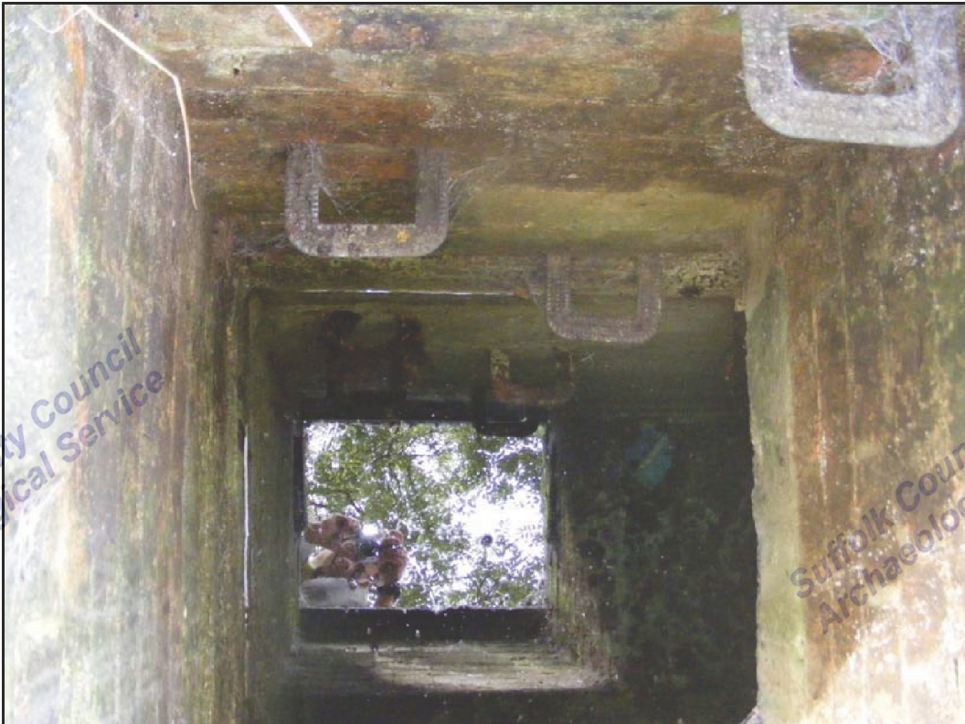
Plate 15. Manhole and rungs
