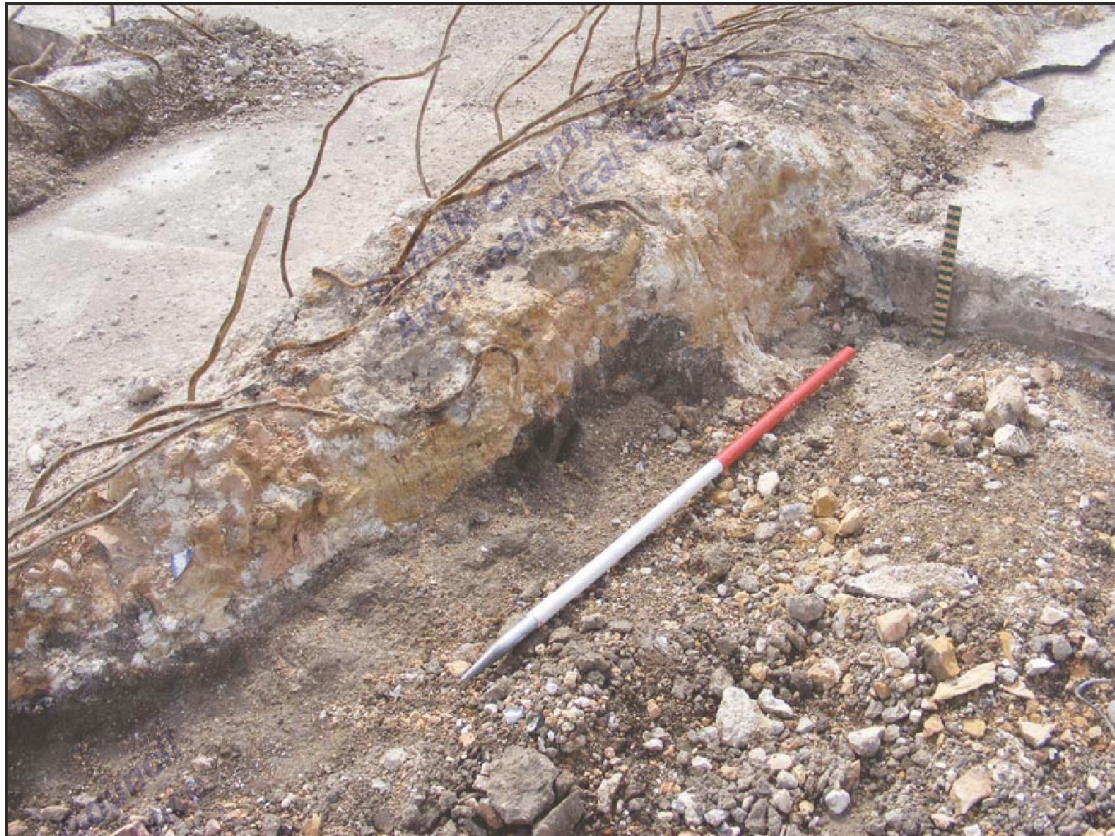
Plate 11. Reinforced and shored walls
