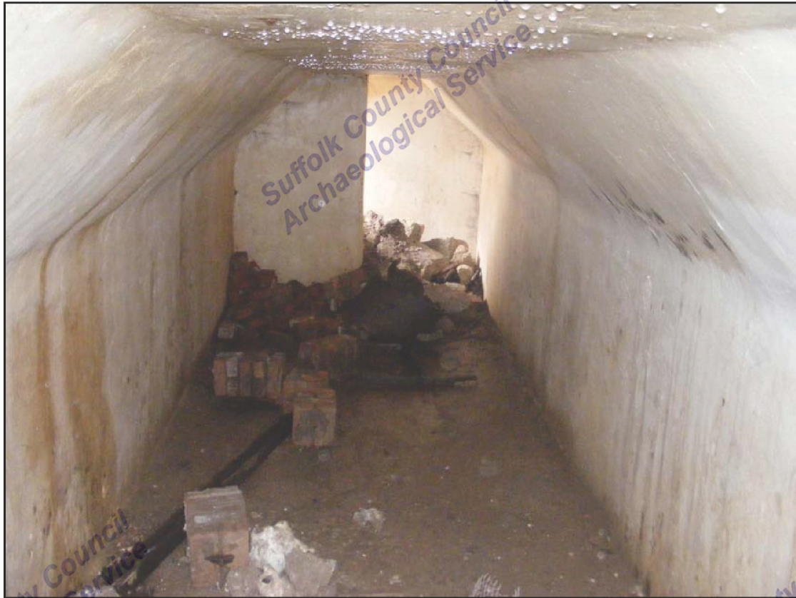
Plate 4. Internal view of structure from opening, looking north
