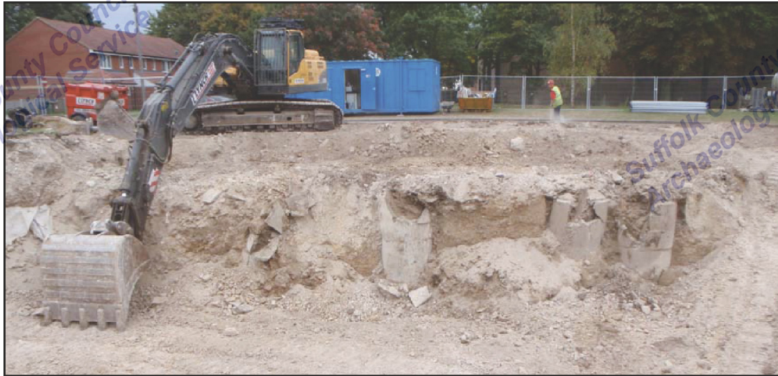
Plate 10. Concrete rings after main tank removal
