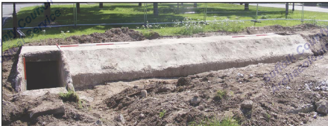
Plate 1. The air-raid shelter, looking east
