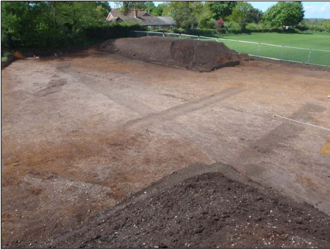
Plate 11. General shot looking NW showing ditch Group 1002 & evaluation trenches
