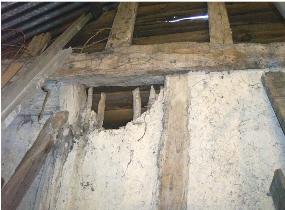
A2.12 Detail of original wattle-and-daub infill of western internal gable
