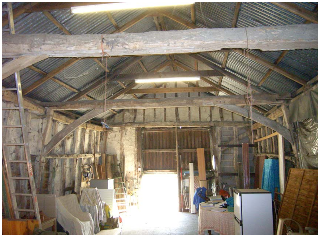
A2.6 General internal view of barn from west showing rails of former hay loft in eastern bay and 20 th century vehicle doors in eastern gable
