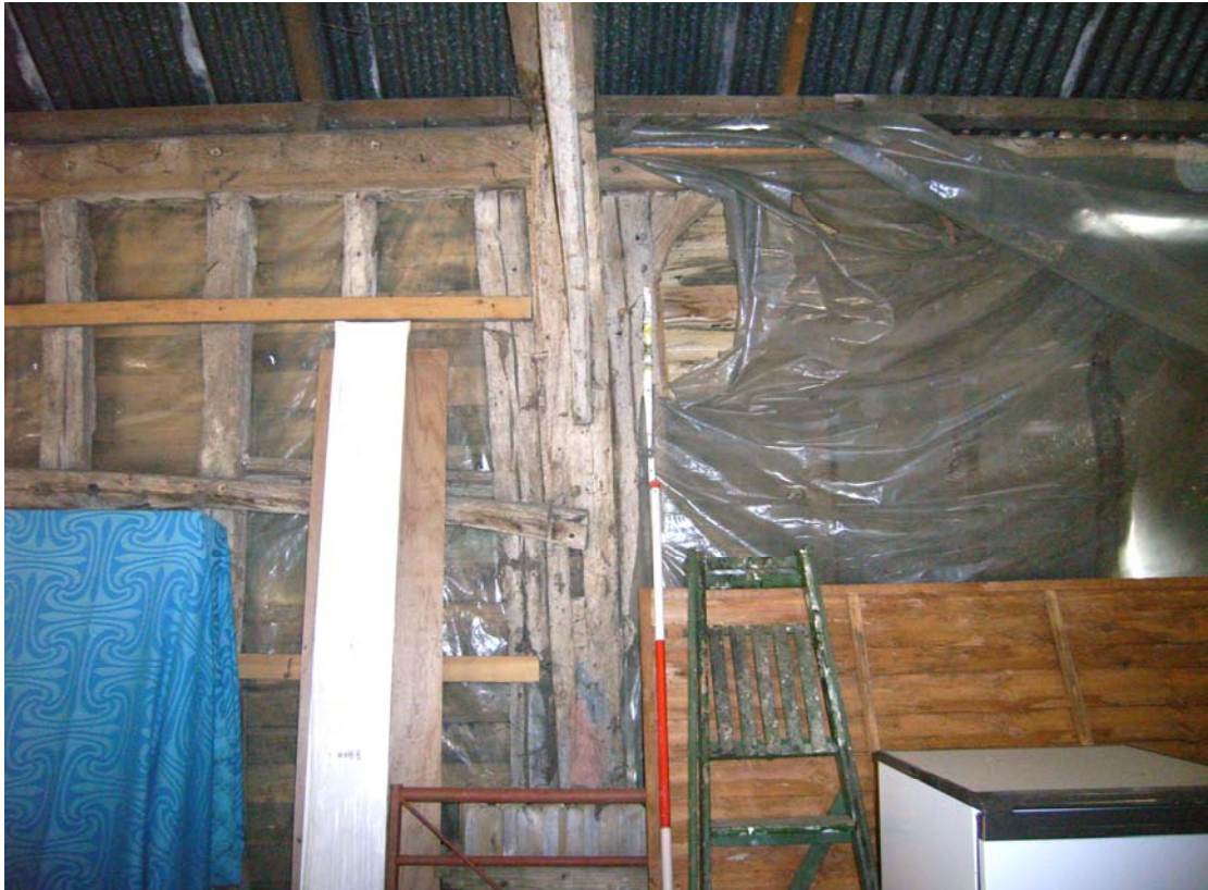
A2.9 Detail of internal southern elevation showing eastern storey post of central bay flanked by jambs of blocked stable door to left and main barn doors to right. The post contains the truncated rail of a removed lateral partition.
