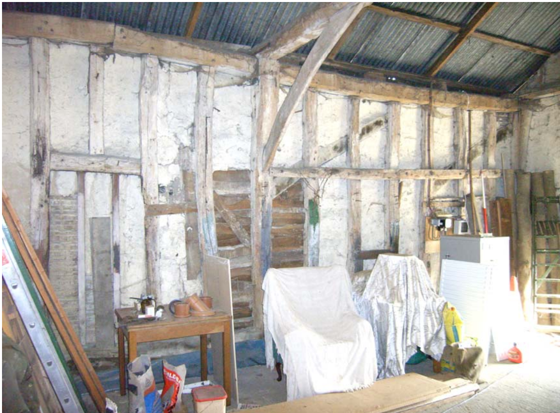
A2.8 Eastern half of northern internal elevation showing central door with raised lintel to left & clamp of removed stable ceiling to right
