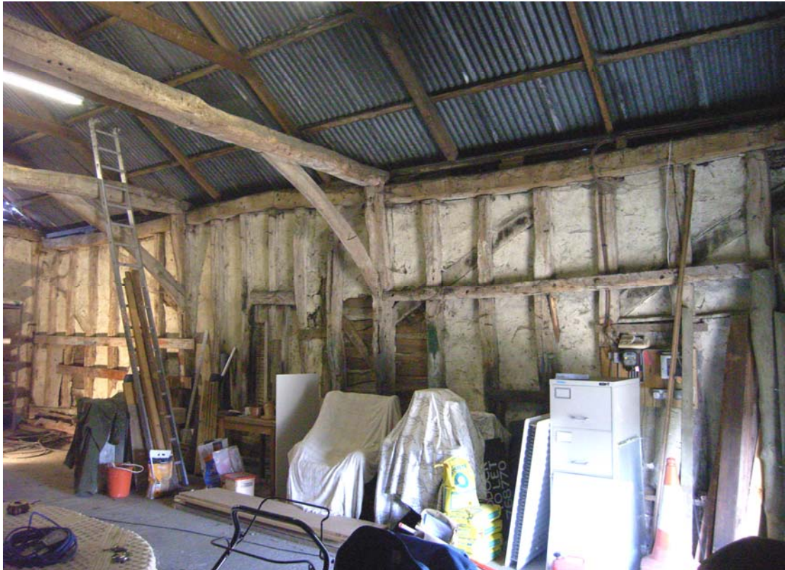
A2.7 Northern internal elevation showing unusual double wall braces in outer bays (externally trenched) and narrow door of central bay
