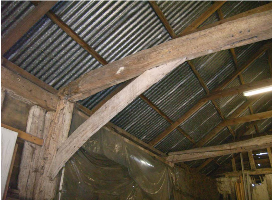
A2.11 Southern end of re-used eastern tie-beam showing empty arch-brace mortise to right of existing brace (seen from east)
