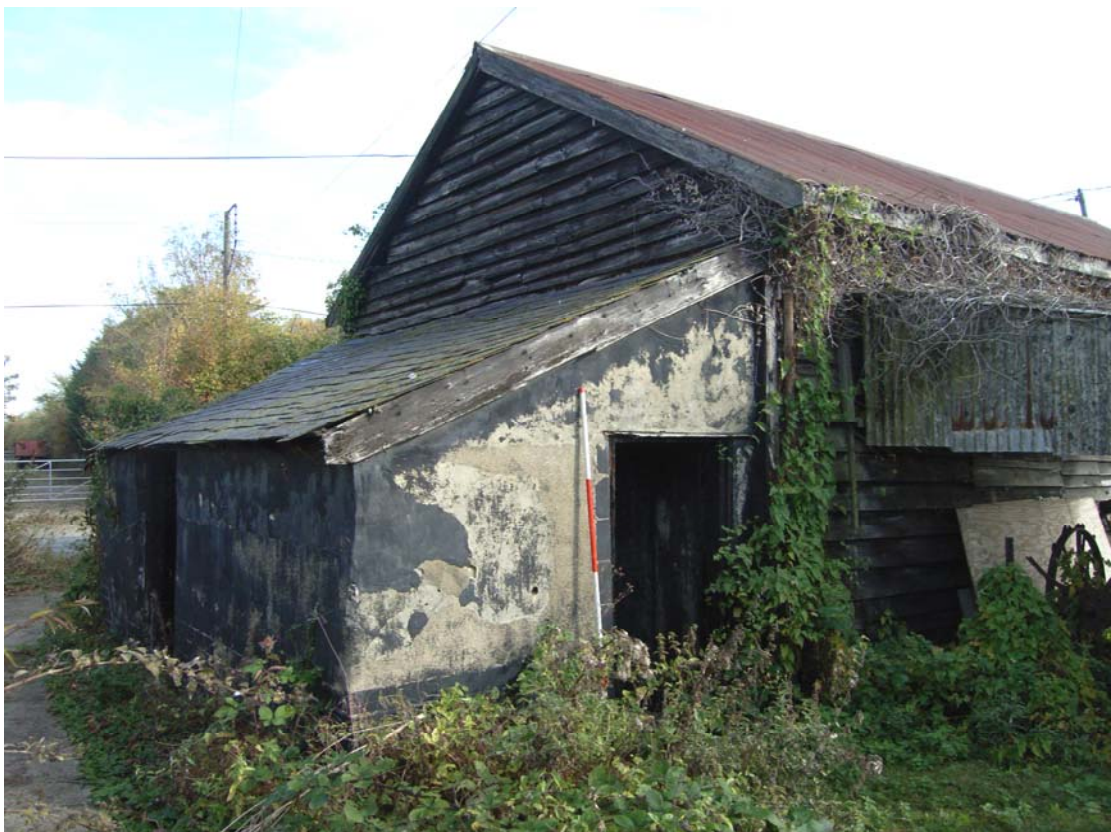
A2.4 Western external gable from south-west showing 19 th century clay-lump slated lean-to shed (B)
