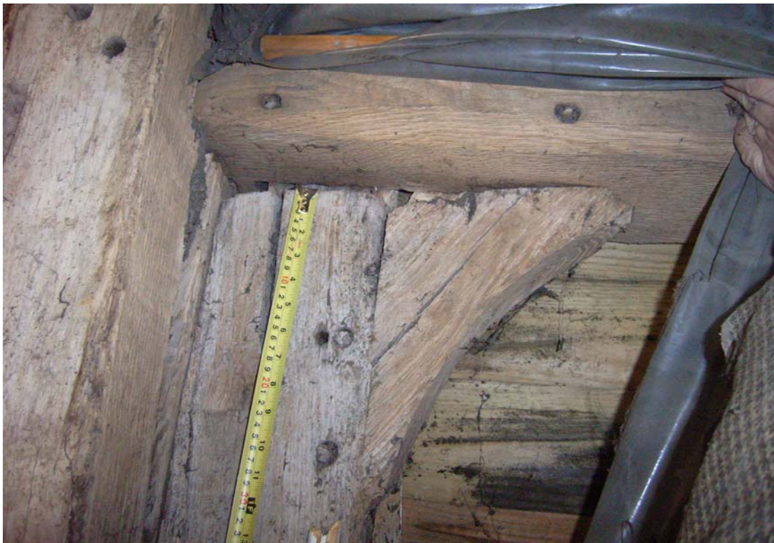
A2.10 Detail of tenoned corner bracket and jamb of main barn door to east of southern central bay
