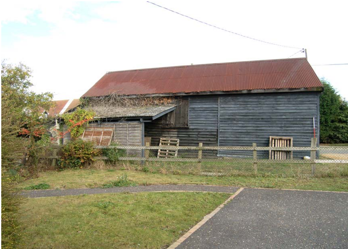
A2.3 Weatherboarded southern external elevation showing corrugated iron roof covering and remnant of central double-hung barn doors
