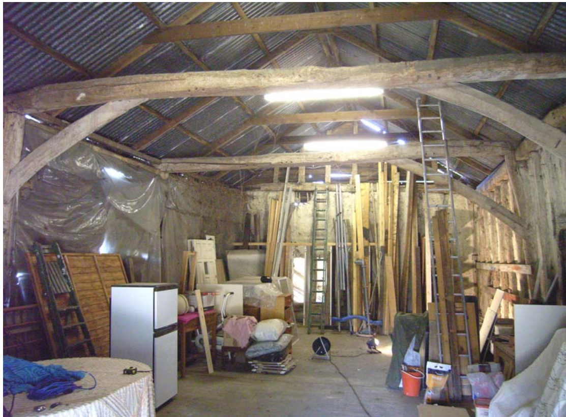
A2.5 General internal view of barn from eastern gable showing original arch-braces and tie-beams beneath rebuilt 20 th century roof structure.
