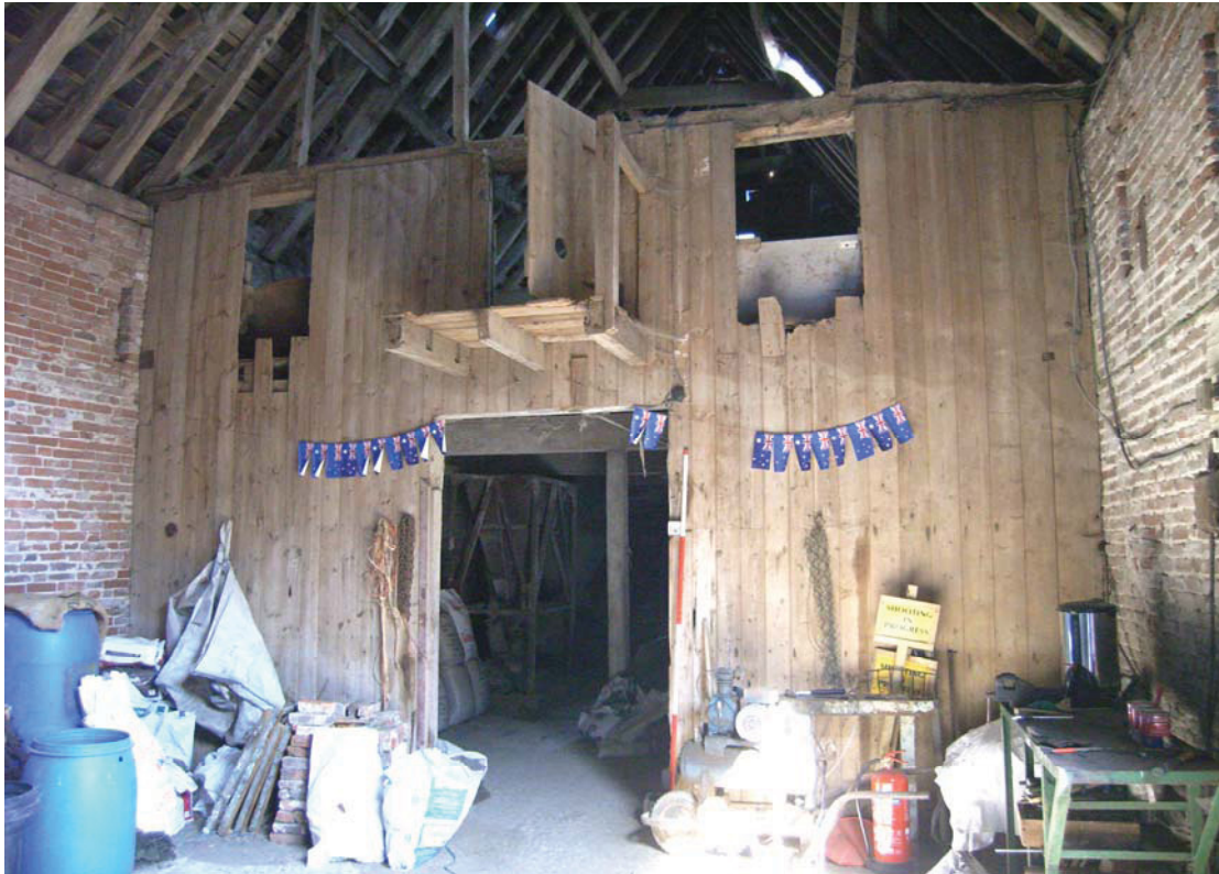
A2.9 The boarded partition of the 20 th century grain and milling floor at the eastern end of the barn. Note the original ventilation slits to left and right.
