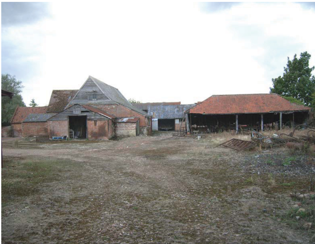
A2.2 General view of site from east showing the barn and attached sheds to left, the entrance to the northern yard in centre and the shelter shed of the eastern yard (N) to right
