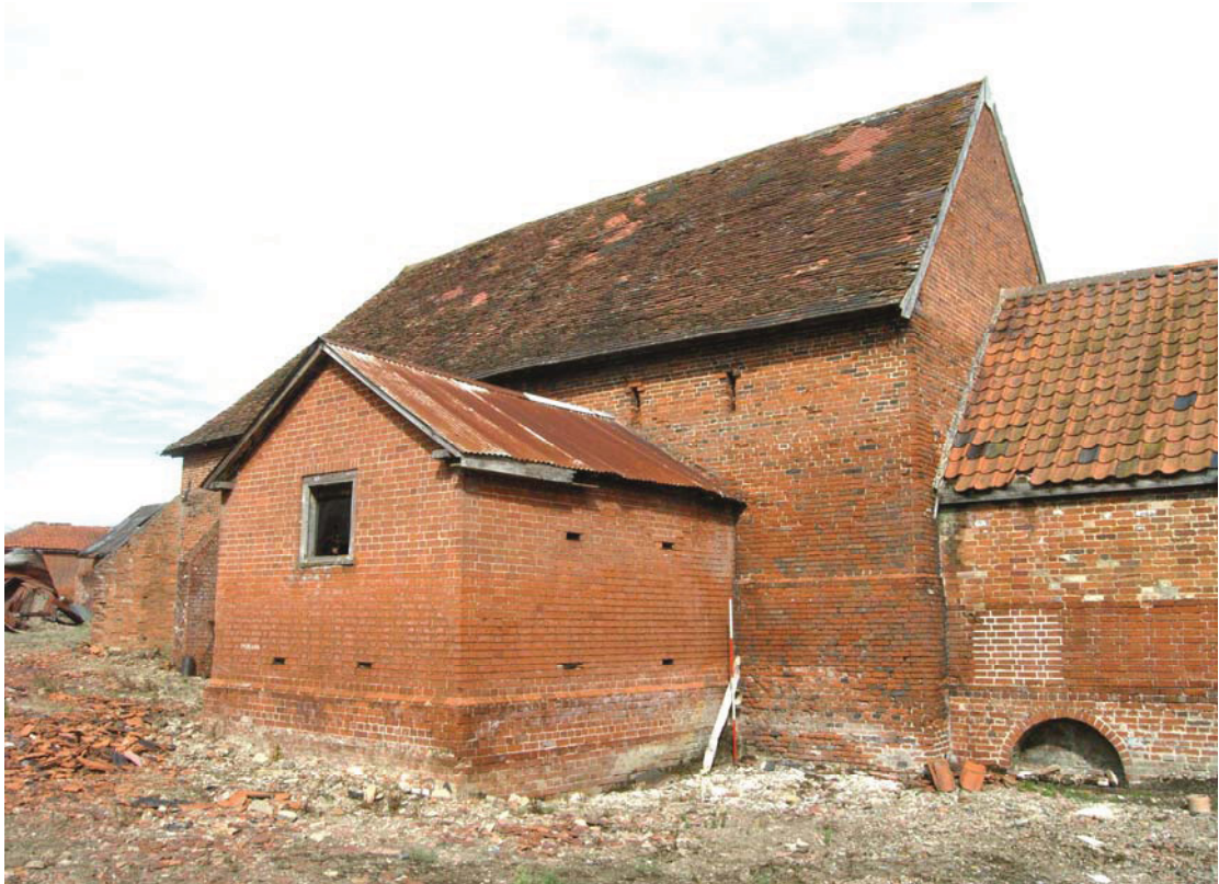
A2.5 Western external elevation of the stable (B) showing its original ventilation slits and the secondary tack room (C) in the foreground. The vehicle shed (D) is shown to the right with an arched plinth that may relate to a yard drain.
