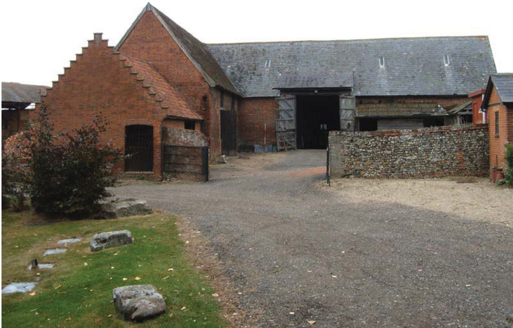
A2.1 General view of yard entrance from south showing the brick barn and contemporary stable wing with later crow-stepped shed to left. A similar wing originally projected from the right-hand side of the barn but has been demolished
